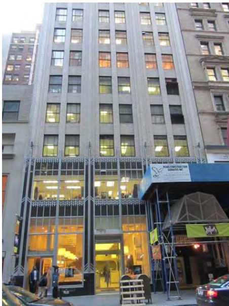
Photo 99: 6 East 45th Street, Title Guarantee and Trust Company (NYCL-Eligible: PROJECT AREA), Projected Development Site 4
