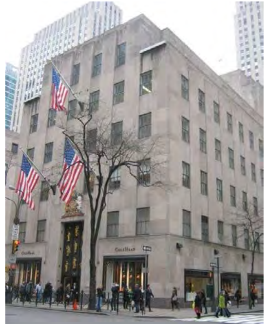
Photo 38(4): 620 Fifth Avenue, Rockefeller Center (British Empire Building) (NYCL, S/NR, NHL)
