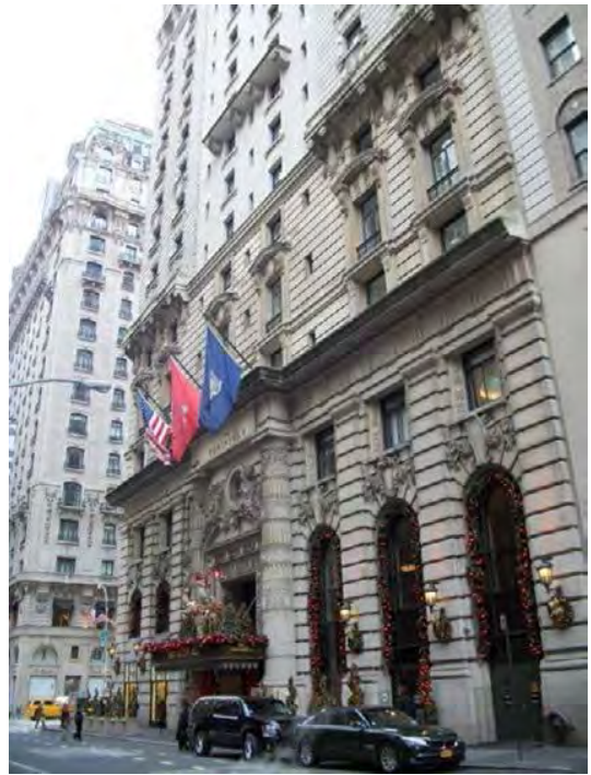
Photo 14: 696 Fifth Avenue, Gotham Hotel (NYCL)
