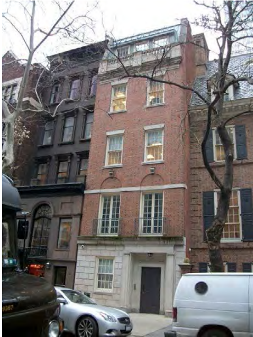
Photo 117: 120 East 55th Street (S/NR-Eligible district: STUDY AREA)
