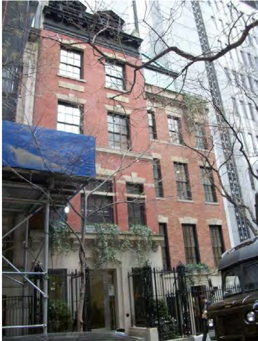
Photo 115: 117 East 55th Street (S/NR-Eligible district: STUDY AREA)
