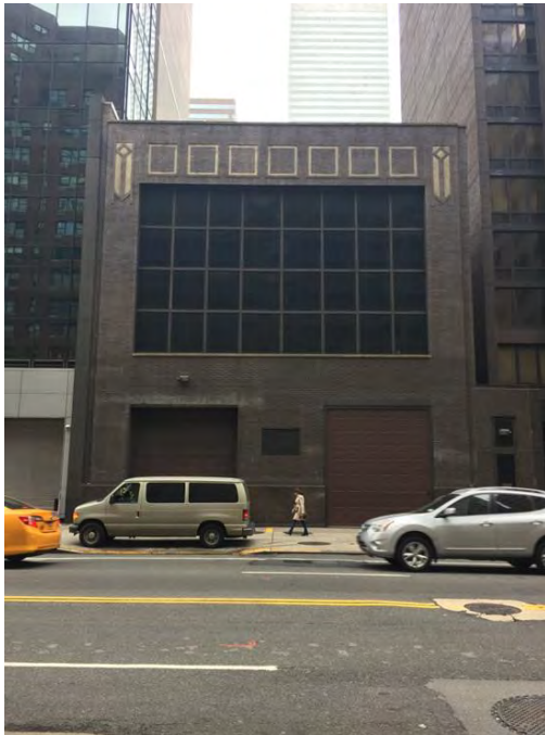
Photo 7: Subway Substation Station 42, South side of East 57 th Street between Lexington and Third Avenue, 154 East 57 th Street (S/NR)
