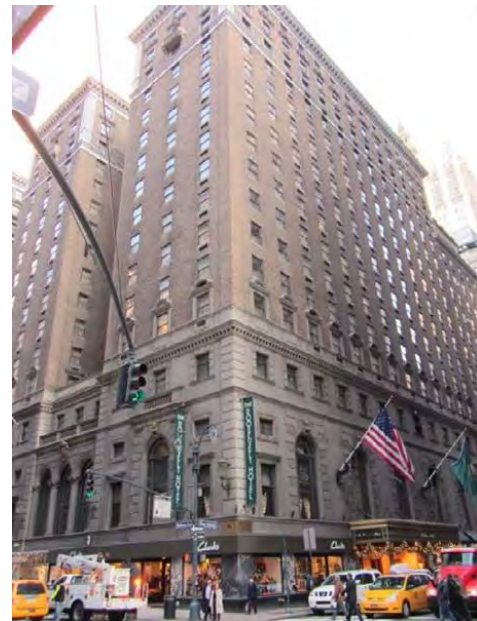
Photo 100: 45 East 45th Street, Roosevelt Hotel (NYCL and S/NR-Eligible: STUDY AREA)
