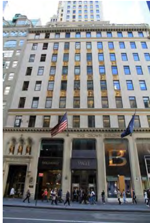
Photo 146: 730 Fifth Avenue, Hecksher Building (S/NR-Eligible: STUDY AREA)
