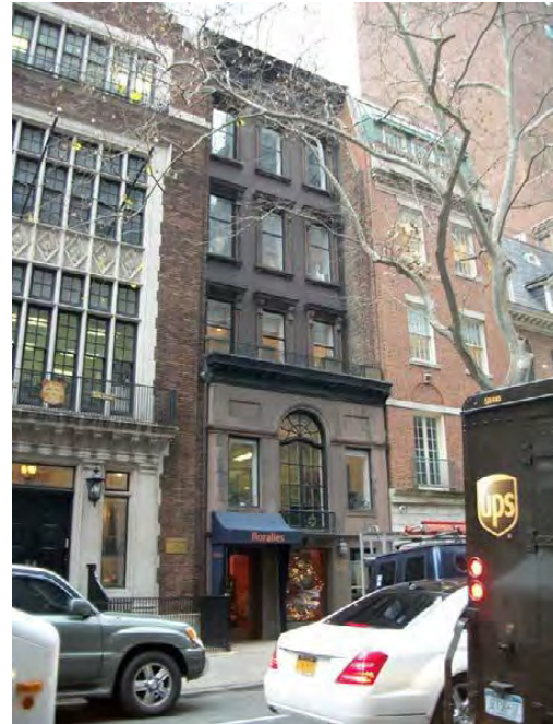
Photo 118: 122 East 55th Street (S/NR-Eligible district: STUDY AREA)
