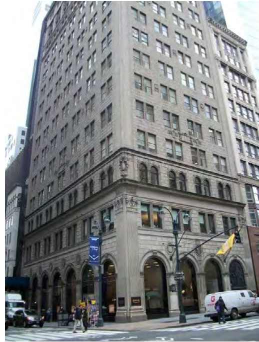
Photo 138: 511 Fifth Avenue Building, Postal Life Building (NYCL-Eligible: STUDY AREA)
