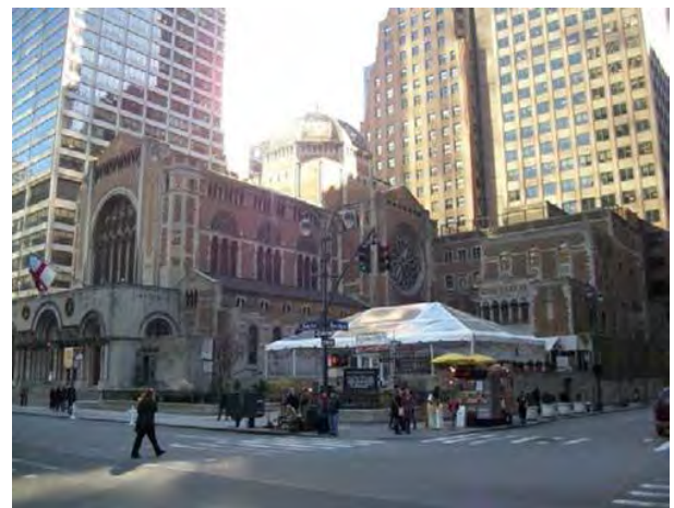
Photo 32: 321 Park Avenue, 109 East 50 th Street, St. Bartholomew's Church & Community House (NYCL, S/NR)
