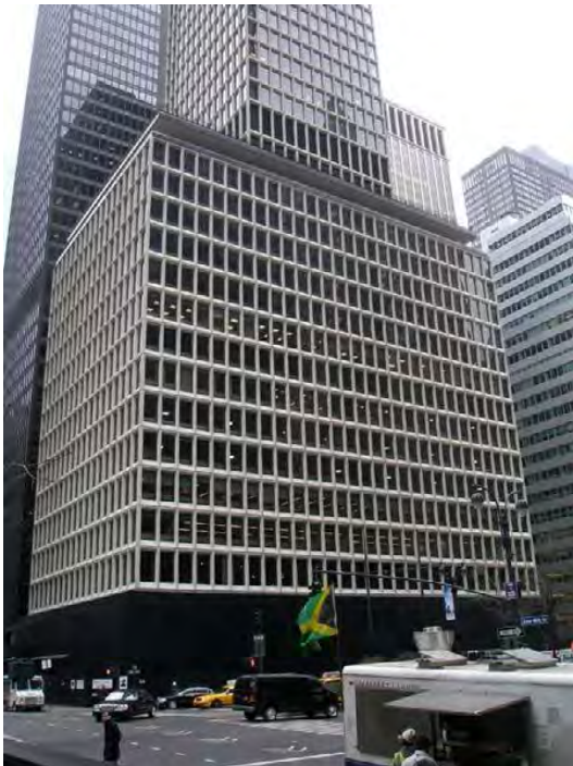
Photo 143: 280 Park Avenue, Bankers Trust Building (S/NR-Eligible: PROJECT AREA)
