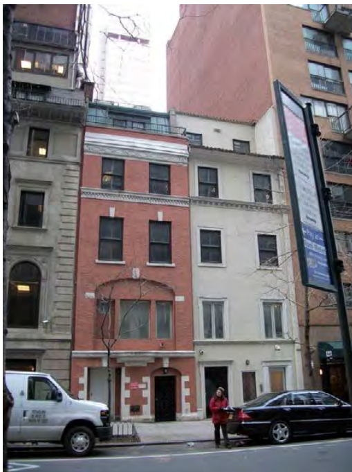
Photo 111: 119 East 54th Street, townhouses (S/NR-Eligible district: PROJECT AREA)
