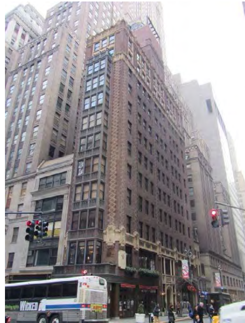
Photo 124: 299 Madison Avenue (NYCL-Eligible: PROJECT AREA)
