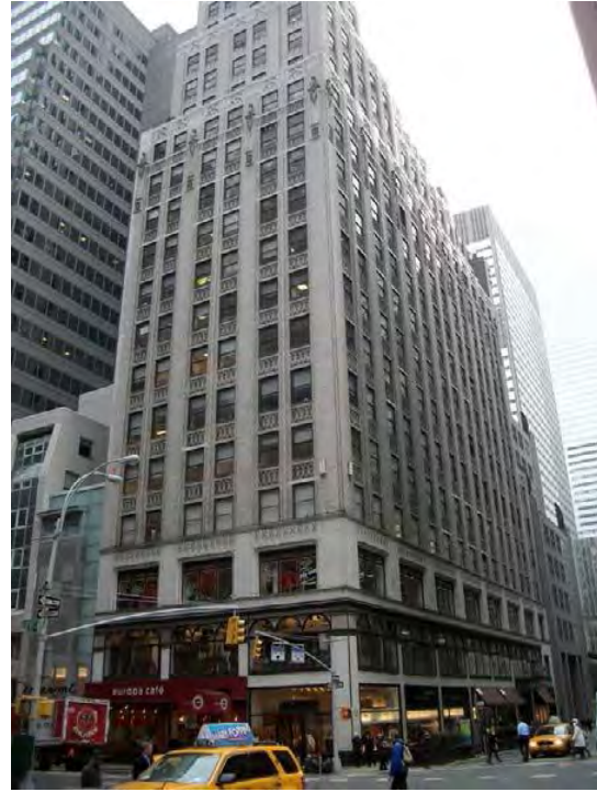
Photo 142: 515 Madison Avenue, Dumont Building (S/NR- Eligible: PROJECT AREA)
