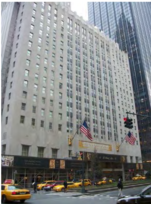
Photo 42: 301 Park Avenue, Waldorf-Astoria Hotel (NYCL, S/NR-Eligible)
