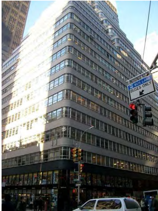
Photo 29: 488 Madison Avenue, Look Building (NYCL, S/NR)
