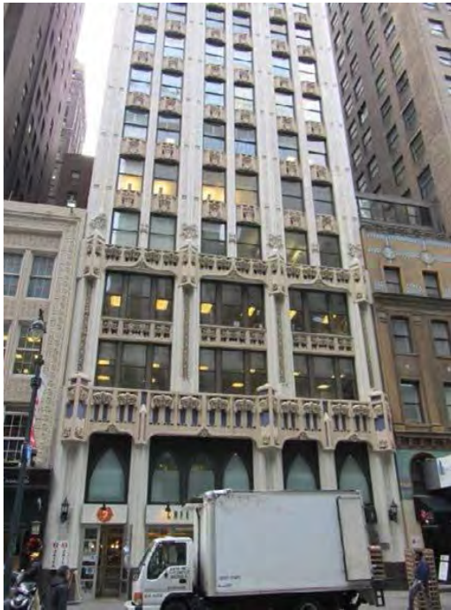
Photo 80: 18-20 East 41 st Street (NYCL)
