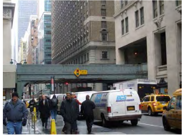
Photo 98: East 45th Street bridges, part of Park Avenue Viaduct, north of Grand Central Terminal and MetLife Building (S/NR-Eligible: PROJECT AREA)
