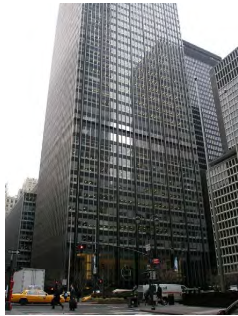
Photo 130: 270 Park Avenue, The Chase Building (aka The Union Carbide Building) (NYCL-Eligible: PROJECT AREA)
