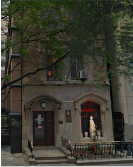
Photo 97: 141 East 43rd Street, Saint Agnes Rectory (S/NR-Eligible: PROJECT AREA)
