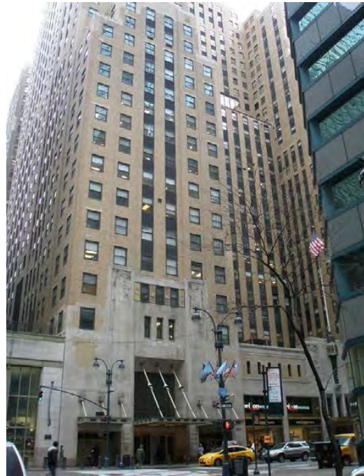
Photo 61: 420 Lexington Avenue, Graybar Building (NYCL, S/NR)
