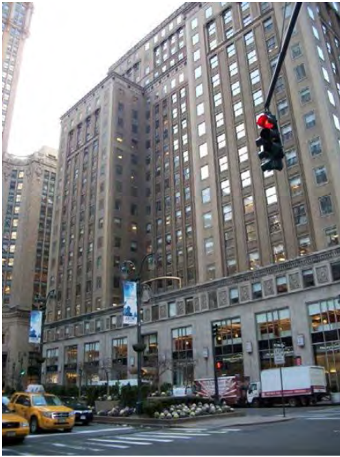
Photo 129: 250 Park Avenue, Postum Building (NYCL and S/NR-Eligible: PROJECT AREA), Projected Development Site 6
