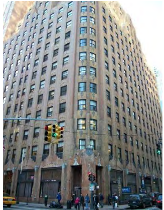
Photo 34: 566-570 Lexington Avenue, General Electric Building (NYCL, S/NR)
