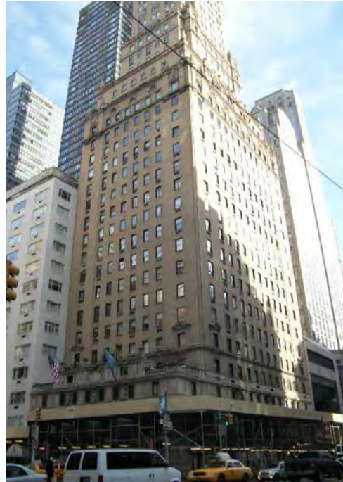
Photo 6: 465 Park Avenue, Ritz Tower 1 (NYCL, S/NR-Eligible)
