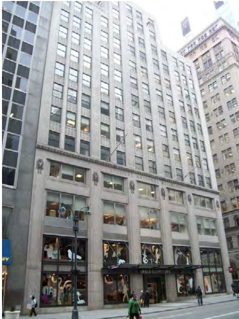
Photo 121: 521 Fifth Avenue, Lefcourt-National Building (NYCL-Eligible: STUDY AREA)
