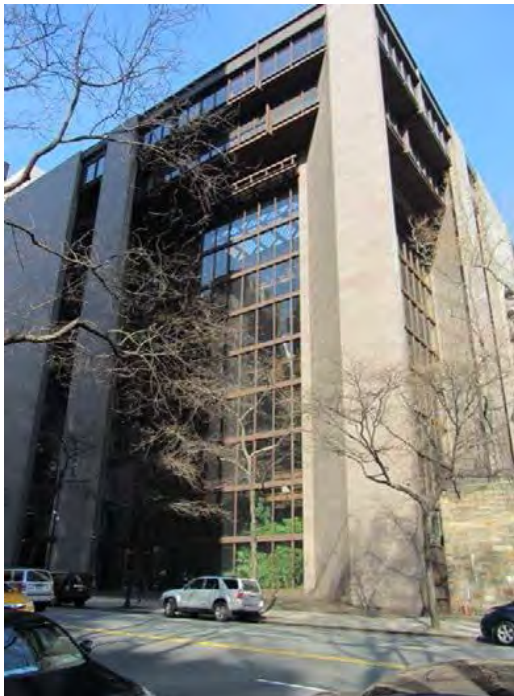
Photo 70: 303 East 42 nd Street, Ford Foundation Building (NYCL)
