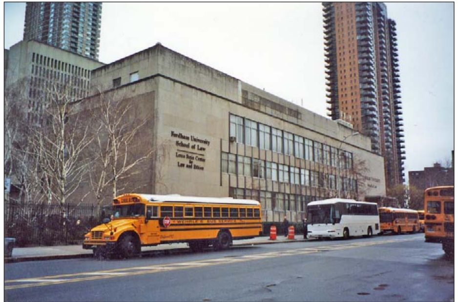
View southwest on West 62nd Street 3
