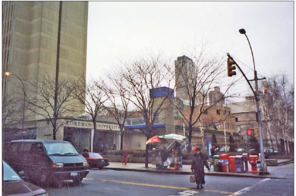
View northwest of the project site's Columbus Avenue frontage. The Lowenstein Center is on the left. The Law School is on the right 5
