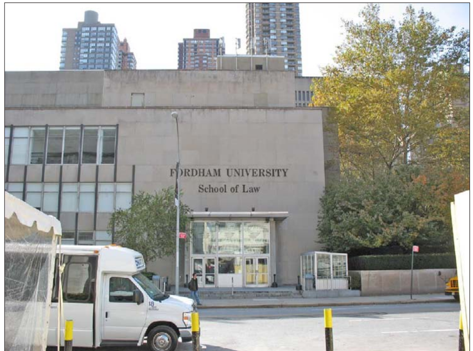
Law School entrance view south across West 62nd Street
