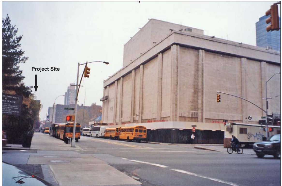
View west on West 62nd Street from Columbus Avenue. 22 The project site is on the left.
