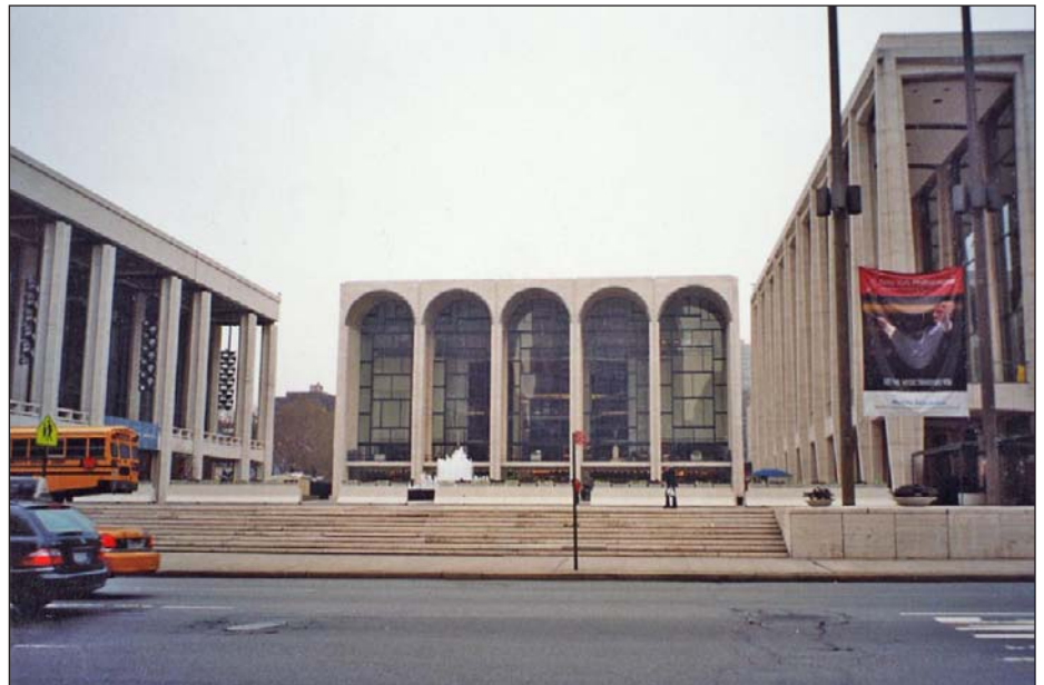
View west of Lincoln Center from Columbus Avenue. Josie Robertson Plaza is in the middle. The Metropolitan Opera House is behind it. The Koch Theater is on the left. Avery Fisher Hall is on the right. 12
