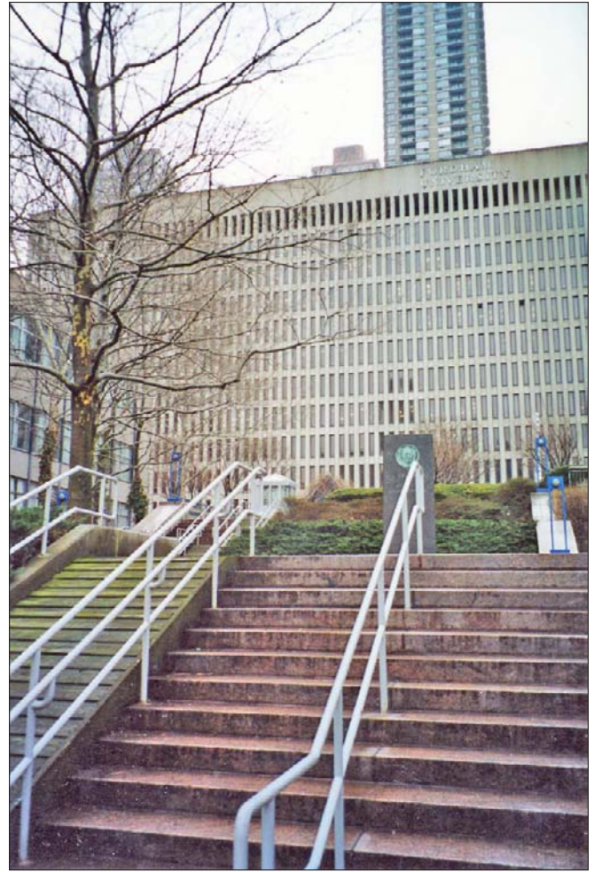
View south from West 62nd Street. The north facade of Lowenstein Center is visible beyond the podium. The Law School is on the left.
