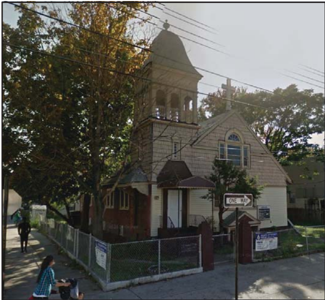
11) Glenmore Avenue Presbyterian Church (S/NR-Eligible & NYCL-Eligible)
