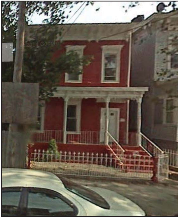
14) 277 Vermont Street (S/NR-Eligible & NYCL-Eligible)
