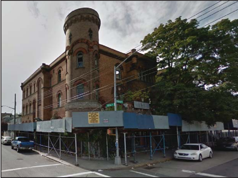
3) 75th Police Precinct Station House (S/NR; NYCL-Eligible)
