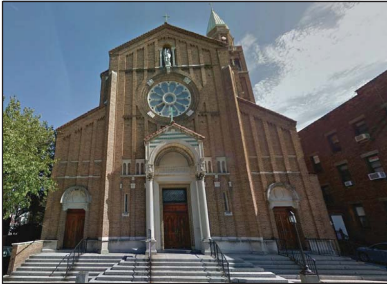
6) St. Michael's R.C. Church (S/NR-Eligible & NYCL-Eligible)
