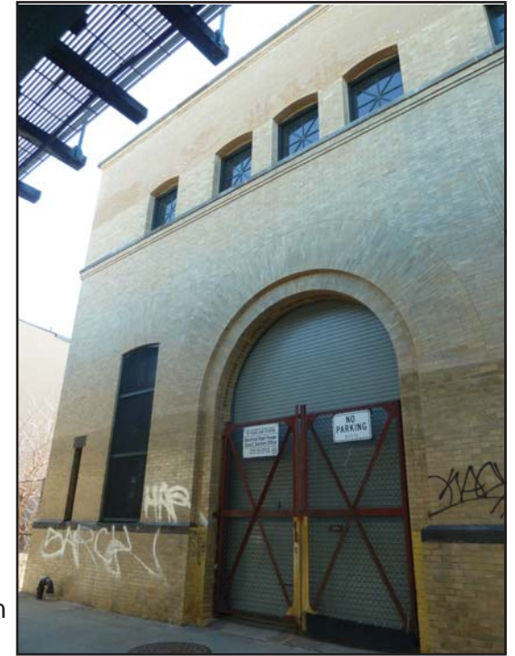
4) BMT Substation #401 (S/NR)
