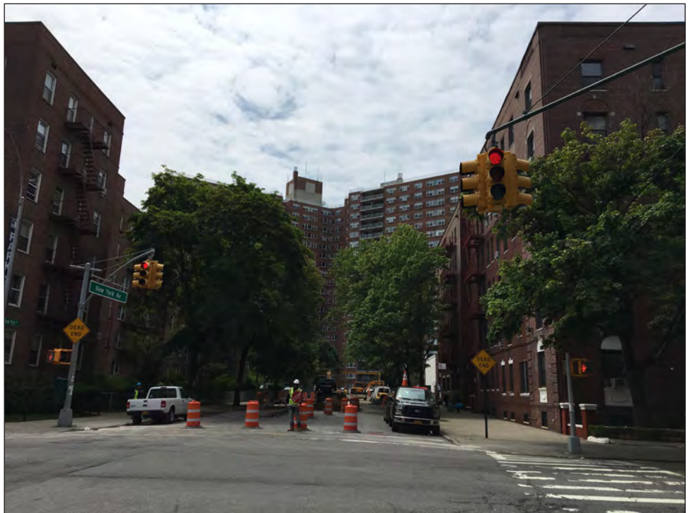
View facing south on New York Avenue from Avenue H looking toward the Philip Howard Apartments
