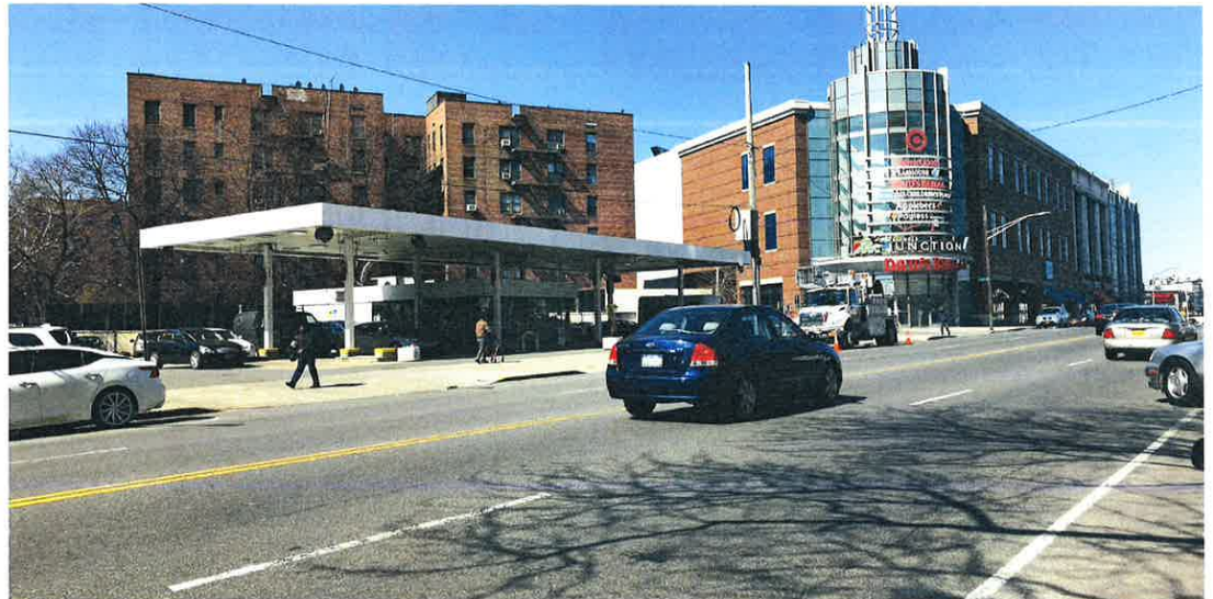
02 VIEW WEST ACROSS FLATBUSH AVE.
