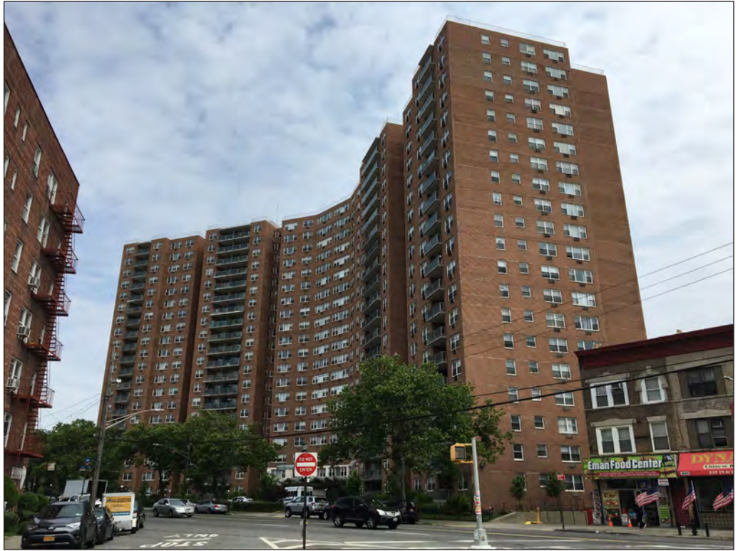
Philip Howard Apartments; 7 View facing east from the corner of Flatbush Avenue and Avenue I.
