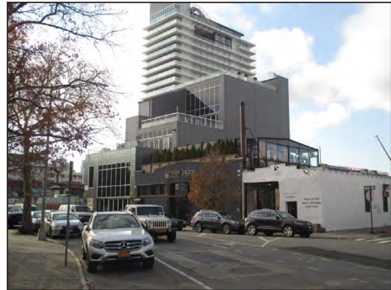
12.) Looking south from the intersection of Nassau Avenue and North 14th Street towards Berry Park (restaurant/bar). The William Vale Hotel can be seen in the background
