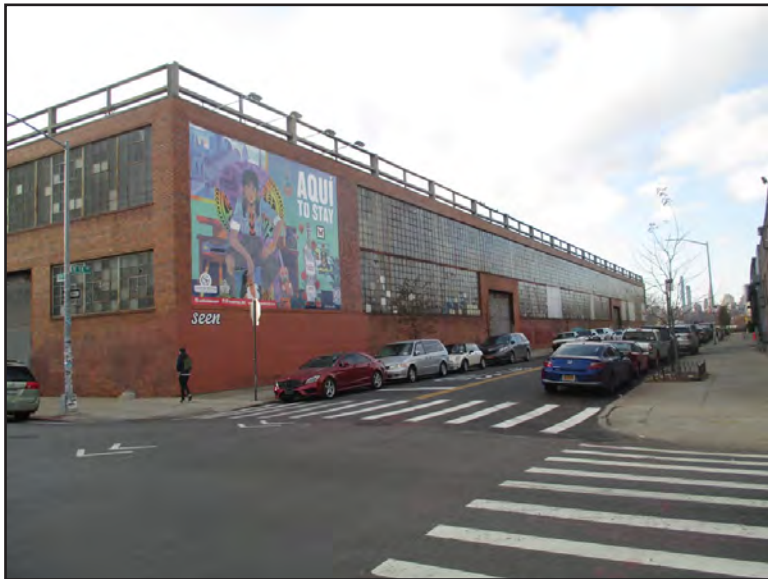
11.) Looking west from the intersection of Wythe Avenue and North 14th Street towards a storage/warehouse use
