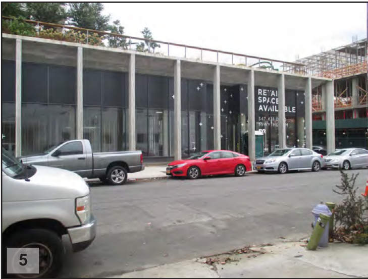
5) Looking south at the William Vale Hotel from the Proposed Development Site
