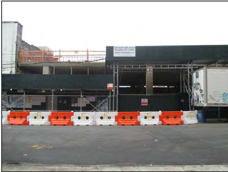
1.) The development site, looking north from North 13th Street
