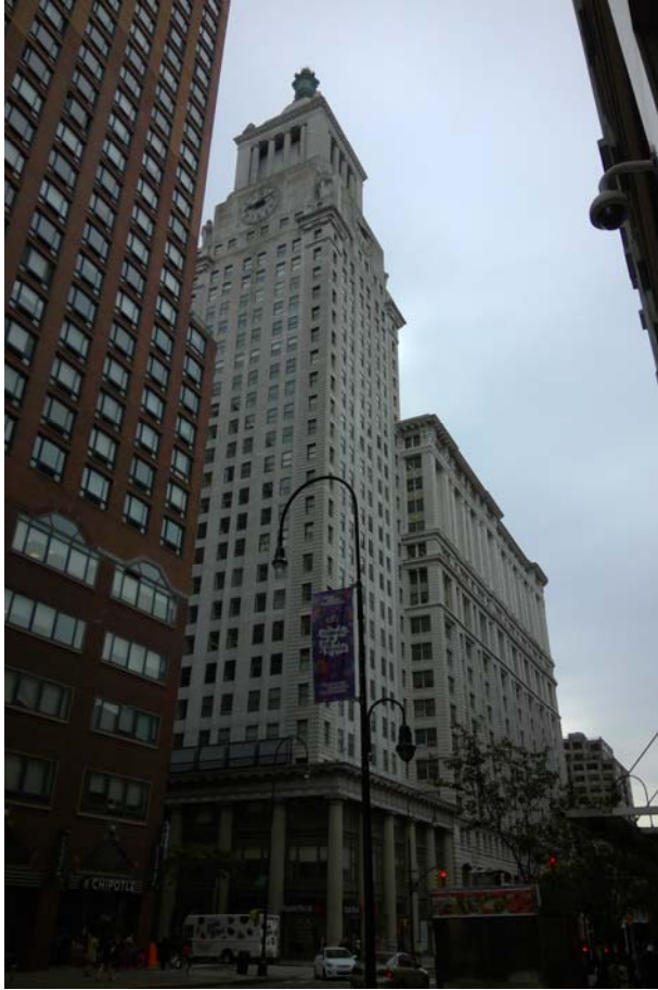
Photo 2.3-16 (2017): Consolidated Edison Building (2017)
