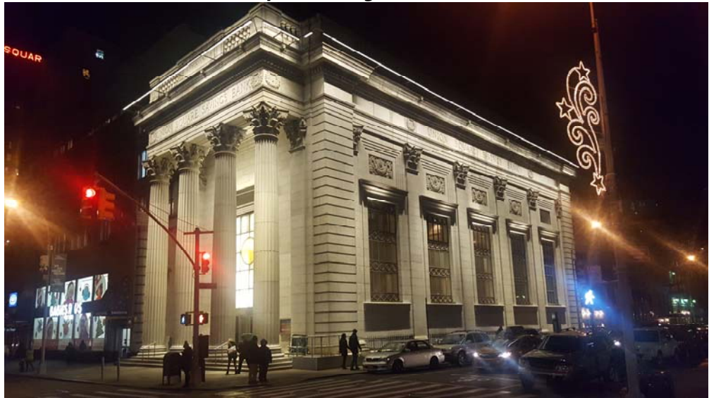
Photo 2.3-10 (2017): Union Square Savings Bank (2017)
