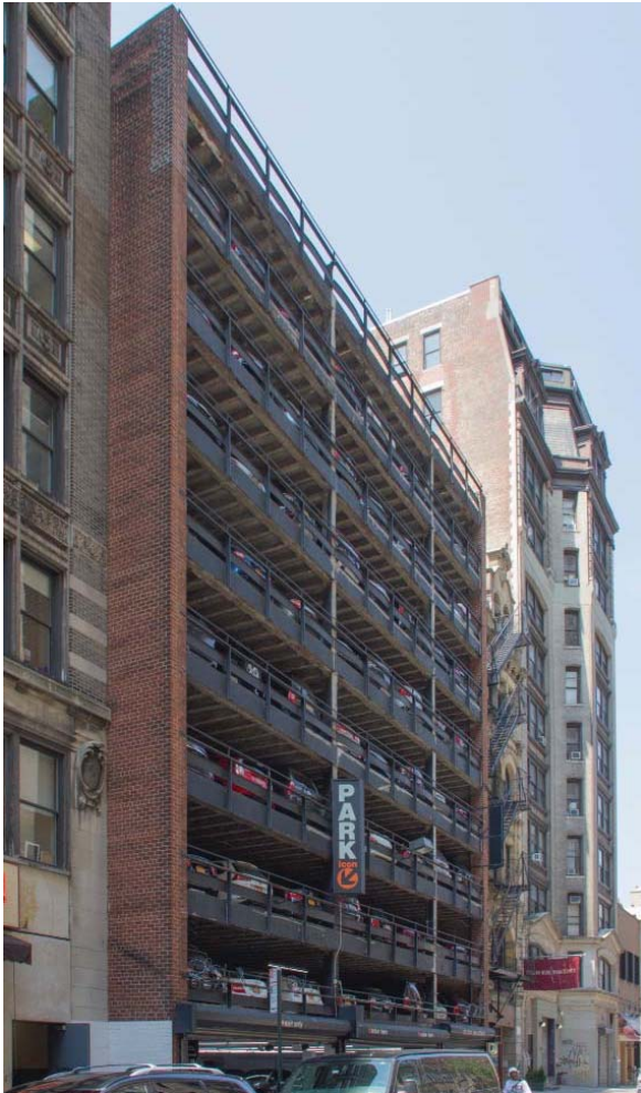
View west along E 16th Street towards Lot 74
