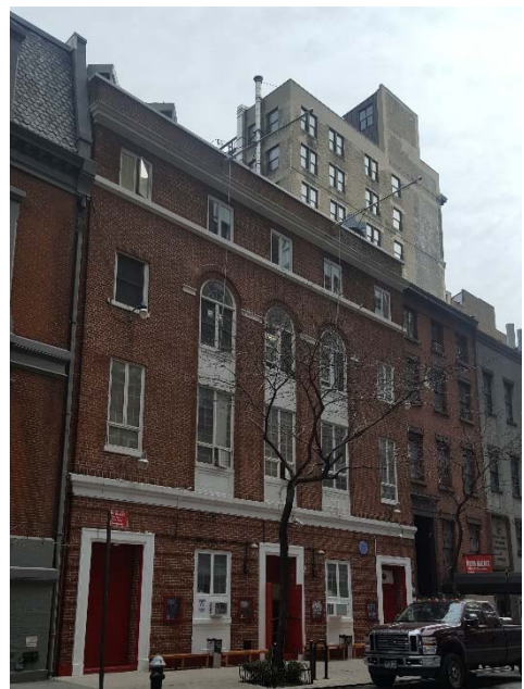
Photo 2.4-4 View of southern façade on Lot 12, which is one of three tax lots in the Affected Area
