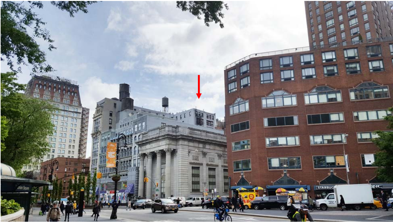
Figure 2.4-5: No-Action Condition View from southern Union Square Park (would not be visible)
