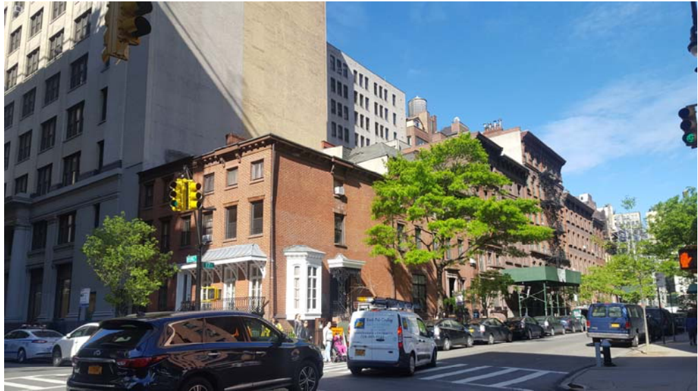
Photo 2.3-13: East 17th Street/Irving Place Historic District (2017)
