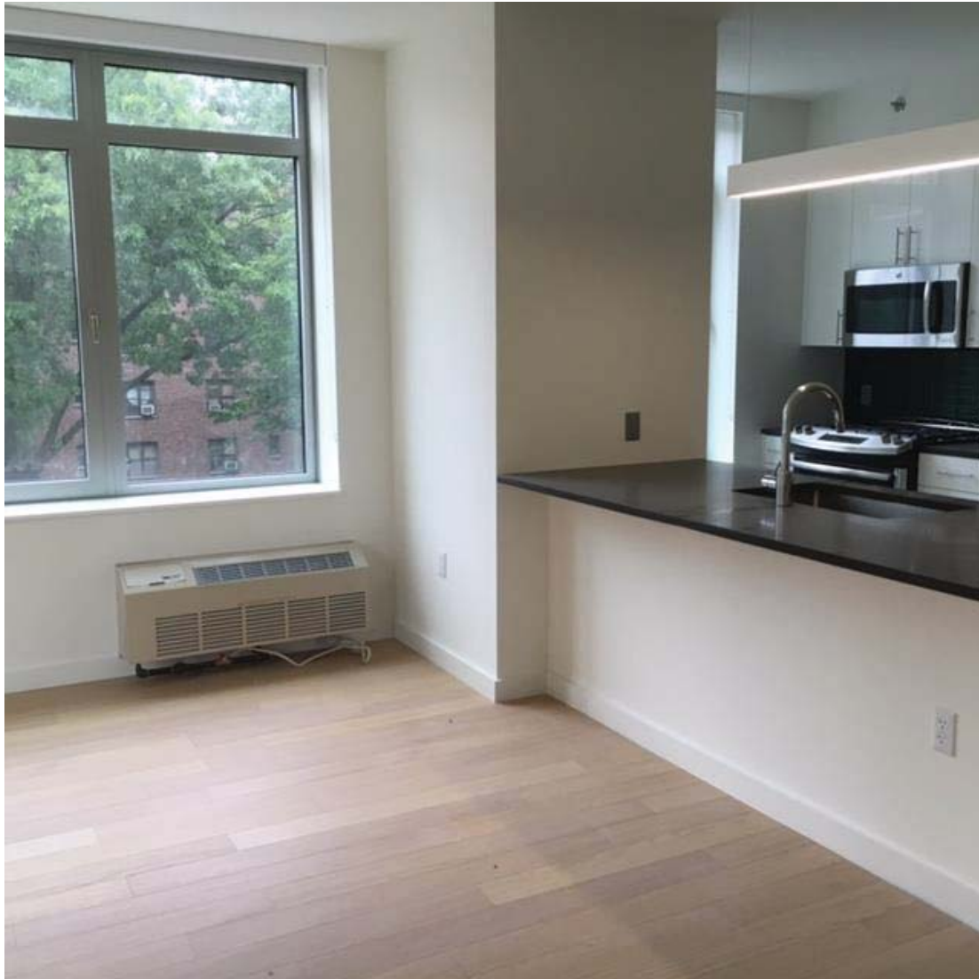
Interior of Apartment 3A showing PTAC and Apartment Window
