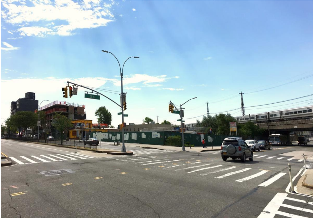
Photograph 3: At the intersection of Queens Boulevard and 69th Street, looking southwest at the Development Site
