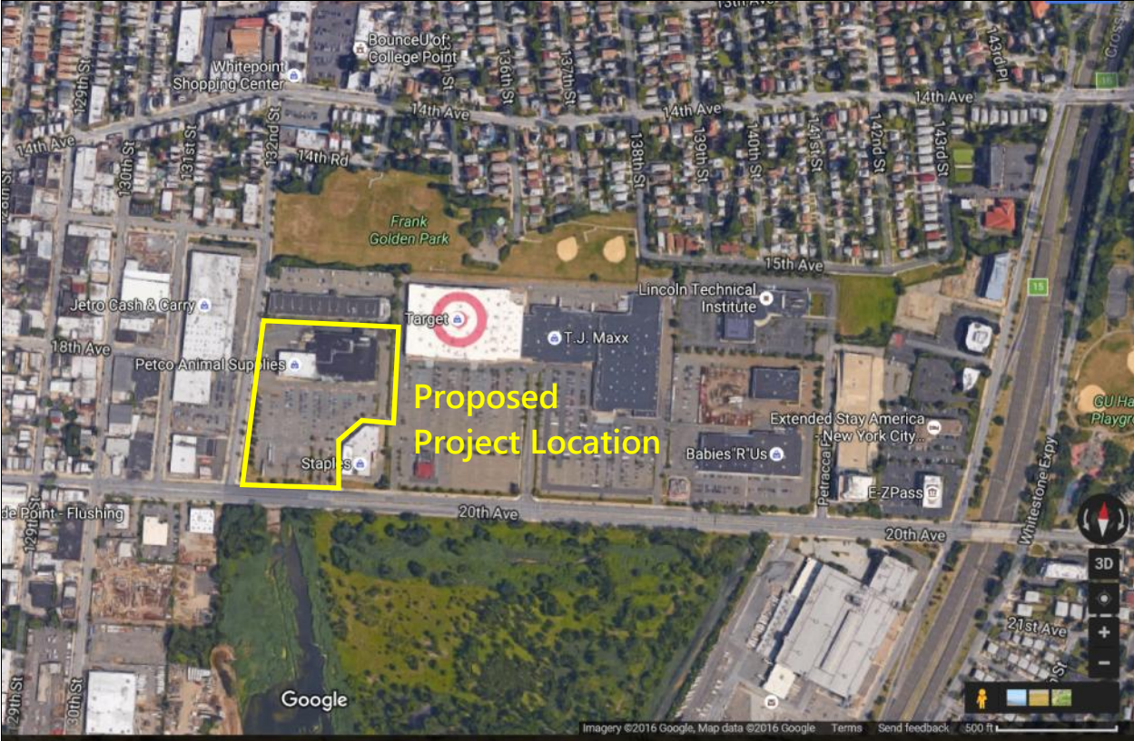
Figure 12. Current aerial image showing the project location with existing parking lot and other extensive development built over the filled-in marshland. The Flushing Airport to the south has sunken back into marshland. Source: http://gis.nyc.gov/doitt/nycitymap/
