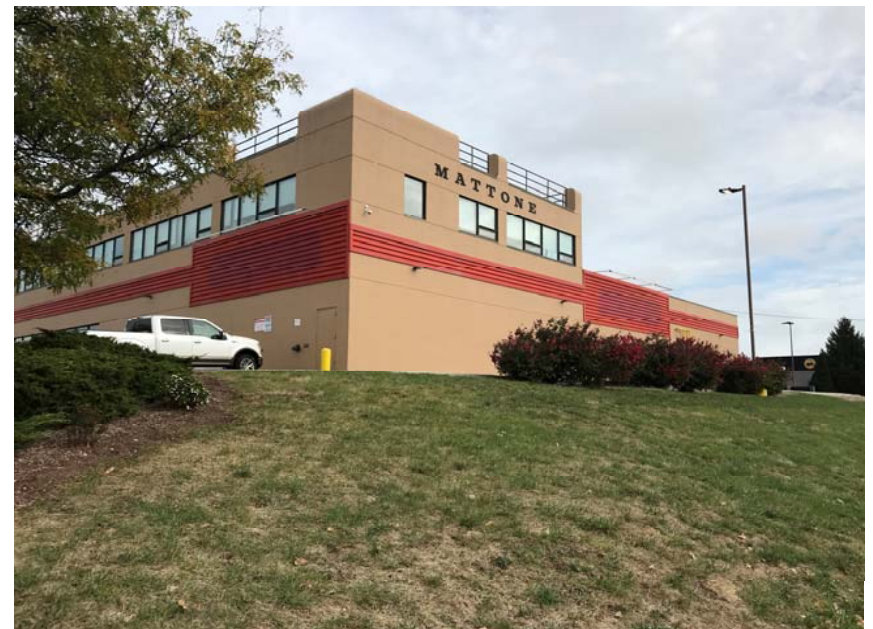
4. View looking towards adjacent site within the Shopping Center
