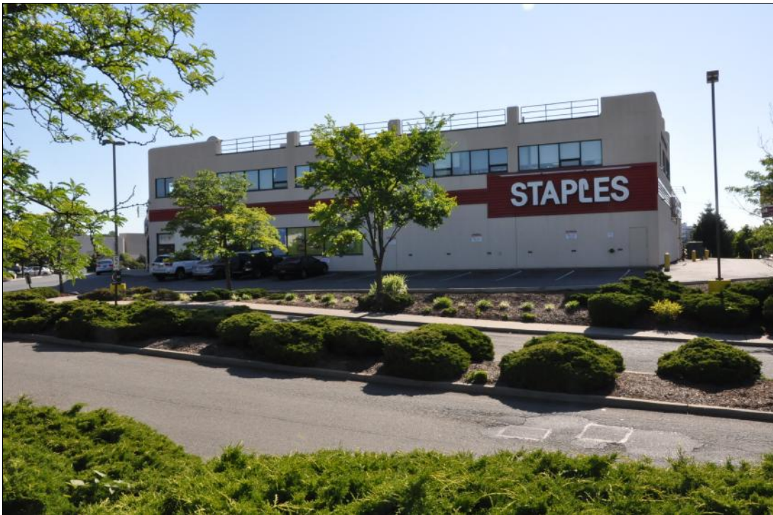
PHOTO 4. Facing northeast across the existing parking lot/project area towards retail outlet located off of APE's eastern corner.
