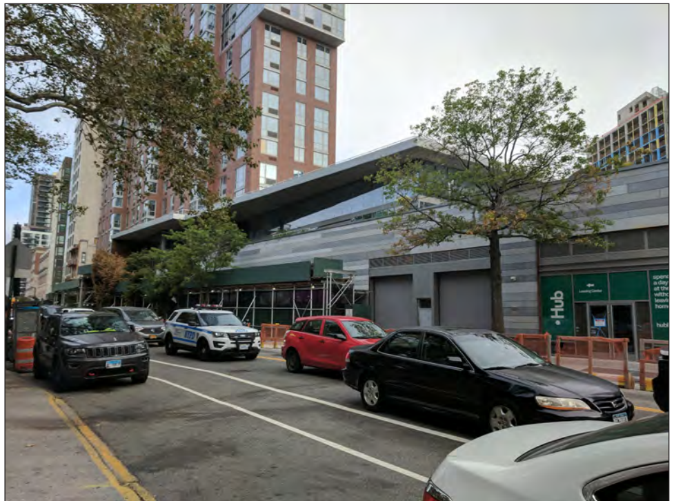
The one- to three-story base of 333 Schermerhorn Street. View from Schermerhorn Street west of 3rd Avenue facing northwest.
