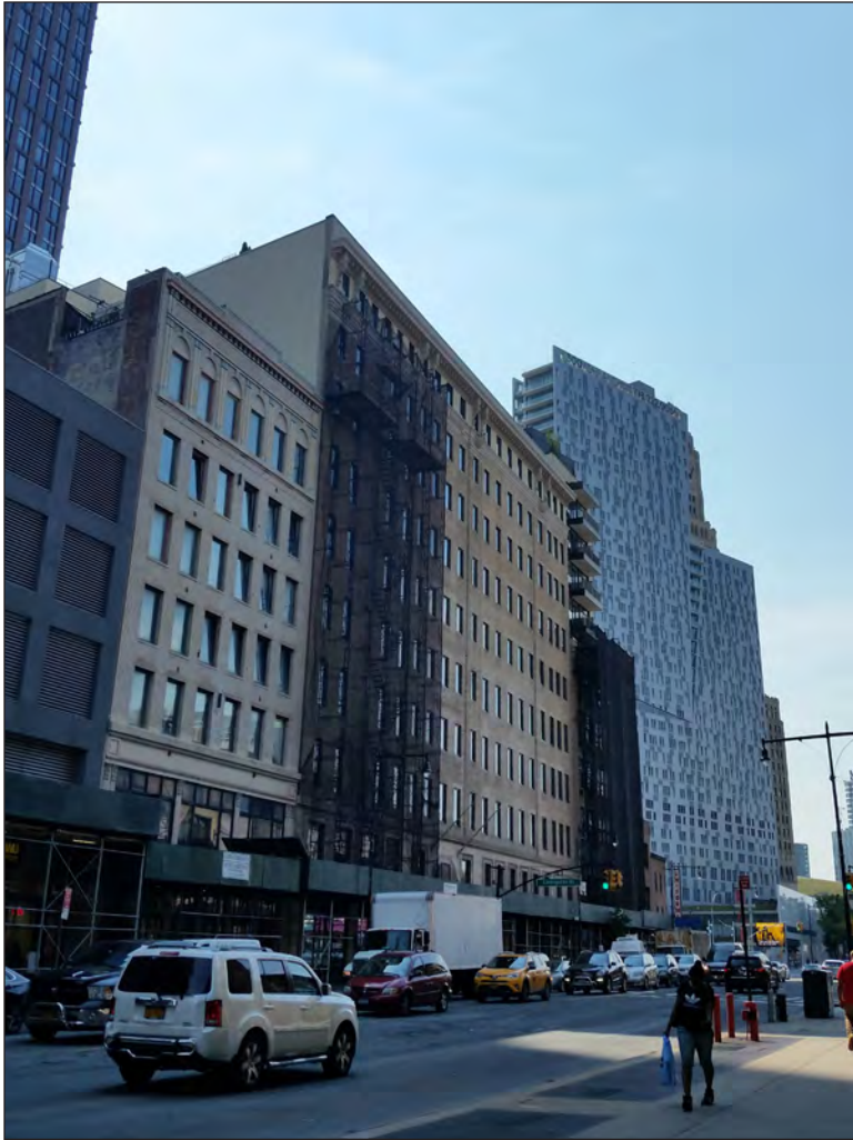
Pioneer Warehouse, 37-53 Flatbush Avenue 1
