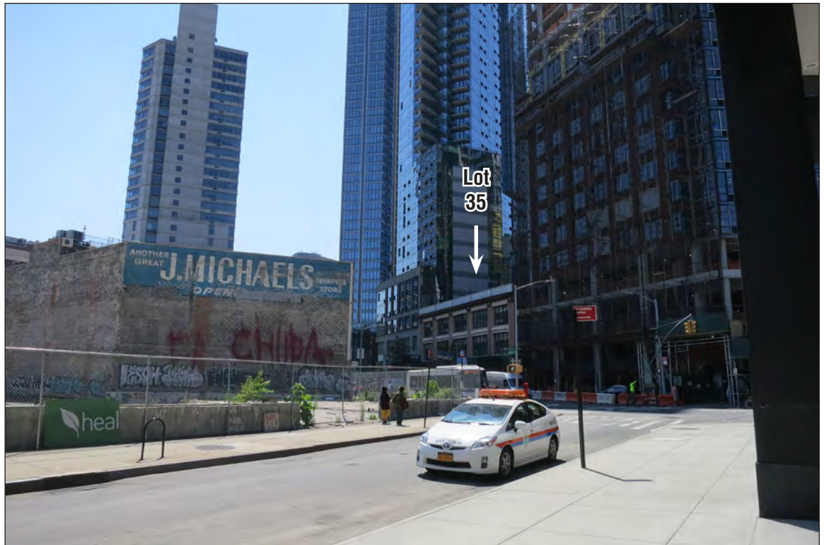
The view from Hudson Avenue facing southeast includes a vacant lot, the Project Area, 250 Ashland Place, and 230 Ashland Place.
