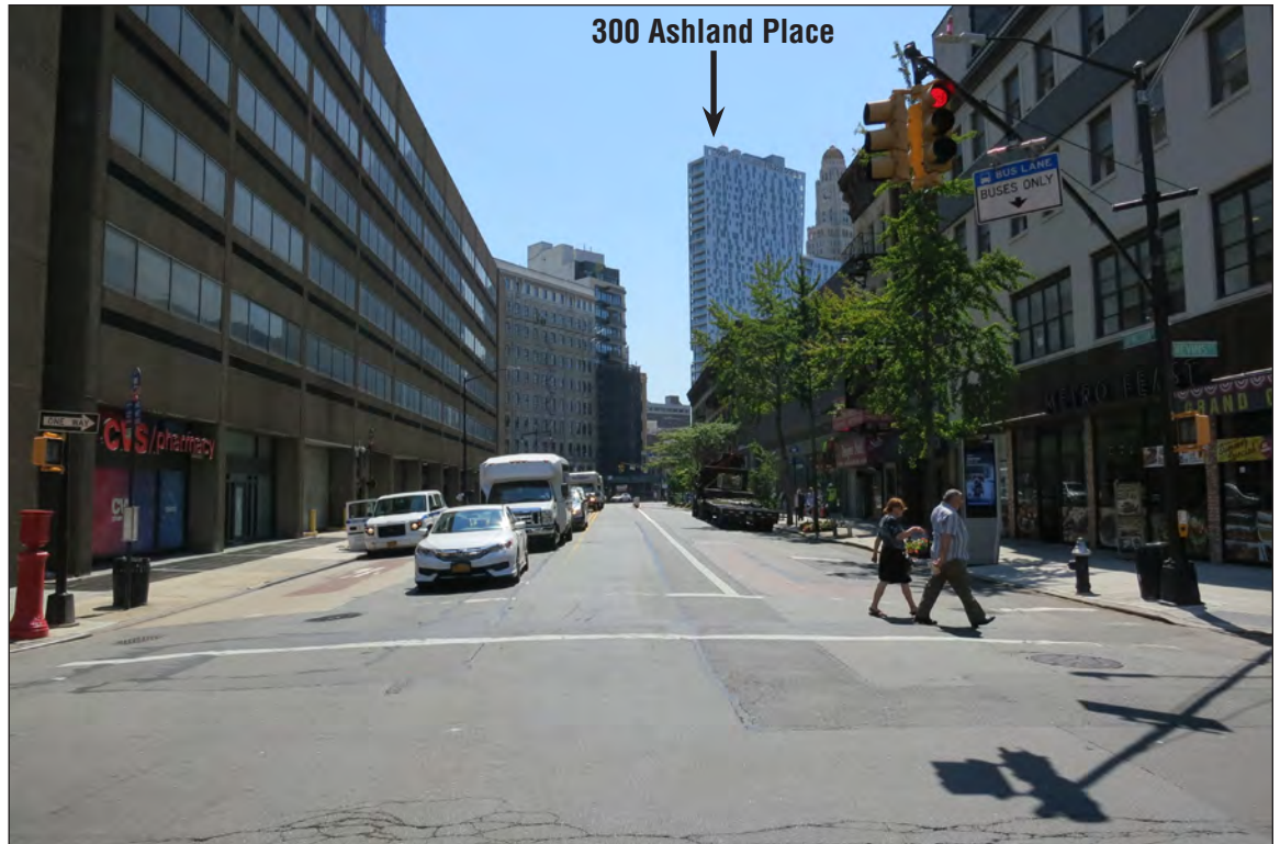
The view from Livingston Street at Nevins Street facing east with 38 Flatbush Avenue on the left and the recently constructed 300 Ashland Place in the background on the right. The domed tower of the former Williamsburgh Savings Bank Tower can be seen behind 300 Ashland Place.
