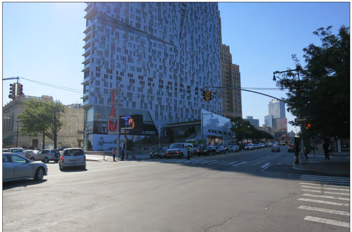
Views south along Flatbush Avenue near Lafayette Avenue include the recently constructed building at 300 Ashland Place and longer views of the Pacific Park development. 18
