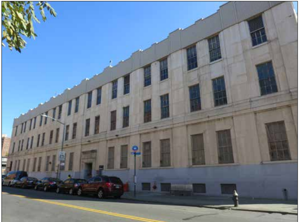
The Verizon Telephone Building located along Rockaway Avenue 14
