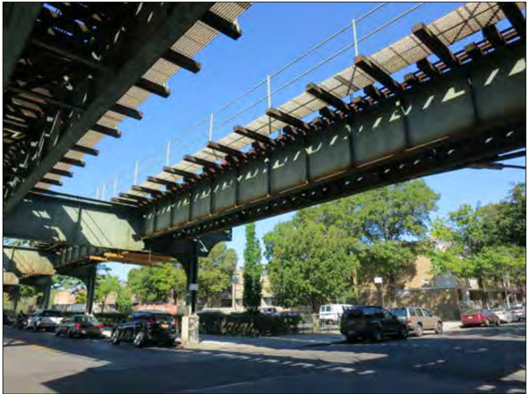
View northwest from Livonia Avenue and Chester Street to Site B 2
