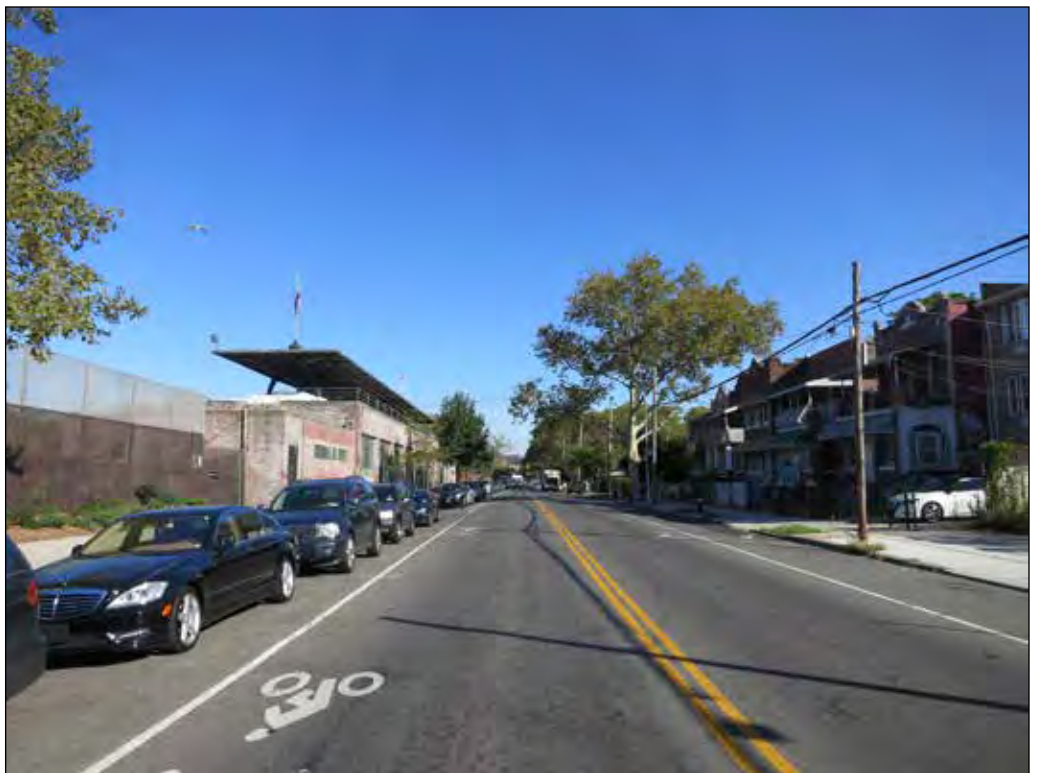
View looking north on Thomas S. Boyland Street. Bicycle markings and parking ribbons are on both sides of the street 10
