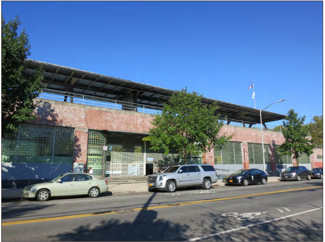
View northwest of the exterior of the Betsy Head Park bath house along Thomas S Boyland Street 3
