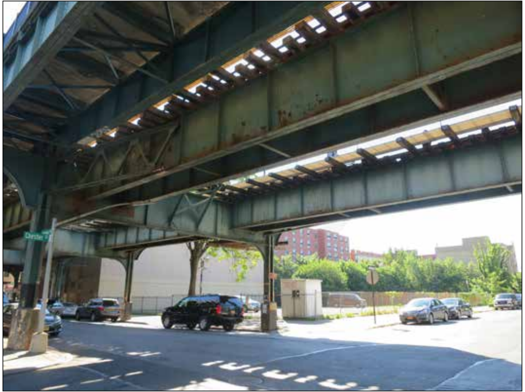
View southeast from Livonia Avenue and Chester Street to Site A 1
