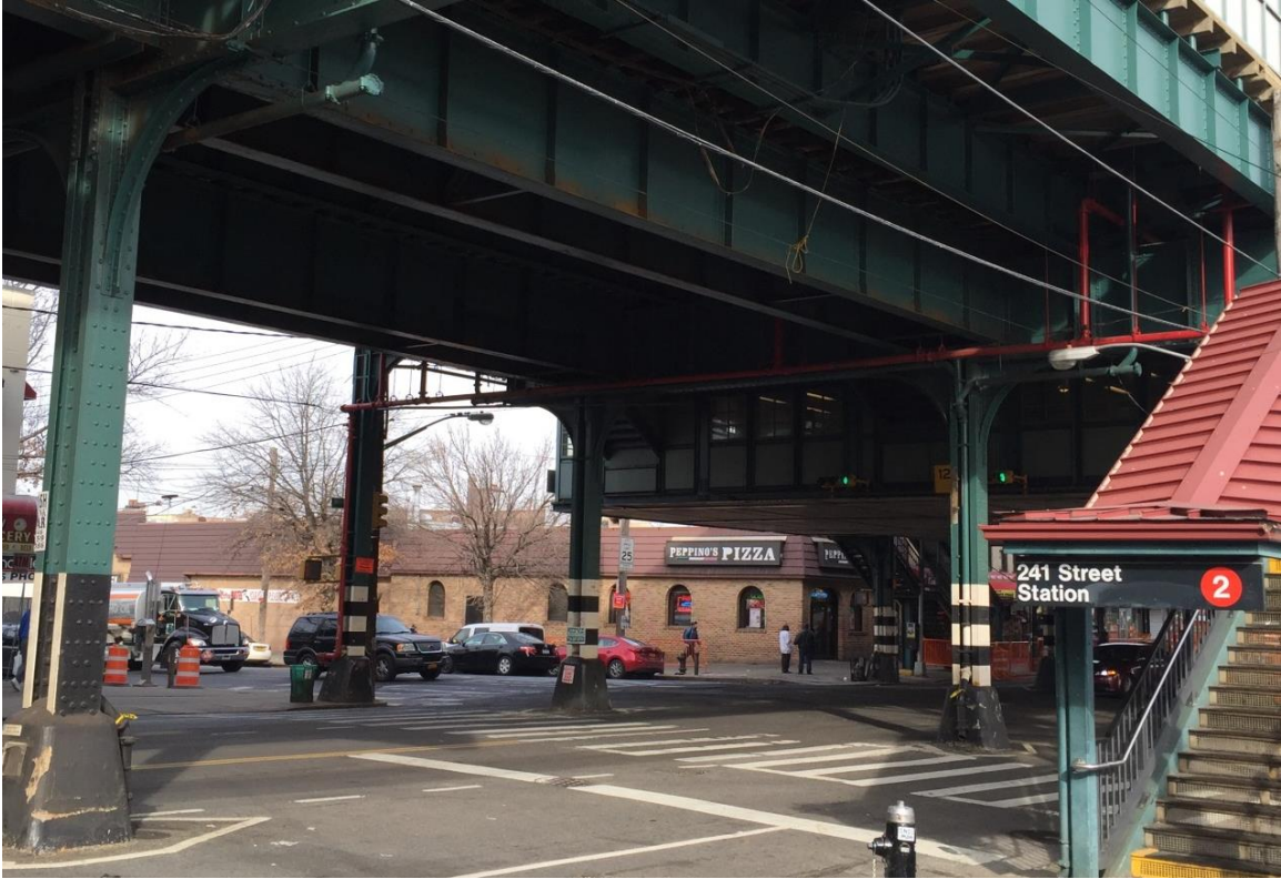
Photograph 5: North view of No. 2 train Wakefield 241st Street entrance from Project Site
