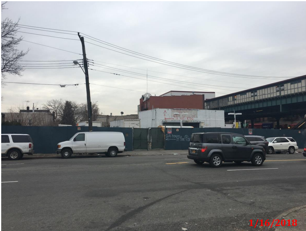
Photograph 24: South view of Project Site from intersection of Cranford Avenue and East 241st Street
