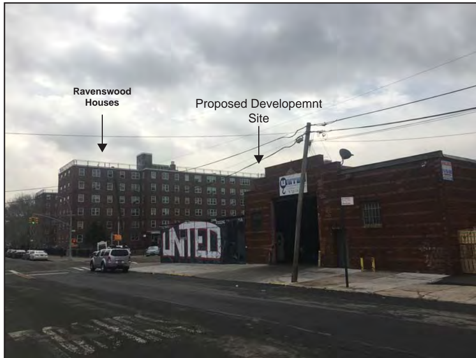
Photo 1: View southeast across 35th Avenue at the northern edge of the proposed rezoning area and proposed development site
