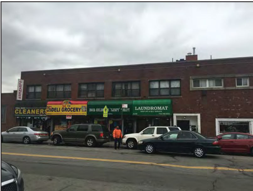
iii. Commercial buildings on 36th Avenue
