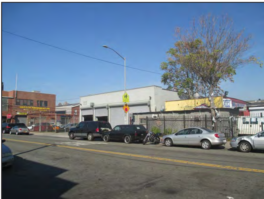
x. Industrial building on 35th Avenue
