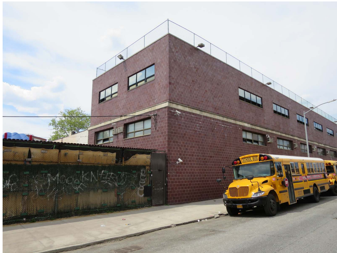
18. View of the Site facing northwest from McDonald Avenue.
