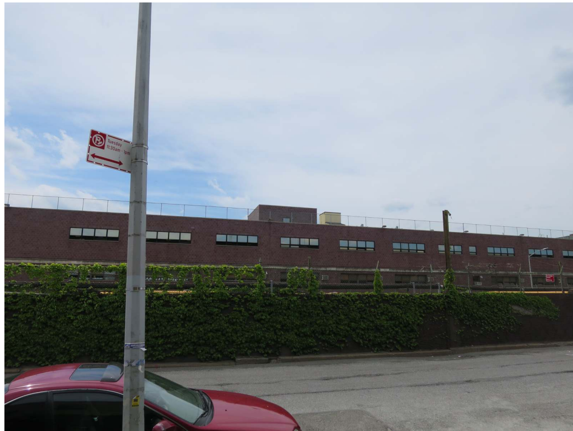
30. View of the Site facing northwest from McDonald Avenue.
