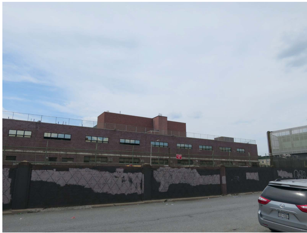
25. View of the Site facing northwest from McDonald Avenue.
