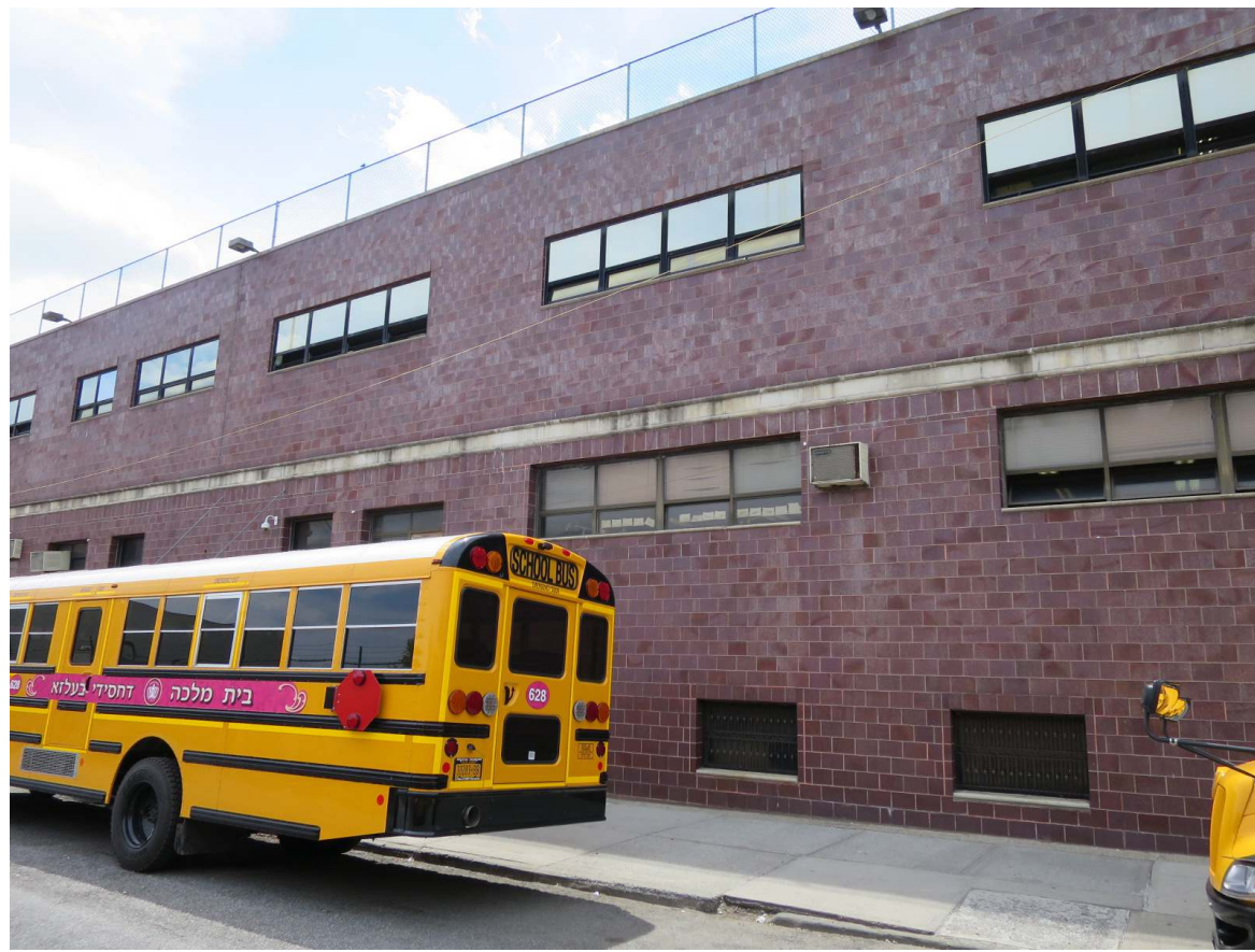
22. View of the Site facing southwest from McDonald Avenue.
