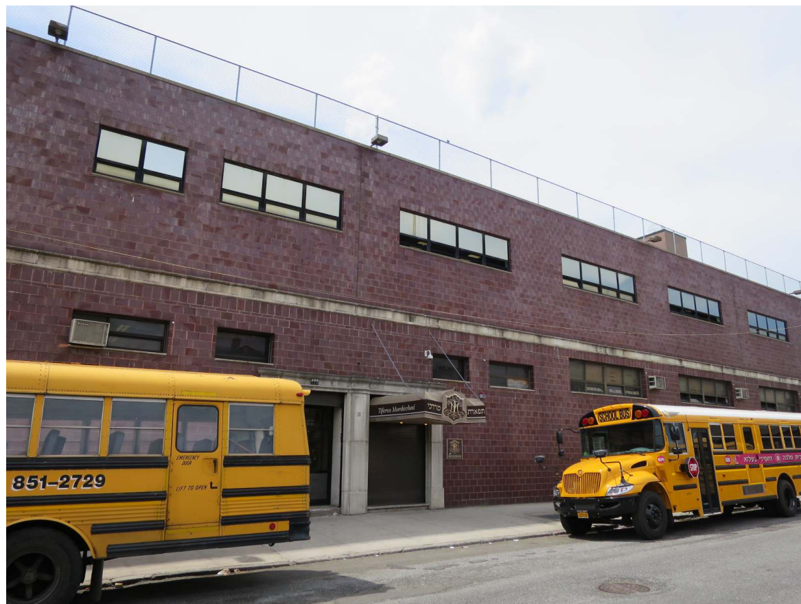
21. View of the Site facing northwest from McDonald Avenue.
