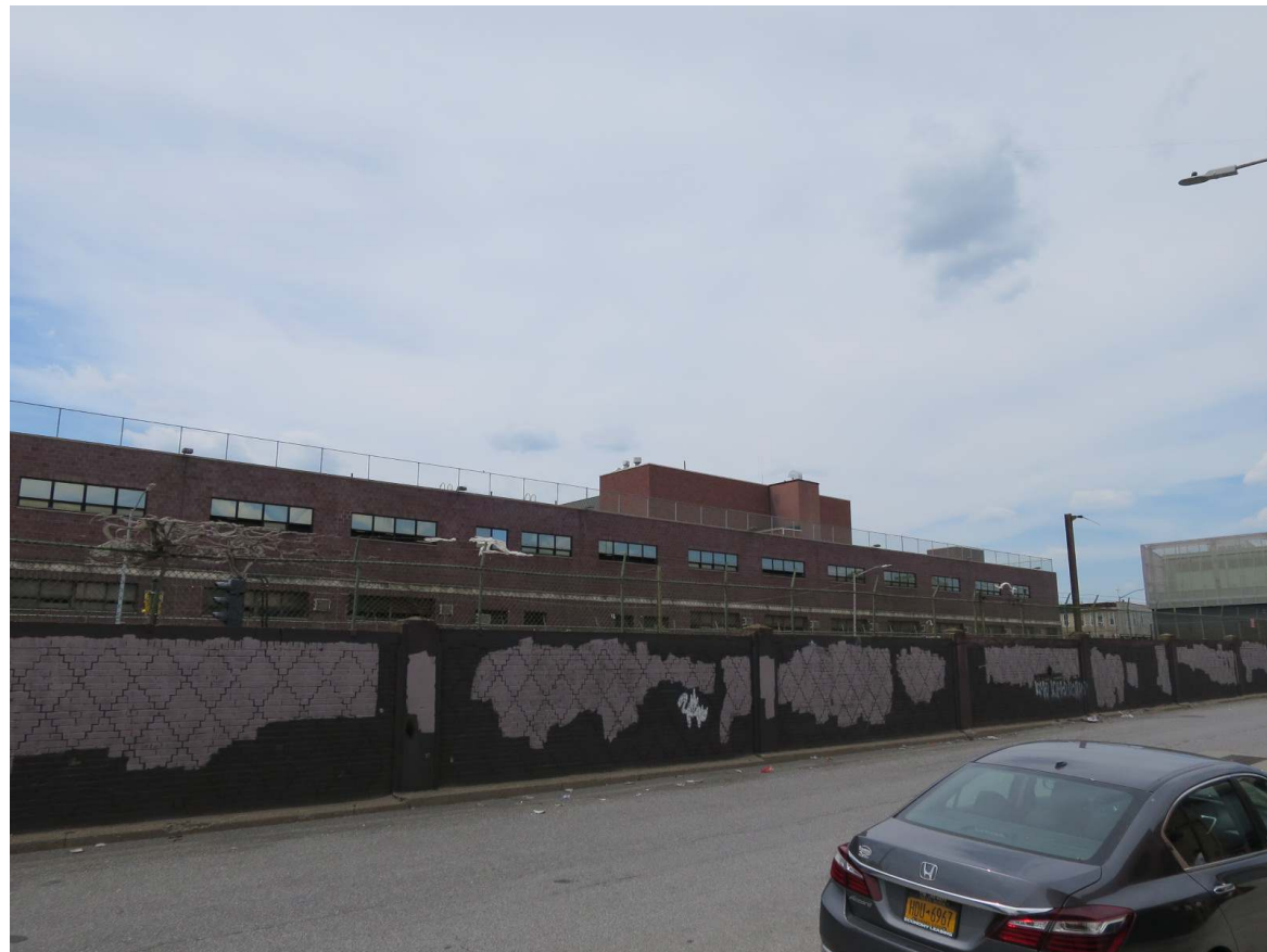
27. View of the Site facing northwest from McDonald Avenue.
