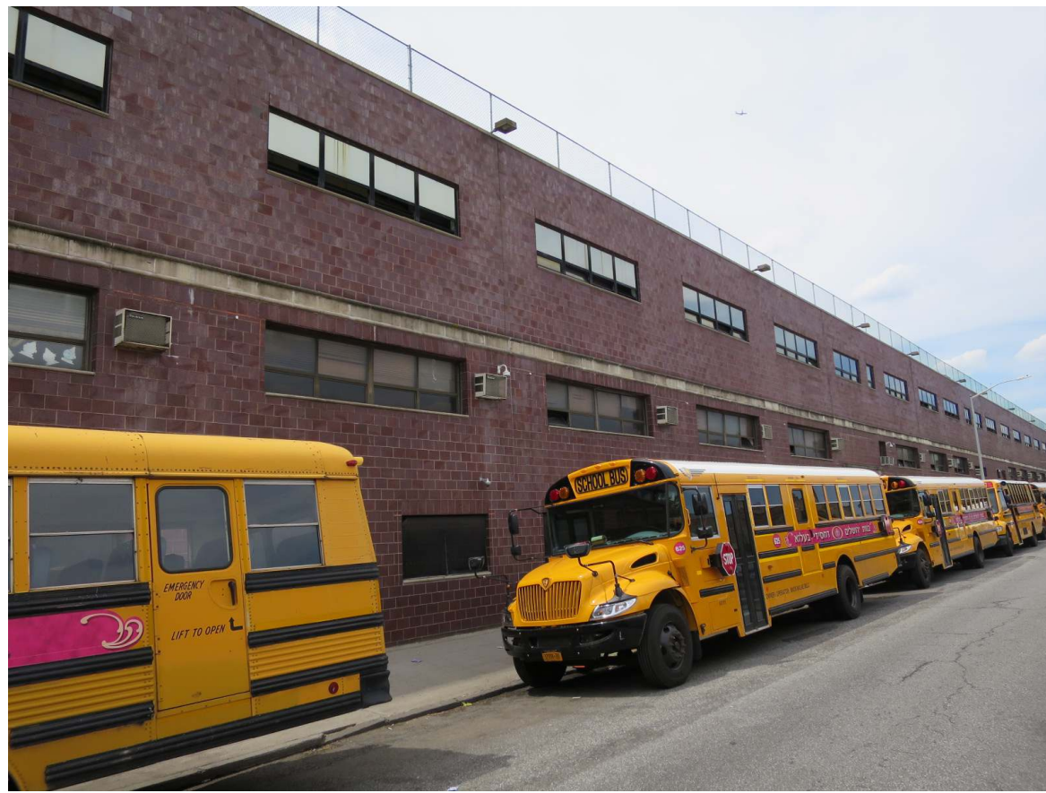
19. View of the Site facing northwest from McDonald Avenue.
