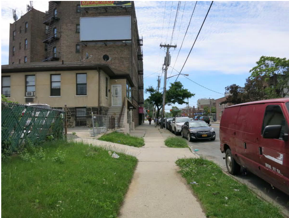
Photo 3: View of Projected Development Site 1 (Lot 8) from Williamsbridge Road looking southeast.
