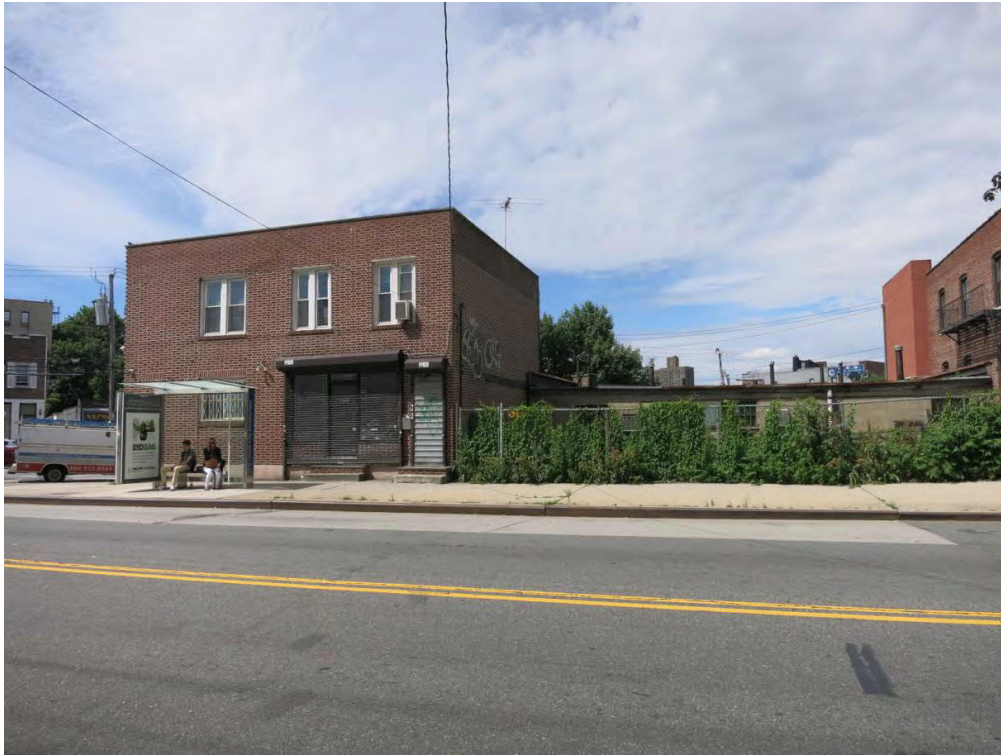
Photo 9: View of the west side of Williamsbridge Road between Allerton Avenue and Radcliff Avenue facing southwest.
