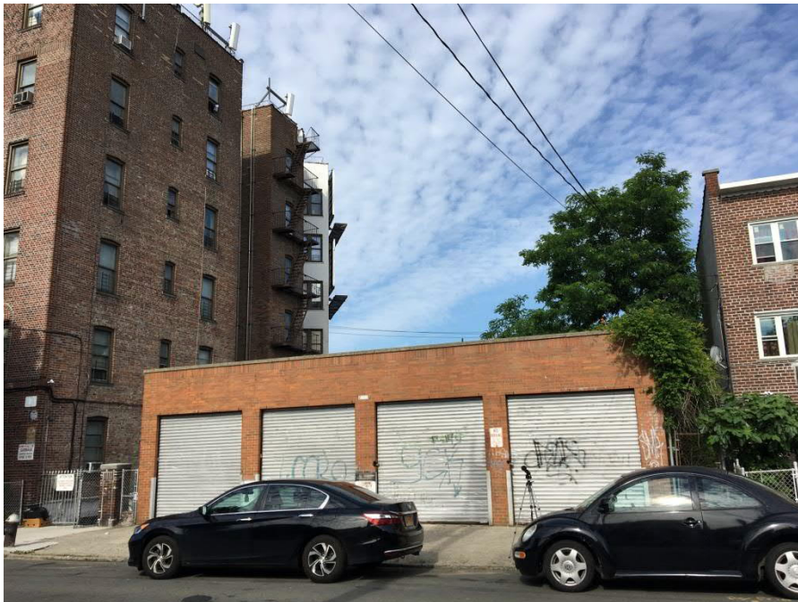
Meter Setup at Location 2
