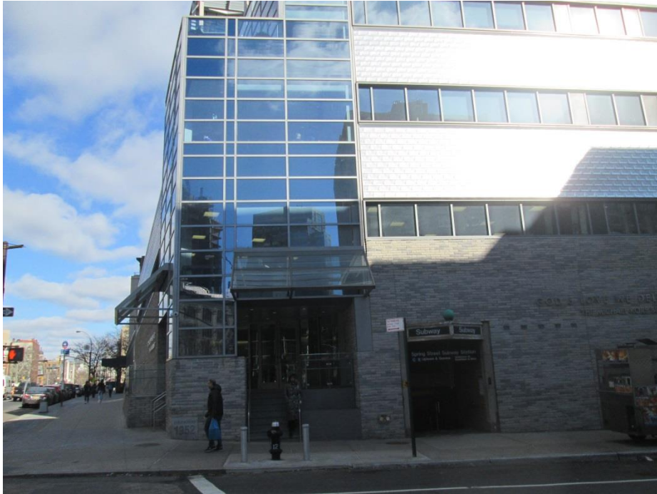
Photo 5: View of adjacent lot with the Project Site in the background from the corner of Avenue of the Americas and Spring Street looking northeast.
