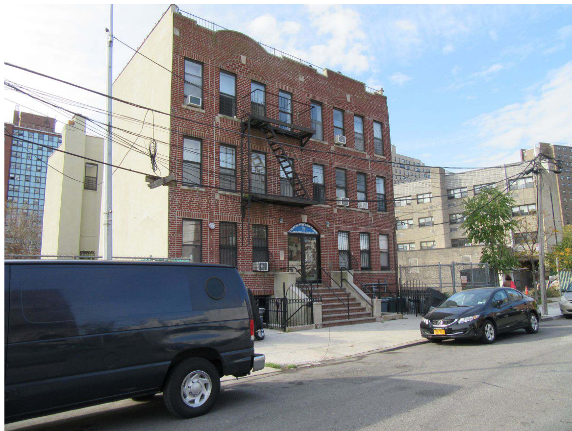
30. View of the side of West 23rd Street facing northwest.
