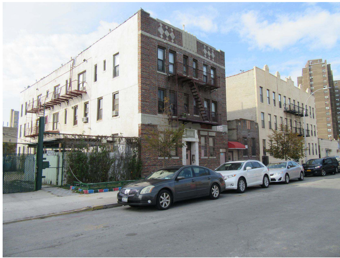
7. View of the Site facing northwest from West 22nd Street.
