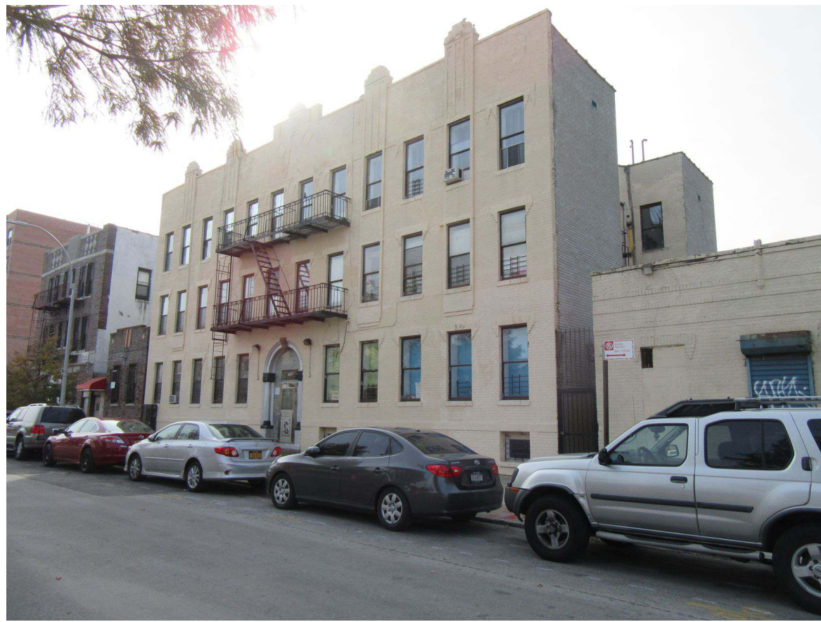
10. View of the side of West 22nd Street facing southwest.
