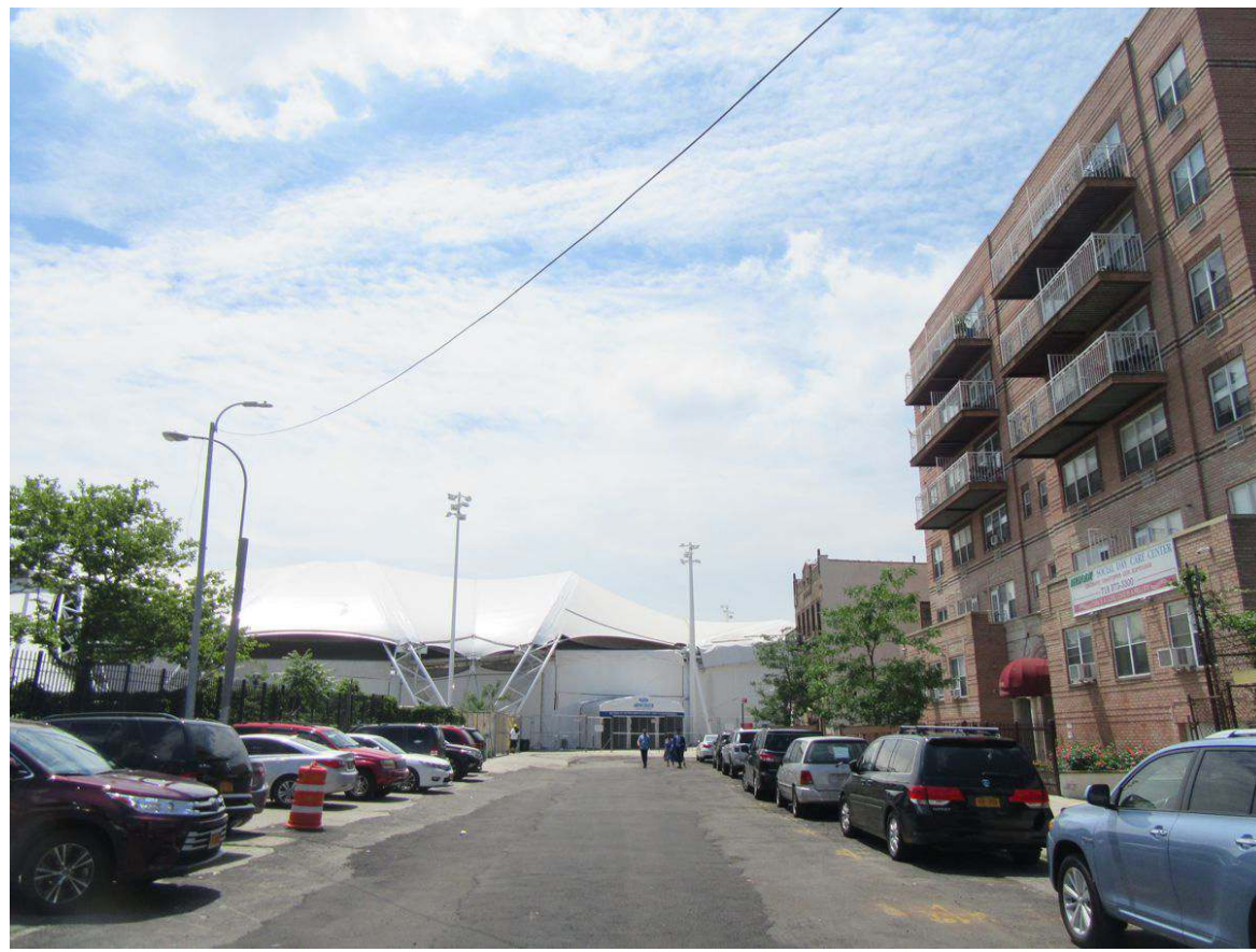
1. View of the amphitheater facing south on West 22nd Street.
