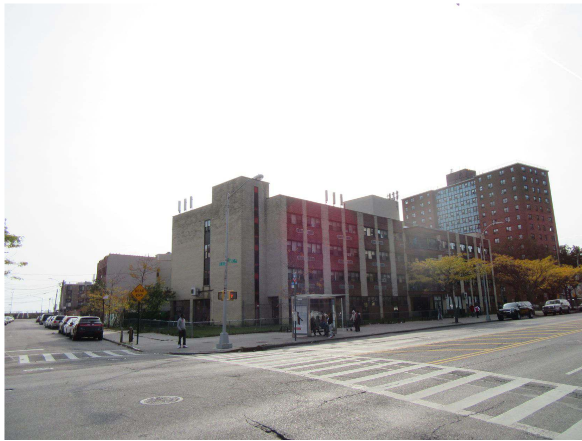
22. View of the side of Surf Avenue facing southwest from West 23rd Street.
