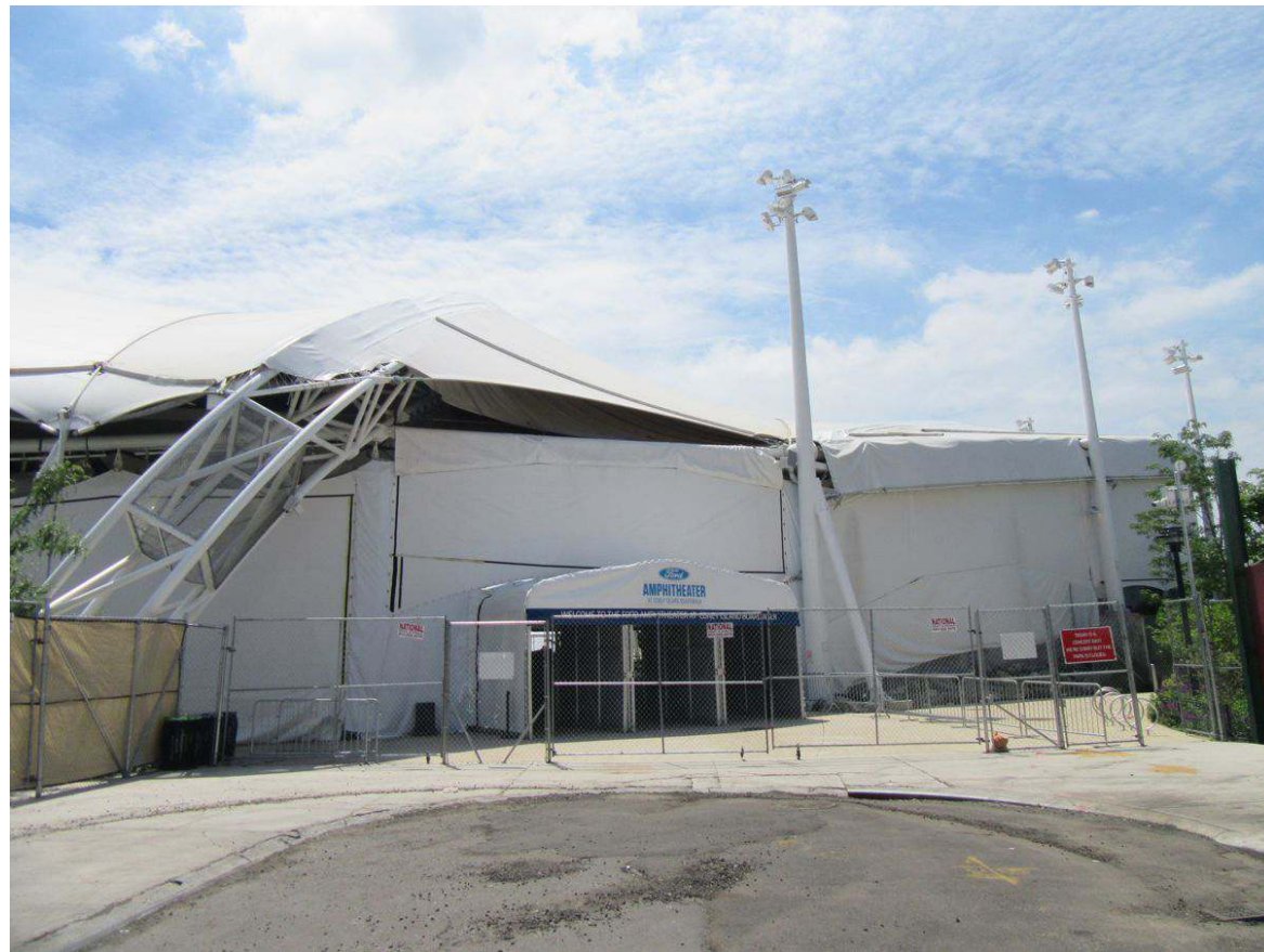
3. View of the amphitheater facing south on West 22nd Street.
