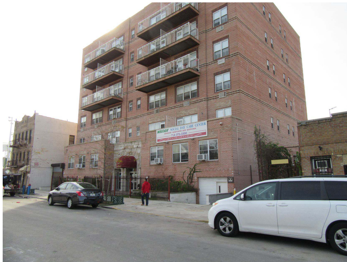
6. View of the side of West 22nd Street facing southwest.
