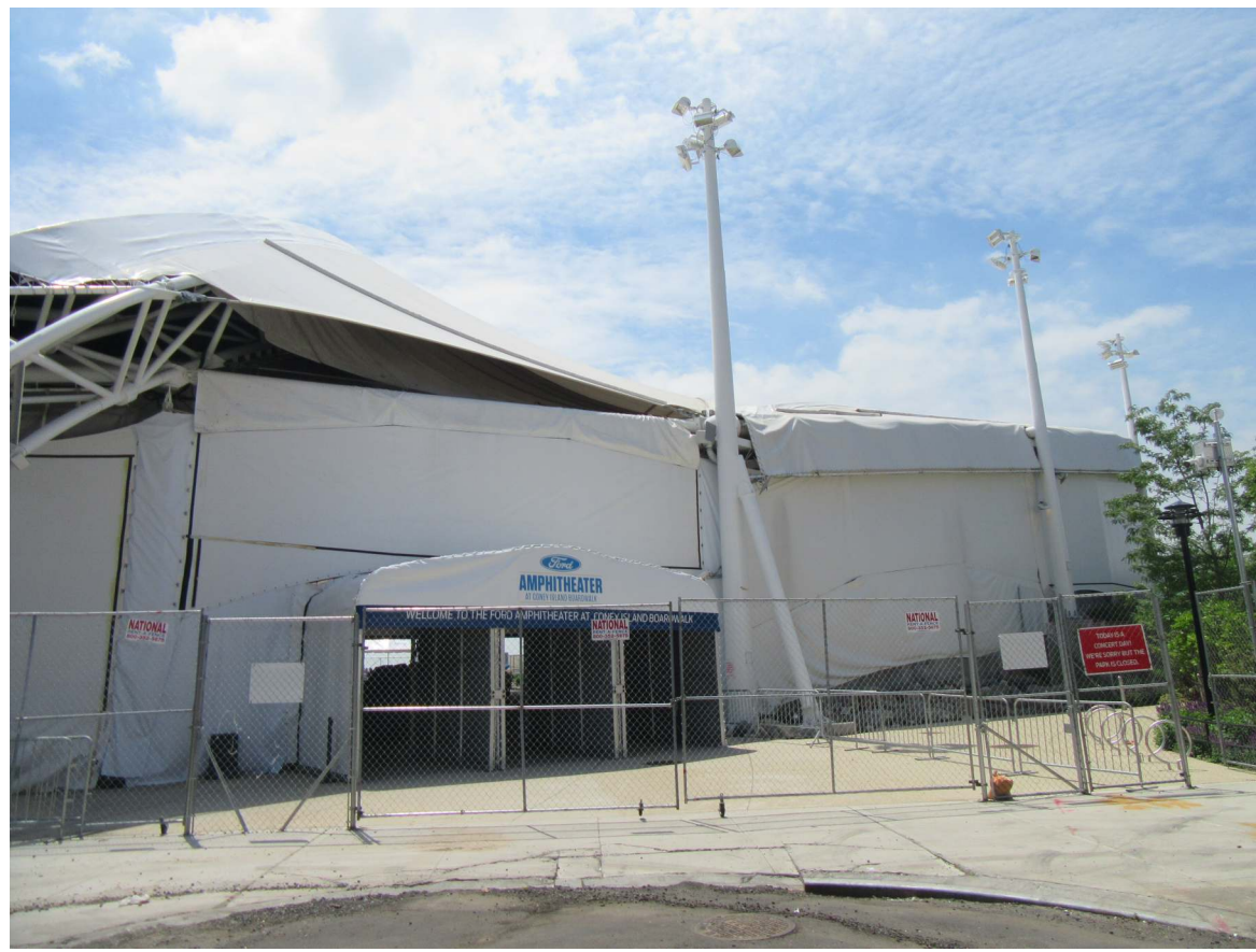
1. View of West 22nd Street facing south.
