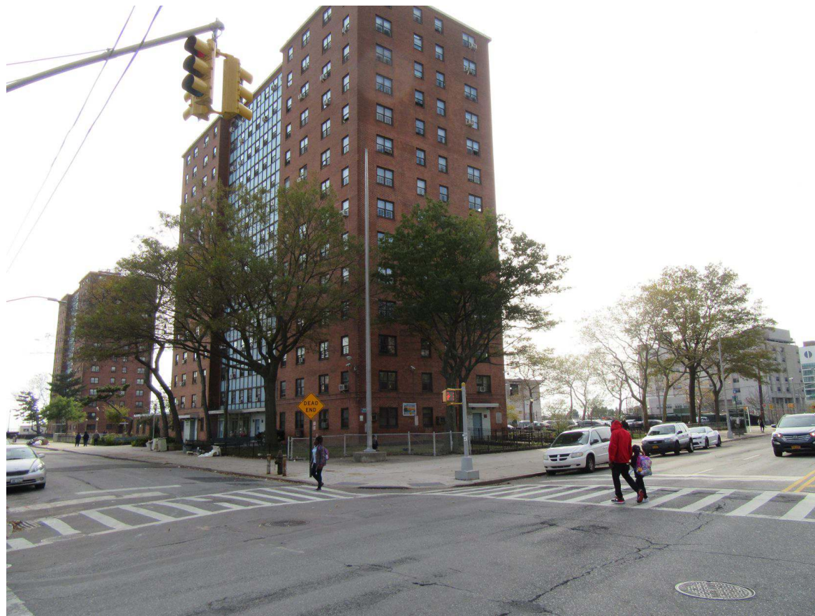
36. View of the side of Surf Avenue facing southwest from West 24th Street.
