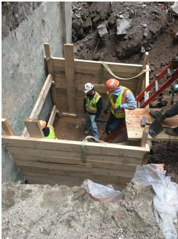
Photo 5: TP-3 - Excavation progress. Facing Southwest
