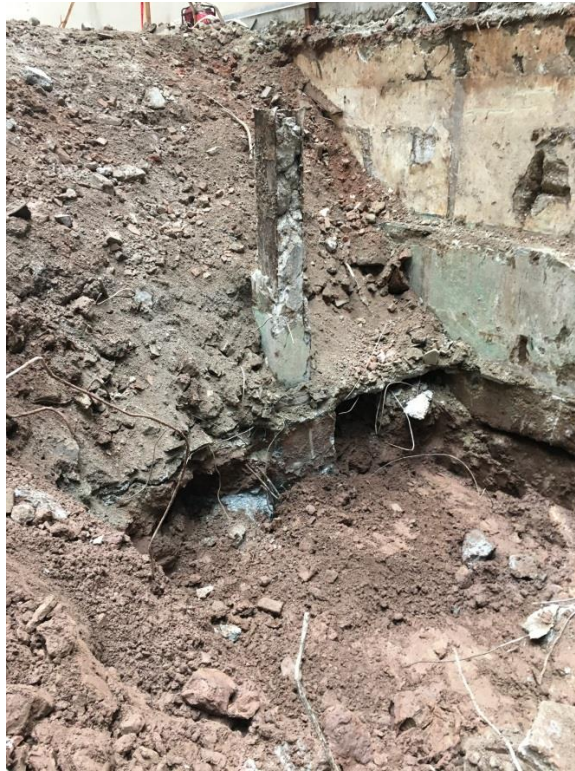
Photo 1: TP-1 - General view of the excavation. Facing Northwest.
