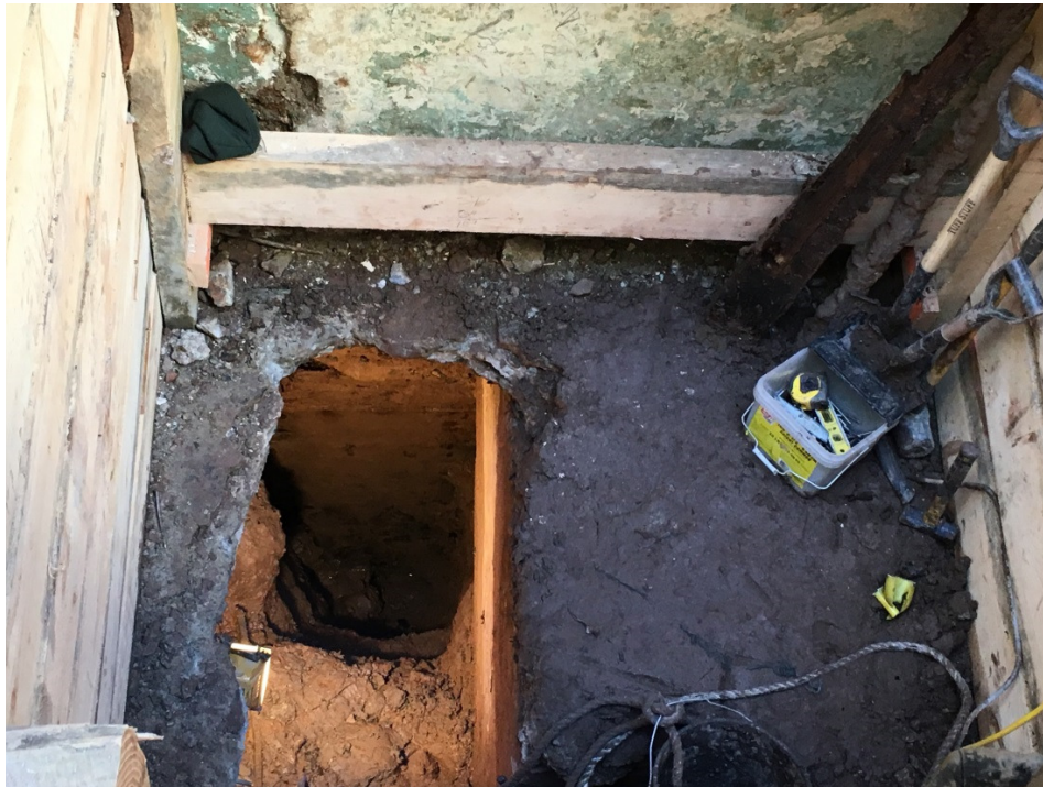
Photo 006: General view of the test pit showing the foundation wall extending to 23 feet below the ground surface, facing south.
