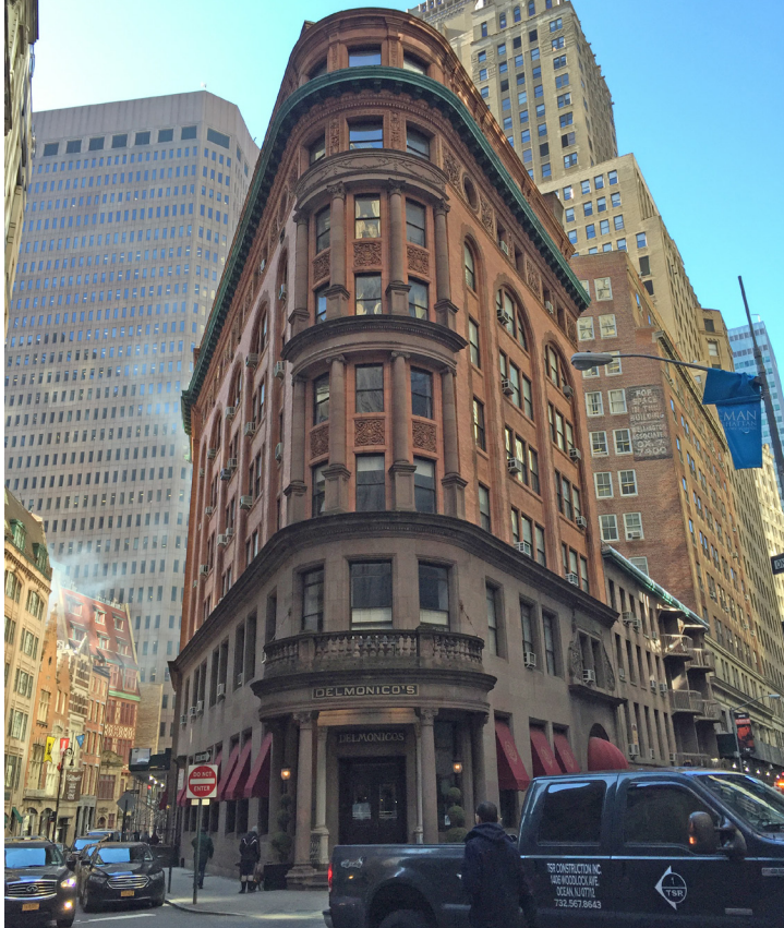
Photograph 25: Delmonico's Restaurant - historic building at 48 Beaver Street (southwest corner of Braver and William streets)
