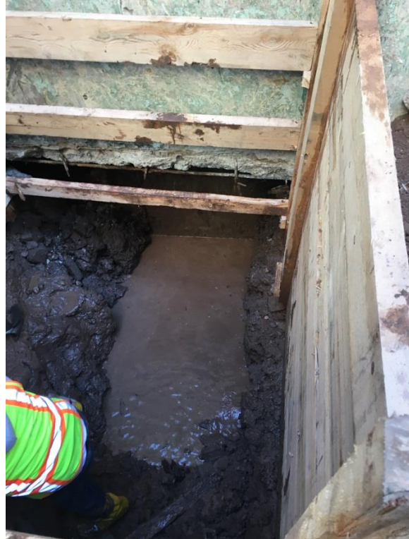
Photo 6: TP-3 - End of Excavation. Looking from above
