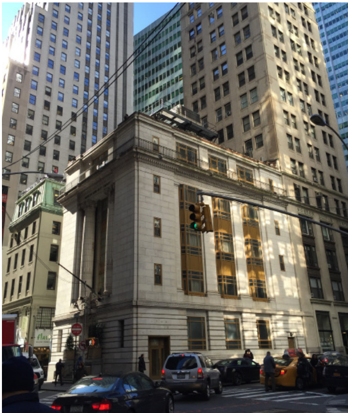
Photograph 20: American Bank Note Building - historic building at 70 Broad Street (southwest corner of Broad and Beaver streets)
