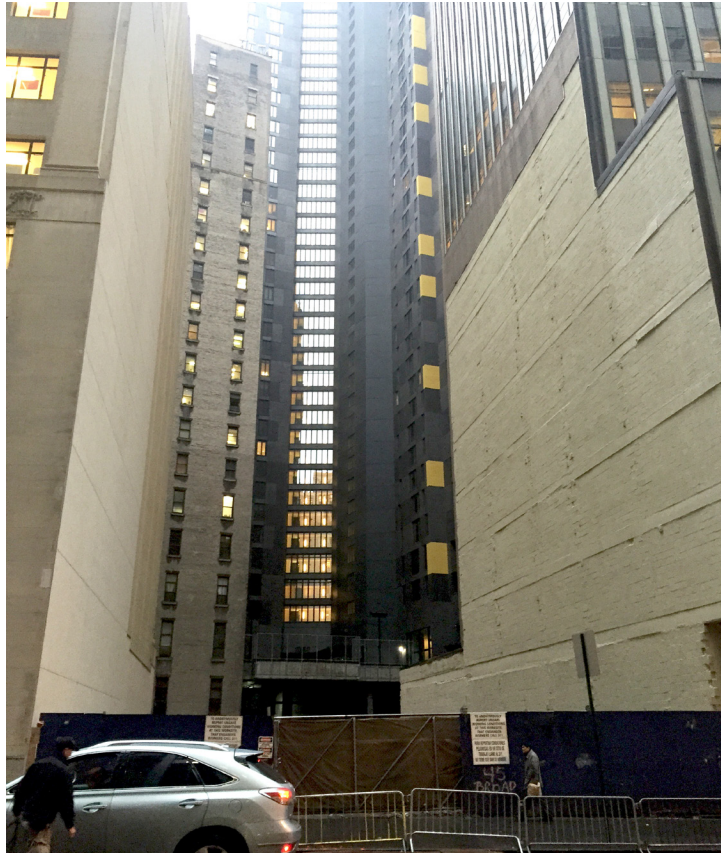
Photograph 1: Directly across the Project Site on Broad Street
