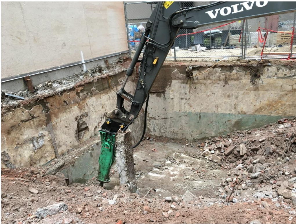
Photo 3: TP-2 - General view of the excavation. Facing Northeast.
