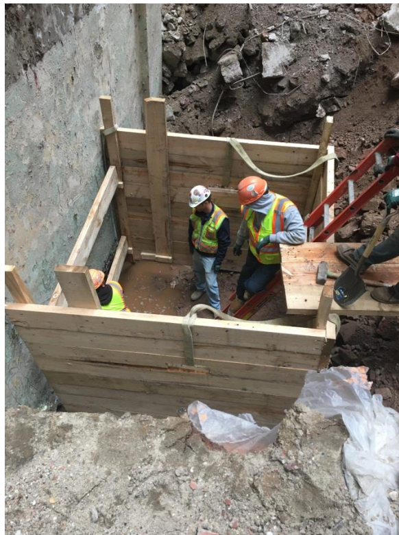
Photo 5: TP-3 - Excavation progress. Facing Southwest
