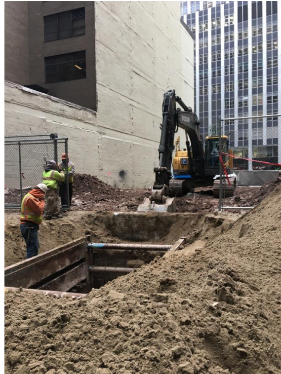
Photo 9: TP-4 - Excavation complete. Facing West
