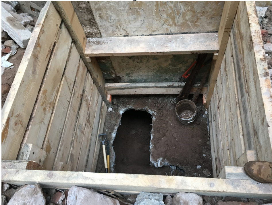
Photo 005: General view of the test pit showing the pile cap encountered, facing south.
