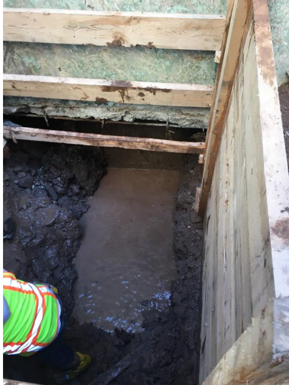
Photo 6: TP-3 - End of Excavation. Looking from above
