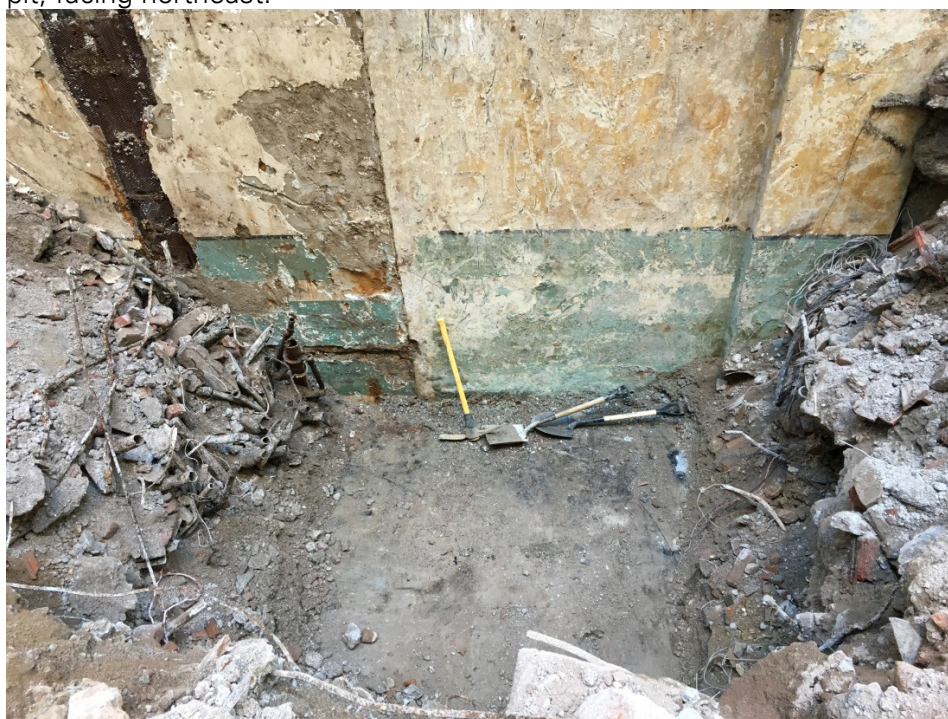
Photo 003: General view of the basement slab encountered at 12 feet below the ground surface, facing south.
