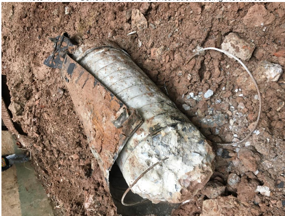
Photo 2: TP-1 - Concrete Raymond pile from former building foundations
