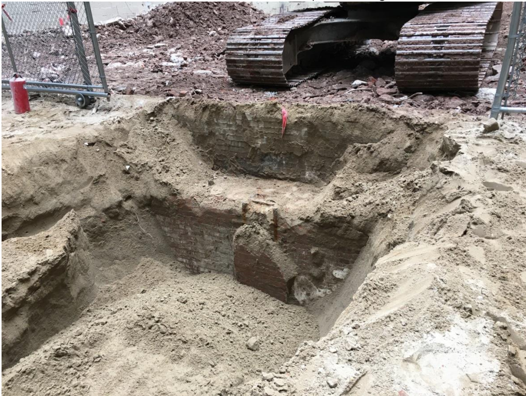
Photo 8: TP-4 - Excavation progress. Facing West
