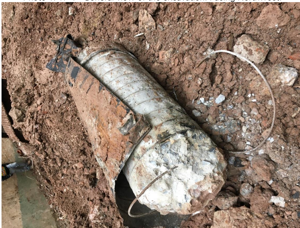
Photo 2: TP-1 - Concrete Raymond pile from former building foundations
