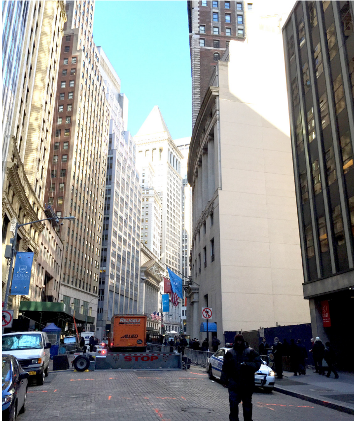
Photograph 3: At Beaver Street, looking north on Broad Street; the Existing 9-story school building and Development Site to the right.
