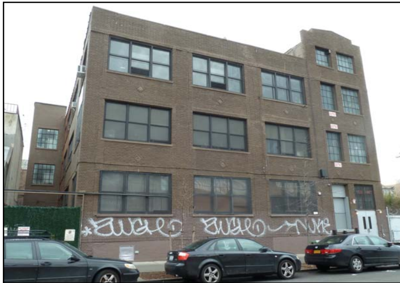
6. View of residential building located on Tax Lot 27 looking southeast from Hart Street.
