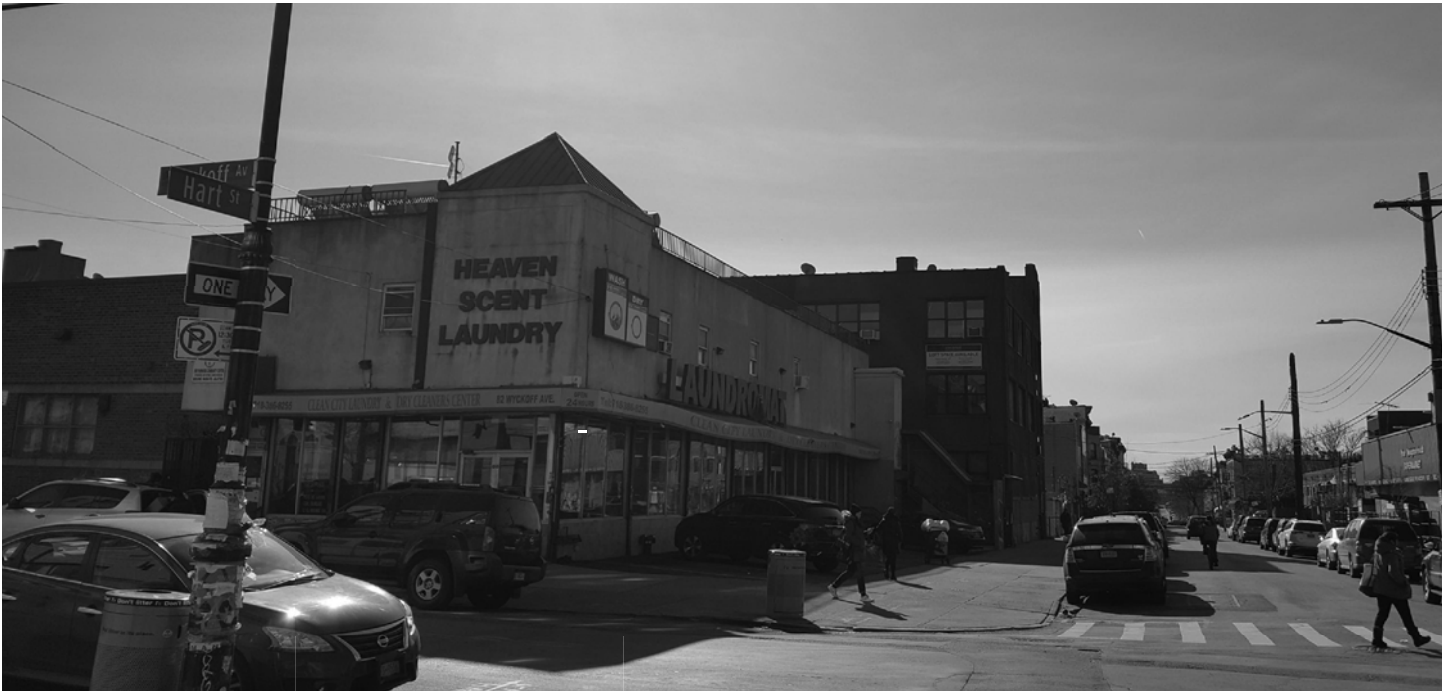
No-Action view of Lot 31 site looking southwest long Wyckoff Avenue
