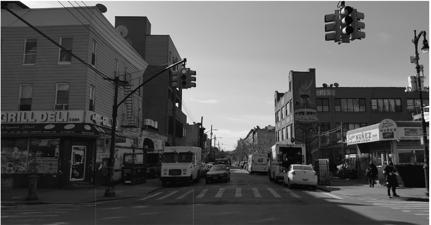
No-Action view of the project site looking southwest long Dekalb Avenue
