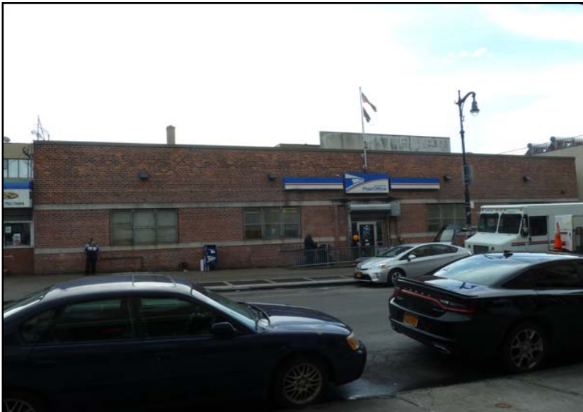
6. View of USPS post office located on Tax Lot 33 looking southwest from Wyckoff Avenue.
