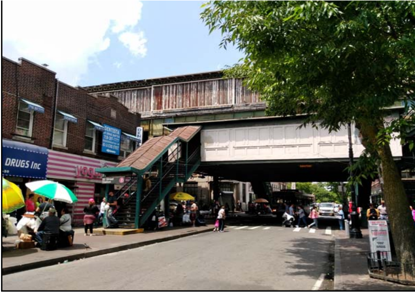
13. View of 82nd Street elevated Subway Station entrance (No. 7 Train) looking northwest along 82nd Street.
