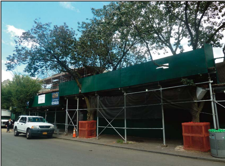
7. View from 82nd Street looking northeast towards proposed development site.
