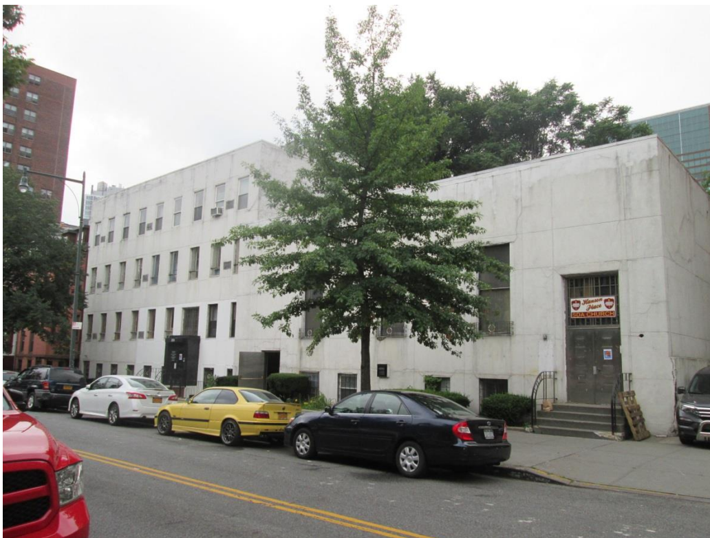
Photo 2: View of Projected Development Site 1, looking southwest on South Portland Avenue.
