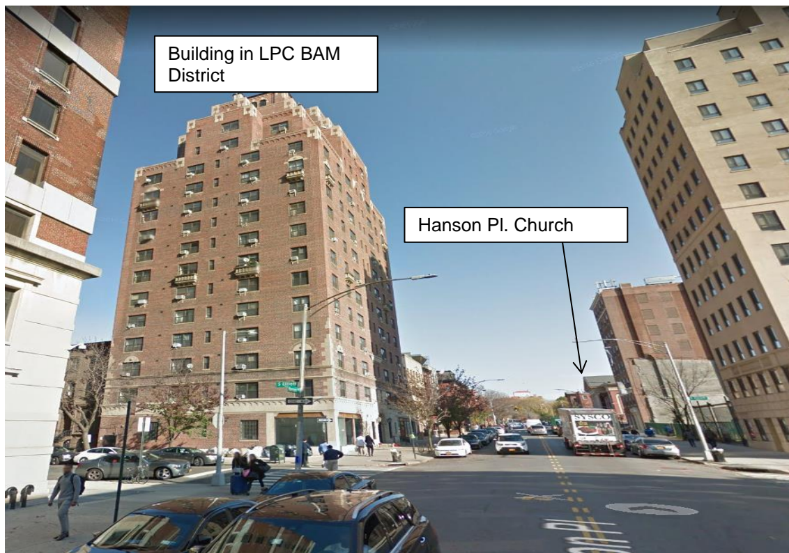
View of building located within BAM Historic District, looking east on Hanson Place from South Elliot Place
