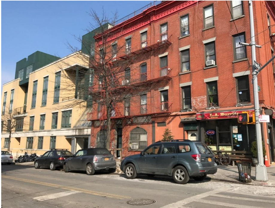
Photo 3: View of adjacent lots (1 & 3) included in rezoning from the corner of Underhill Ave. and Dean St. looking northeast.
