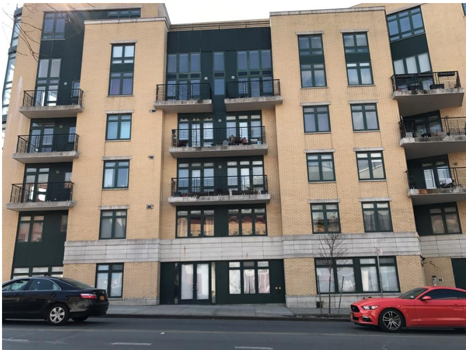
Photo 2: View of Applicant Site from Washington Avenue
