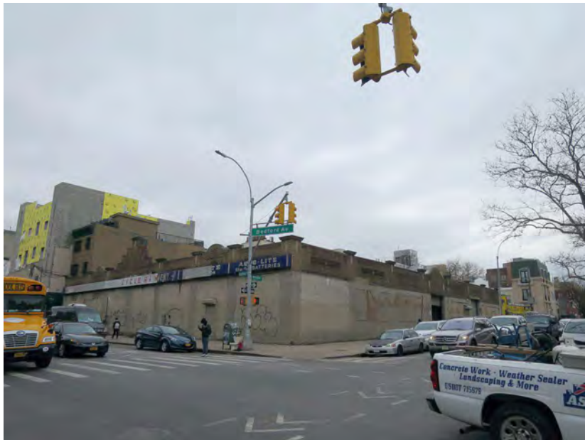
9. View of the intersection of Willoughby Avenue and Bedford Avenue facing southwest from the Site.
