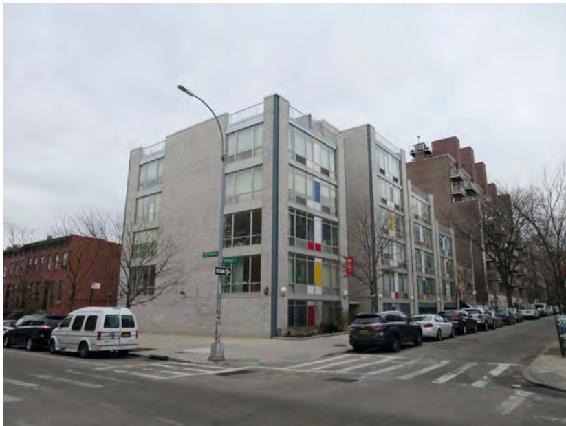
18. View of the intersection of Willoughby Avenue and Spencer Street facing southeast.
