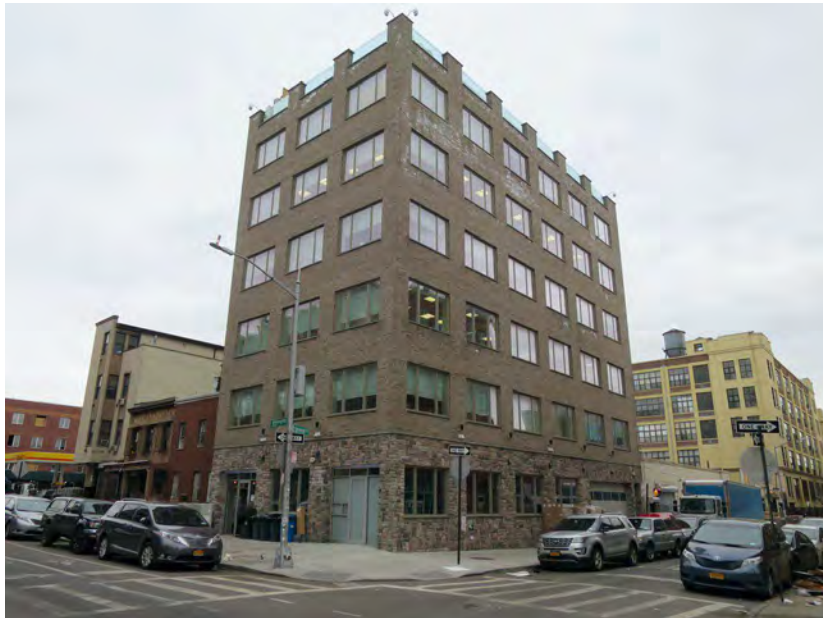
15. View of the intersection of Willoughby Avenue and Spencer Street facing northwest.
