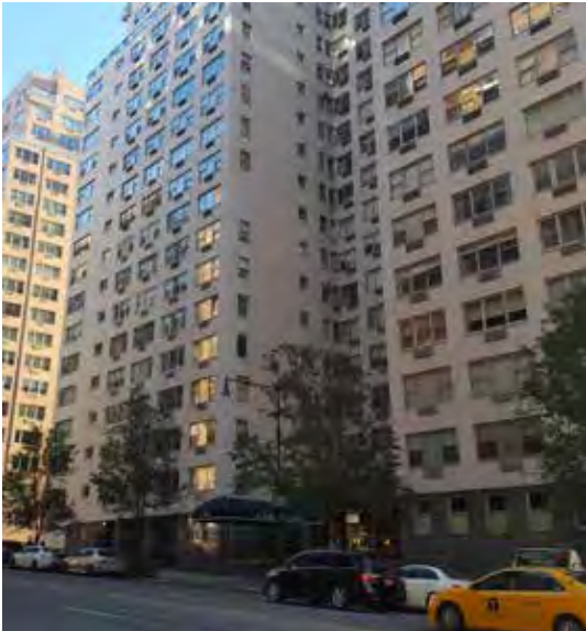
Photo 2.4-7 Cannon Point South (45 Sutton Place) has a recessed front courtyard
