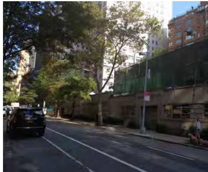
Photo 17 View looking northwest along East 55th Street
