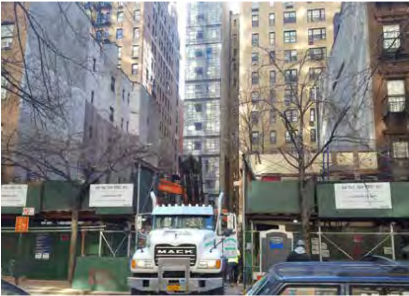
Photo 13 View of ongoing demolition at projected site 1a (photo captured February 6, 2017)
