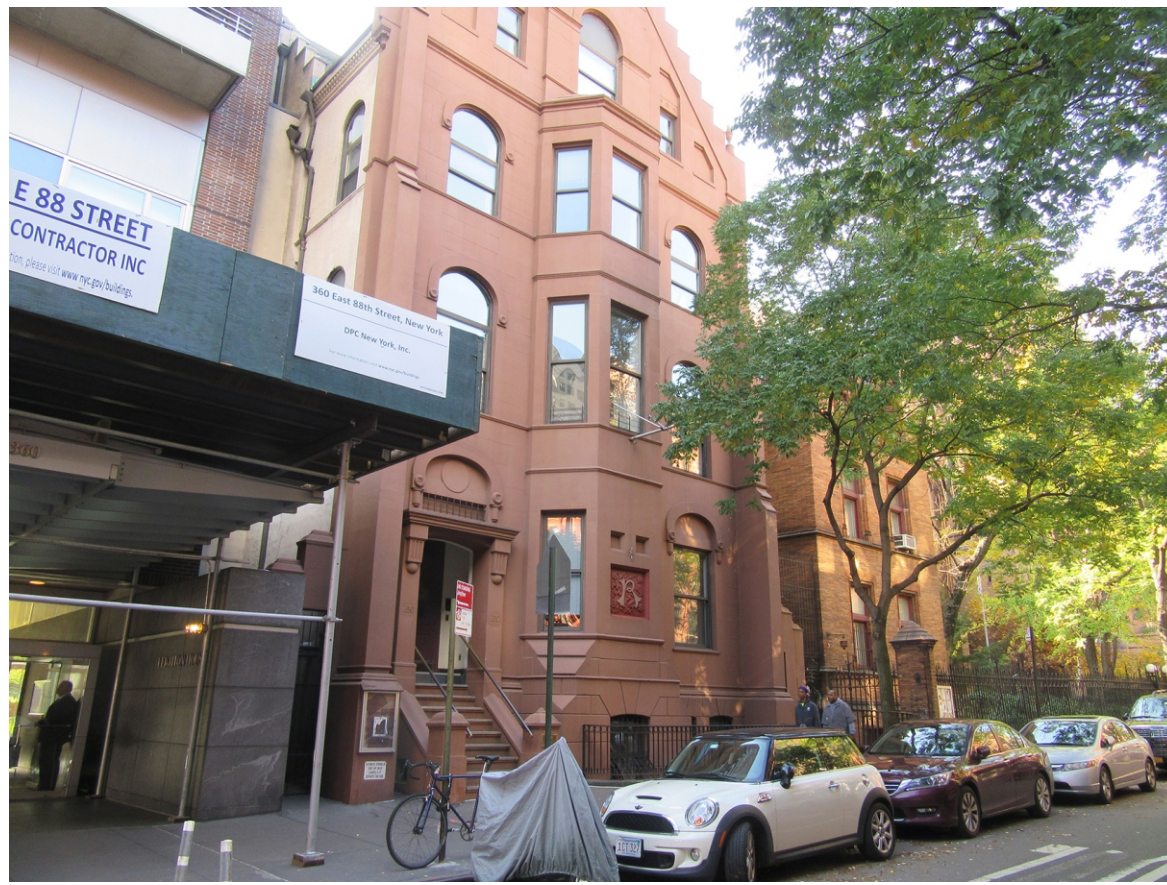
1. View of the Site facing southwest from East 88th Street.
