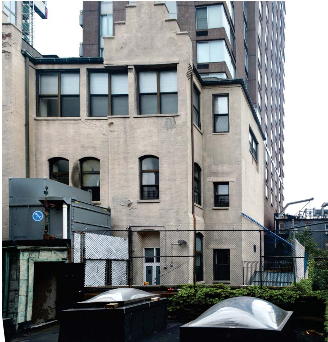
EXISTING VIEW FROM CHURCH ROOF TO TERRACE
