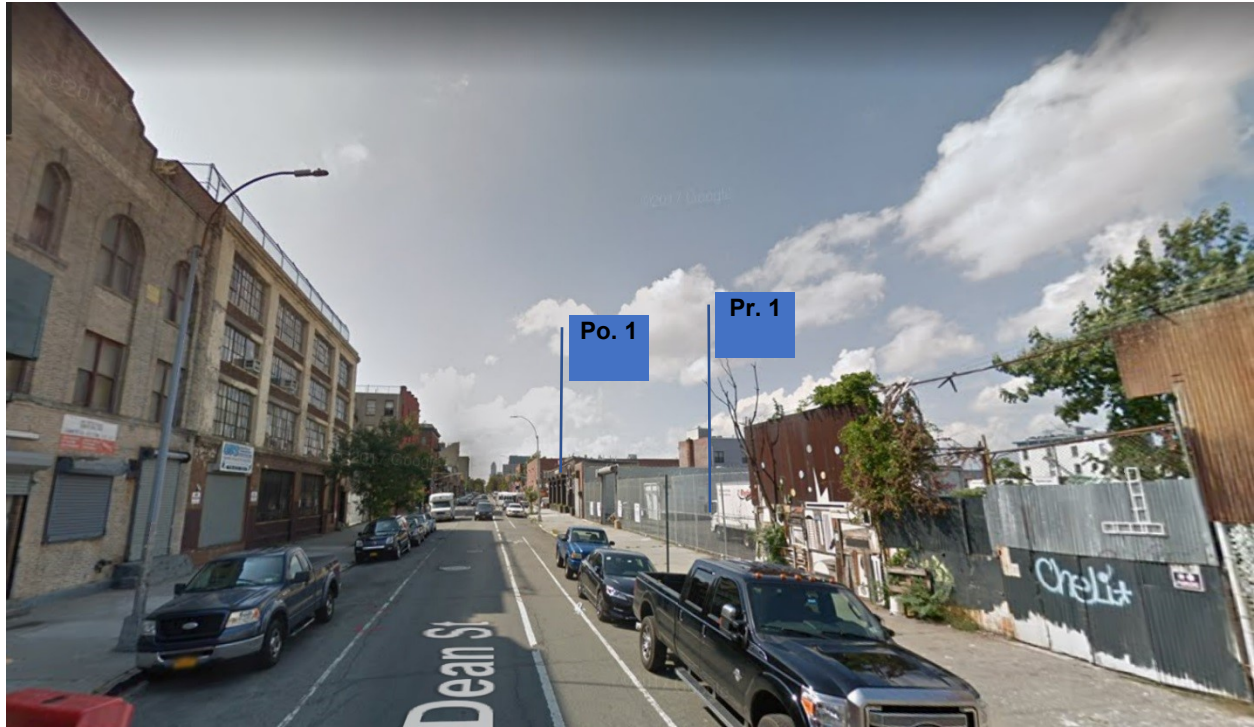
Figure 2.6-2: Existing Condition 1– Looking West on Dean Street
