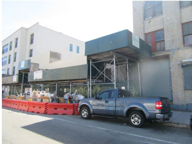
4. View of the south side of Dean Street facing southeast from the Site.
