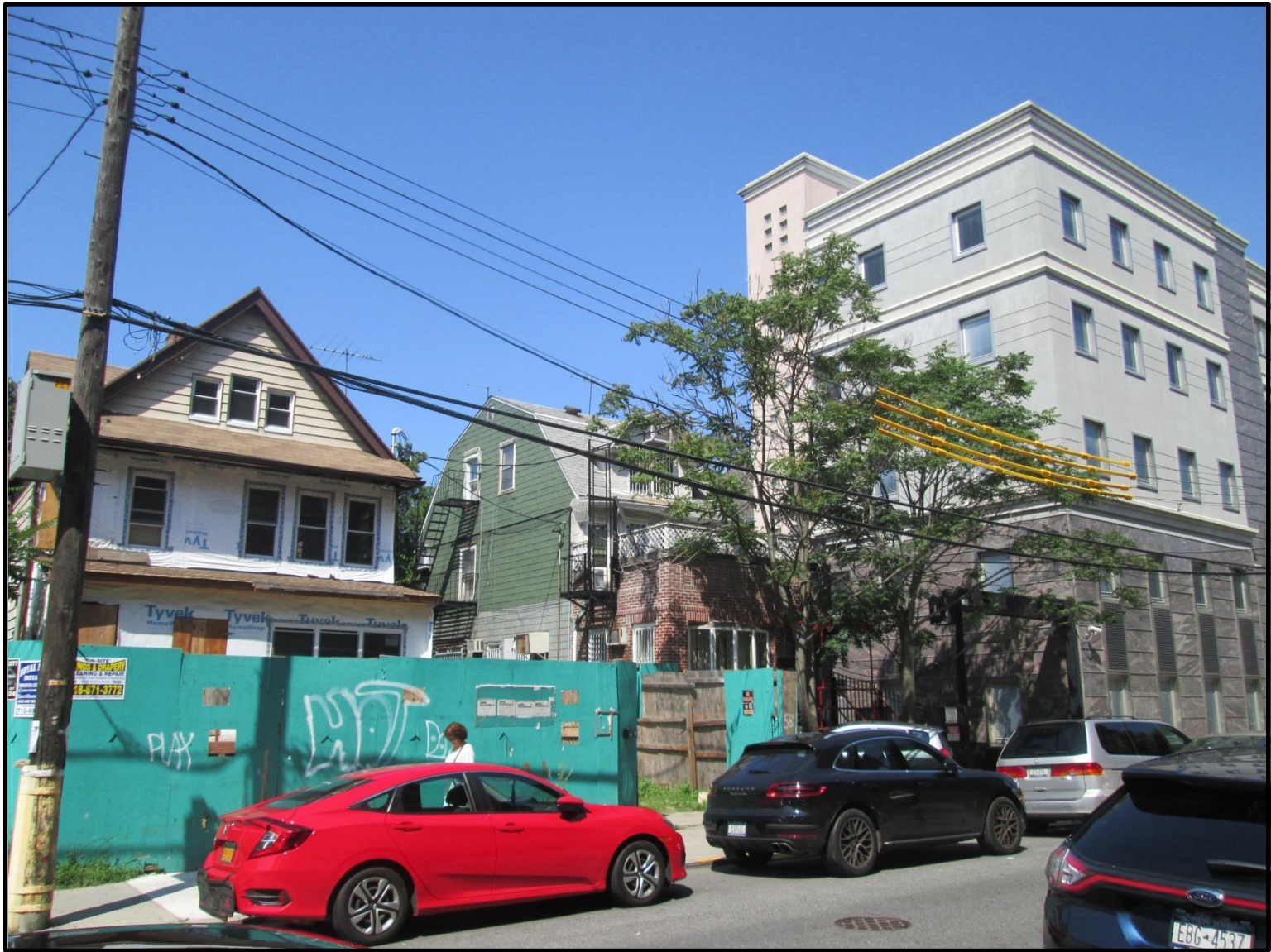
View of Projected Development Site 1 from East 13 th Street, facing west.
