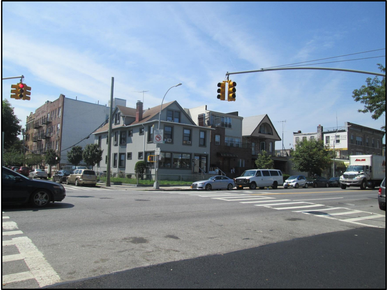
View of Projected Development Site 2 from Avenue P, facing south.
