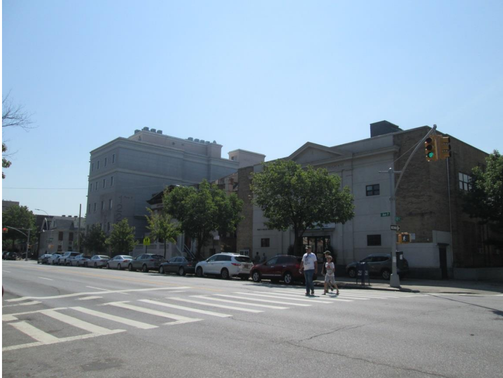
Photo 5: View of Projected Development Site 1 and neighboring community facility buildings on Avenue P from the northeast corner of East 12 th Street and Avenue P, facing southeast.
