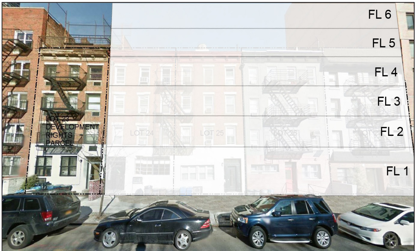
With-Action view of the project site looking north along East 33rd Street
