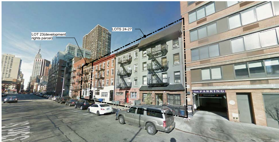
3. View of development site looking north west
