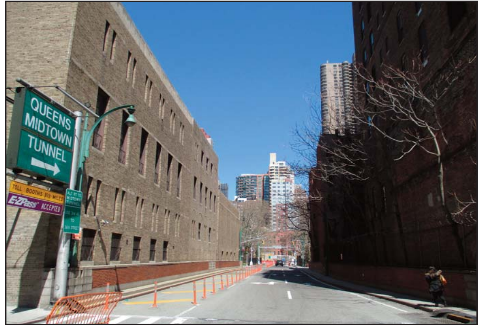
10. View of Queens Midtown Tunnel Entrance looking north from East 34th Street
