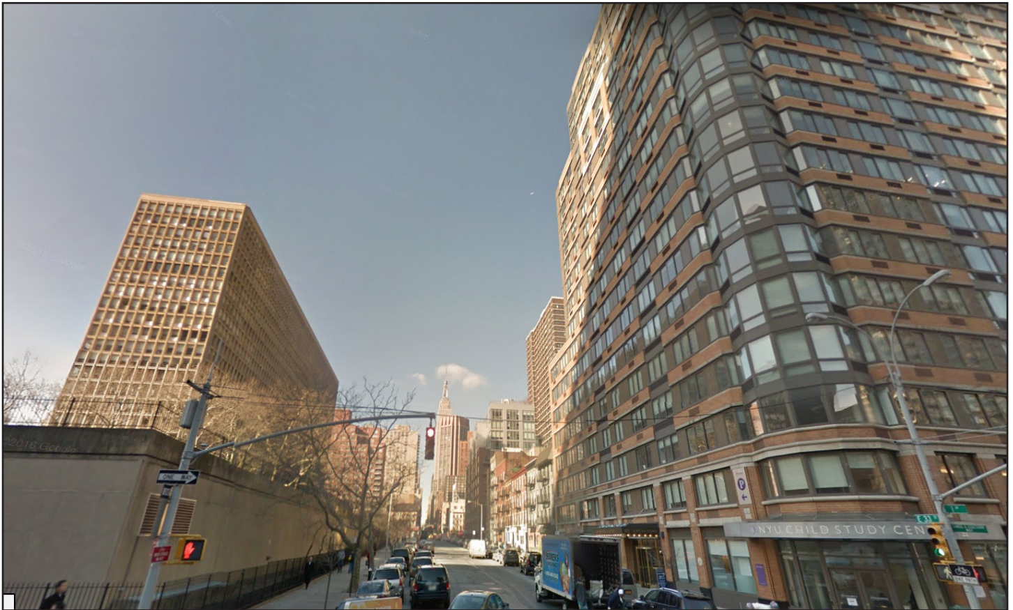
No-Action view of the project site looking west along East 33rd Street
