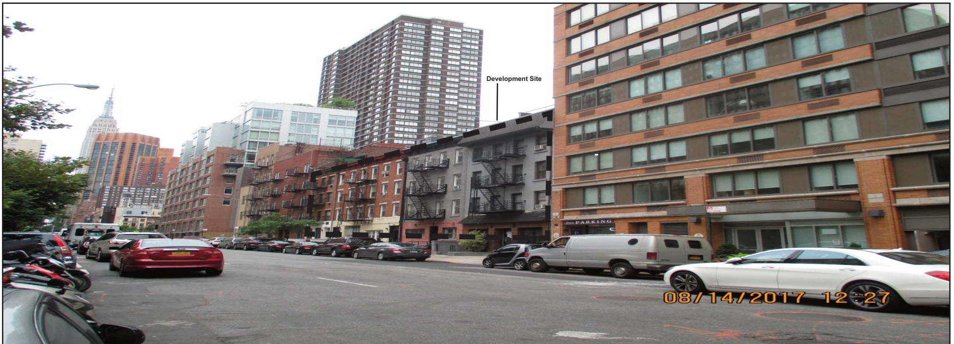
26. View of development site looking northwest
