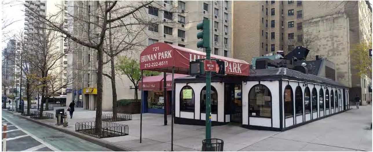
Figure UD-5: Existing One-Story Building at Southwest Corner of Subject Site
