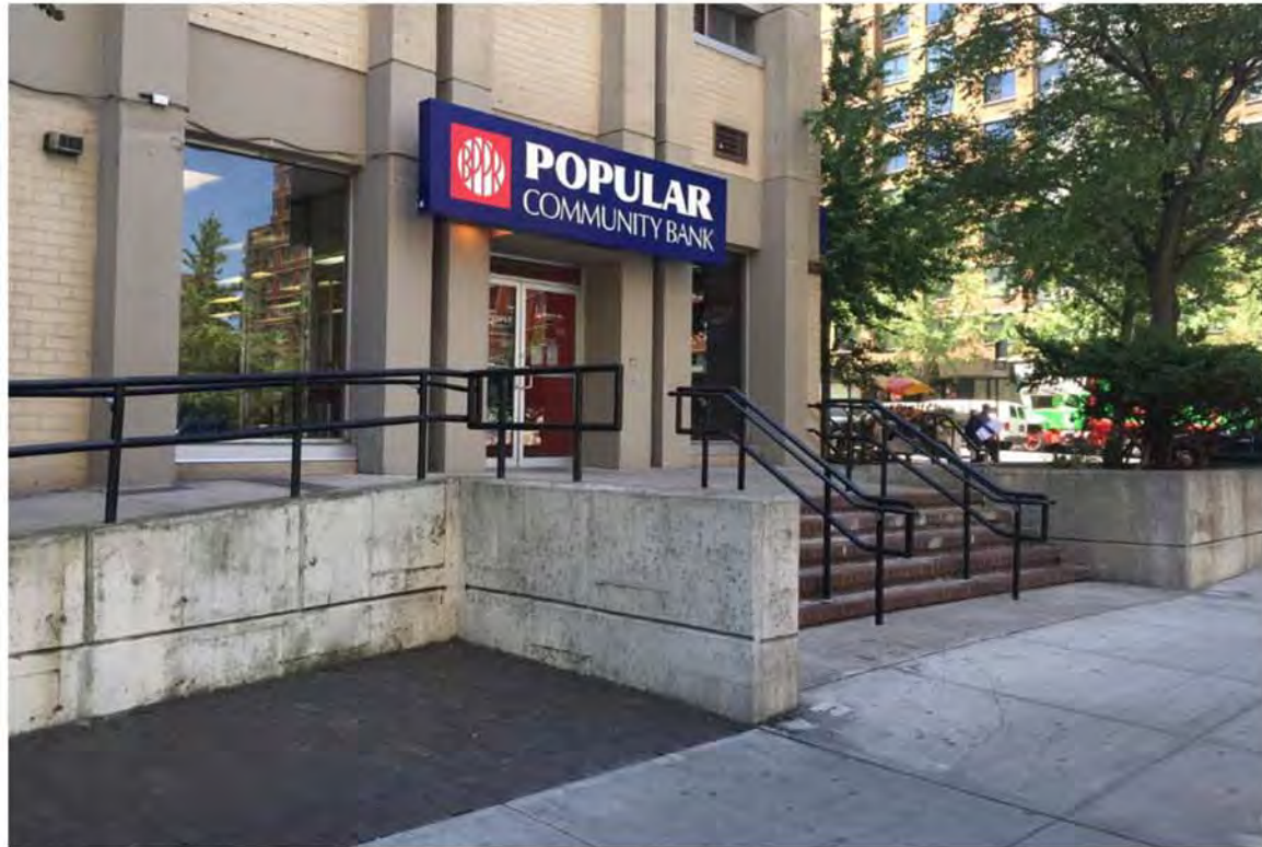
03 96TH ST ELEVATION LOOKING SOUTH
