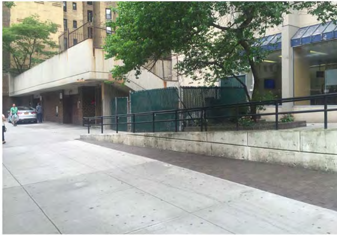
01 96TH ST ELEVATION LOOKING SOUTH
