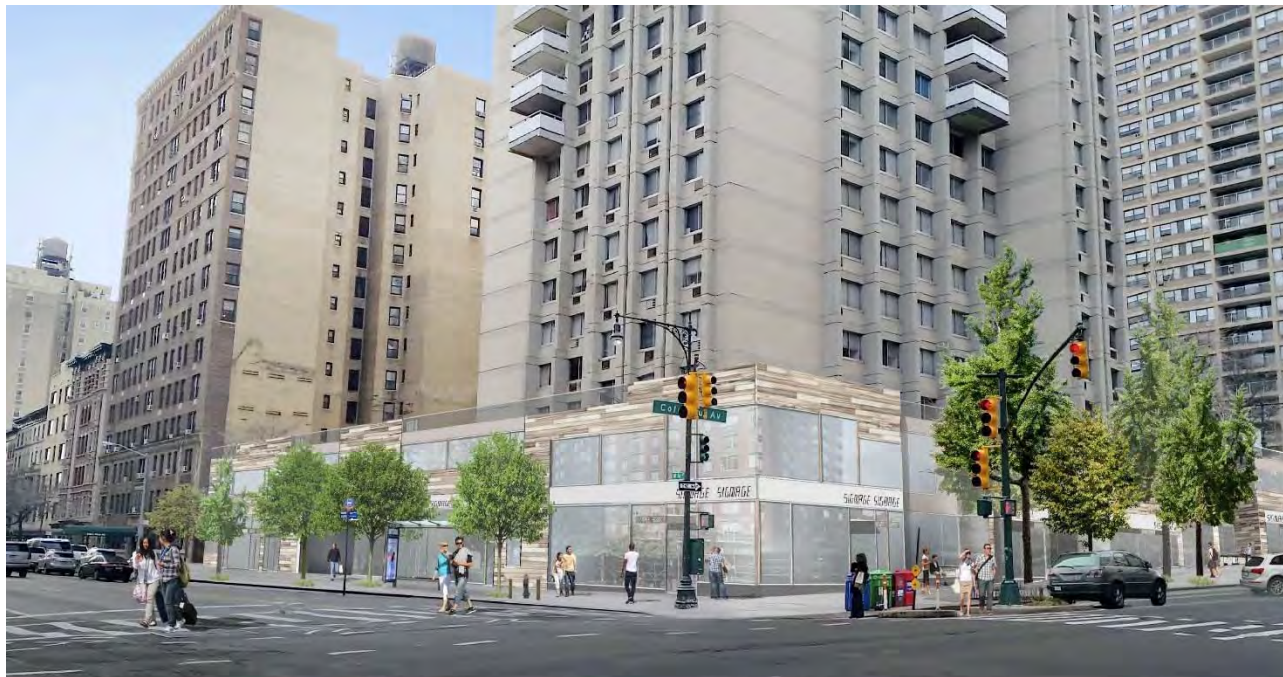
Figure UD-4: Proposed Development from Southwest Corner of Columbus Avenue and West 95 th Street
