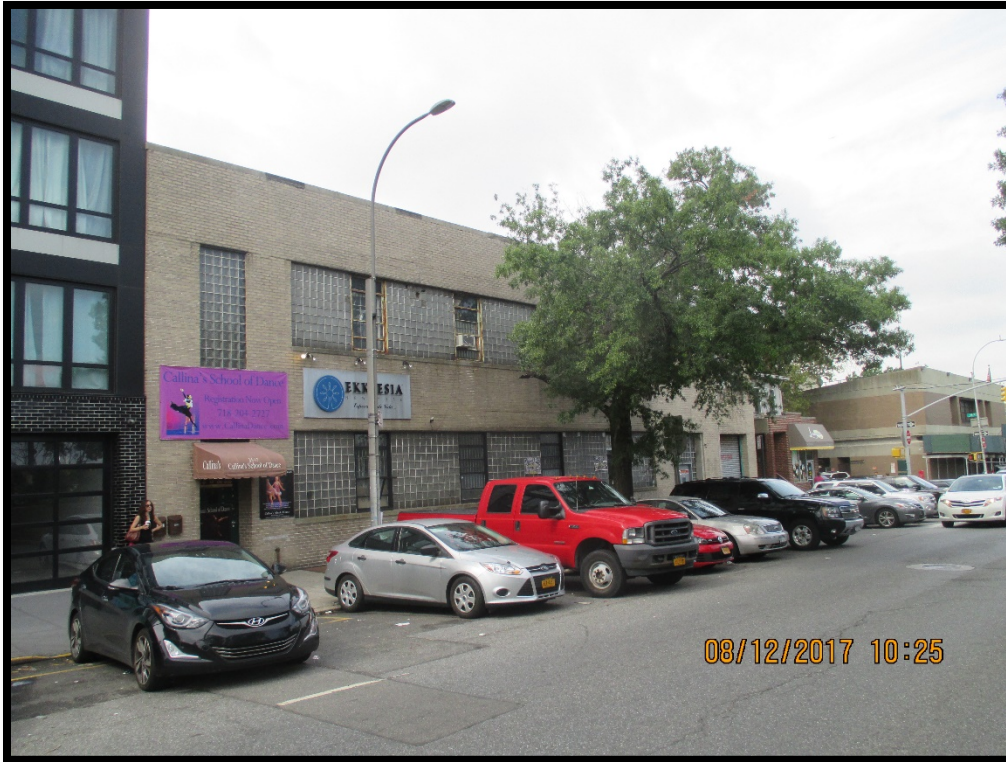
Photo 3 View of Projected Development Site 1, facing southwest from Astoria Blvd. South.
