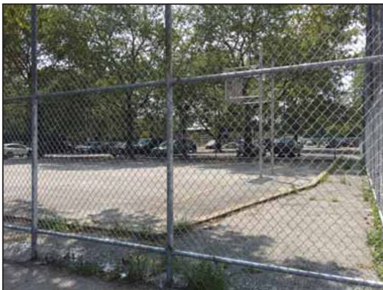
View south from the corner of Turnbull Avenue and White Plains Road of the existing basketball court.
