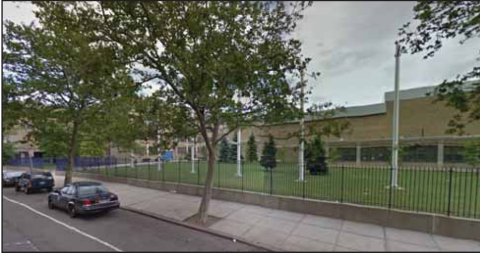
Public school on south side of Lafayette Avenue (view southeast)
