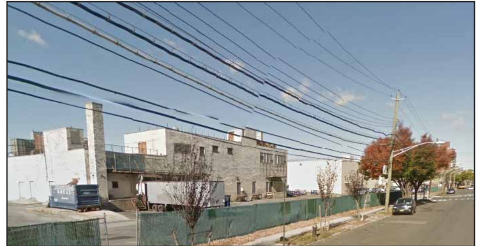
Shops at Bruckner Bruckner Boulevard loading on west side of Pugsley Avenue (view northwest)
