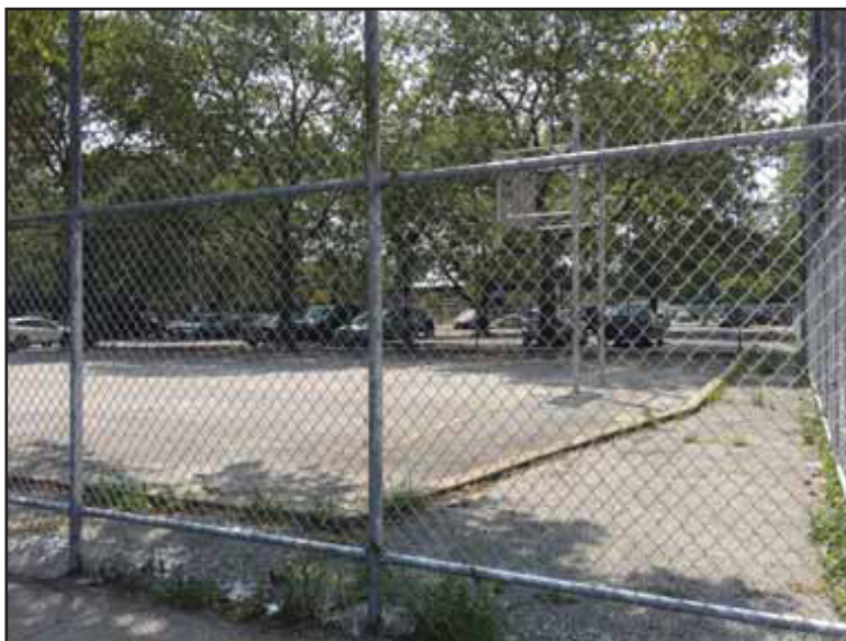
3. View south from the corner of Turnbull Avenue and White Plains Road of the existing basketball court.
