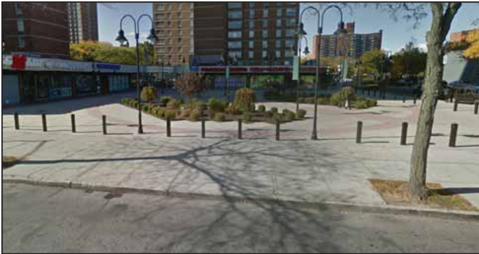
Plaza at southwest corner of White Plains Road and Lafayette Avenue (view west)
