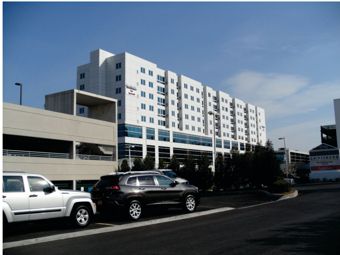
3. View of the Site facing southeast from Bassett Avenue.
