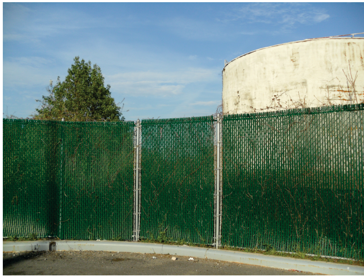
31. View of the side of Marconi Street facing northeast from the Site.
