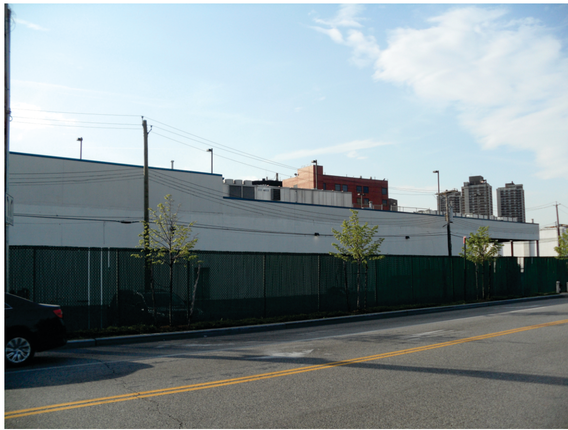
19. View of the west side of Marconi Street facing northwest.
