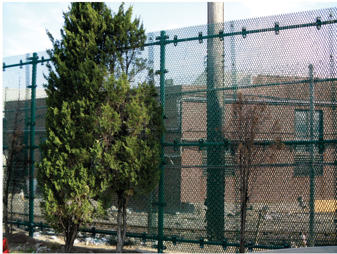
16. View of the side of Waters Place facing southeast, between Eastchester Road and Marconi Street.
