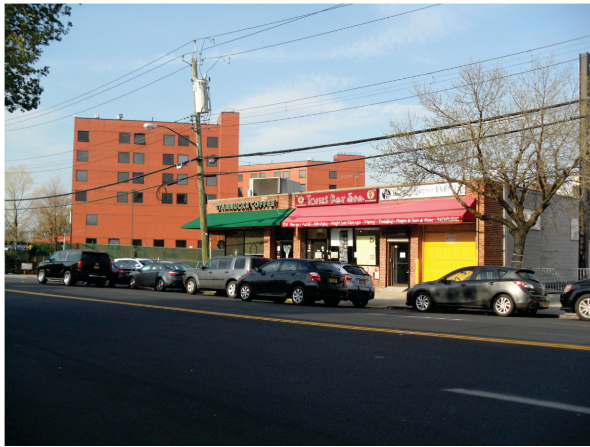
13. View of the side of Eastchester Road facing northeast between Bassett Avenue and Waters Place.
