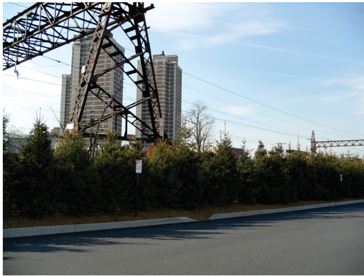
4. View of the side of Bassett Avenue facing northwest from the Site.
