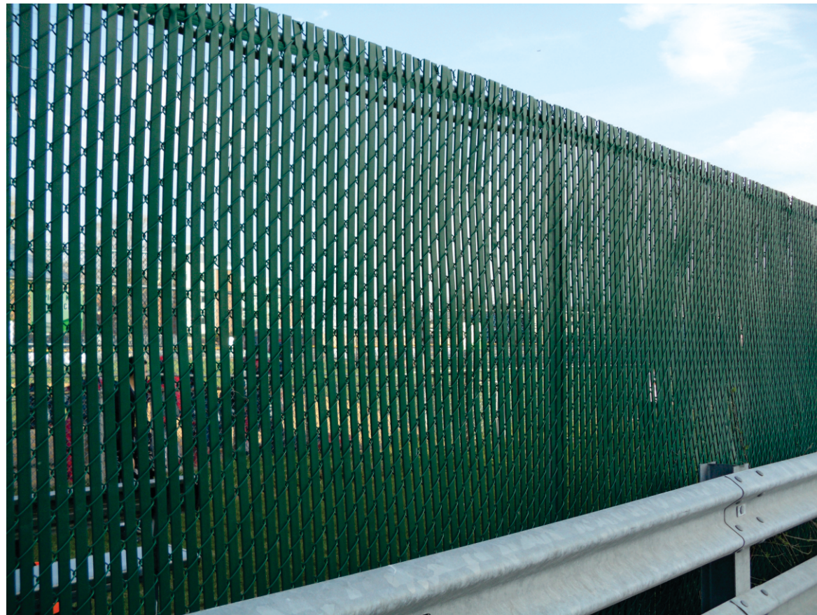
27. View of the side of Marconi Street facing southeast from the Site.
