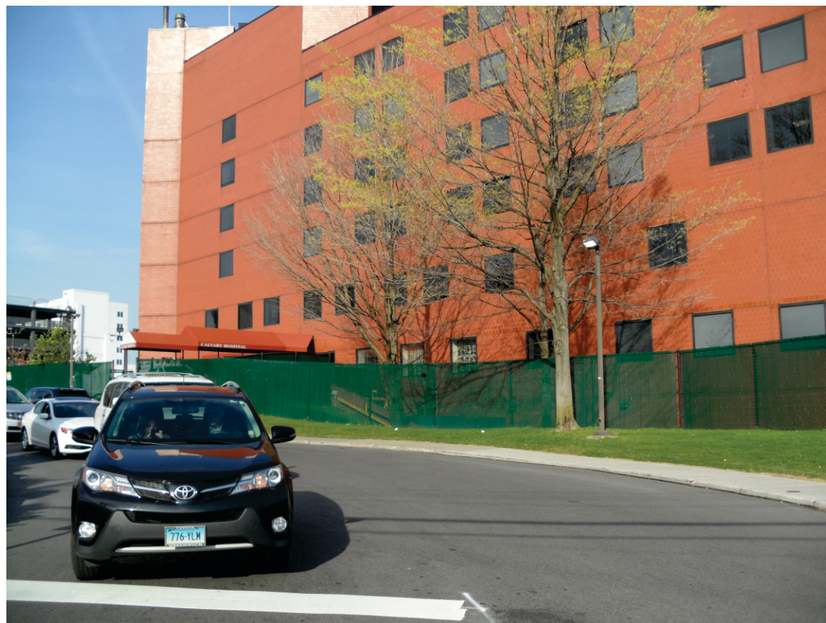
9. View of Bassett Avenue facing northeast (Site ahead at center).
