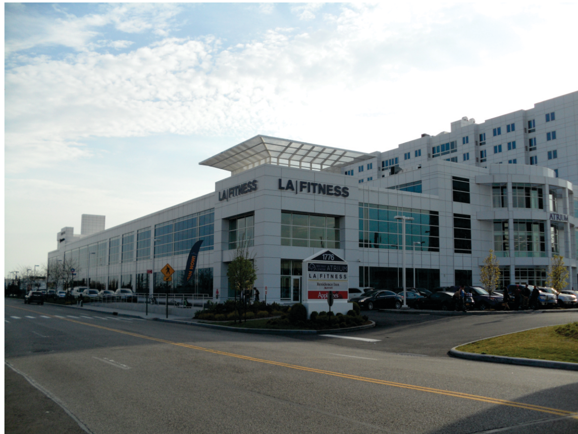
30. View of the Site facing southwest from Marconi Street.
