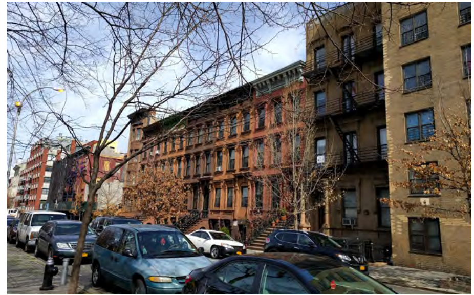
Photo 10 View of low-rise residential rowhouses looking north on East 124th Street
