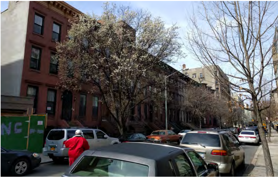
Photo 13 View of low-rise rowhouses looking west on East 127th Street
