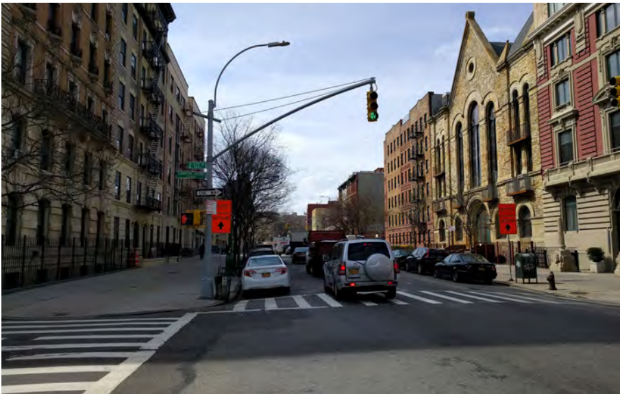
Photo 7 View of mid-rise multifamily residential buildings looking south on Fifth Avenue
