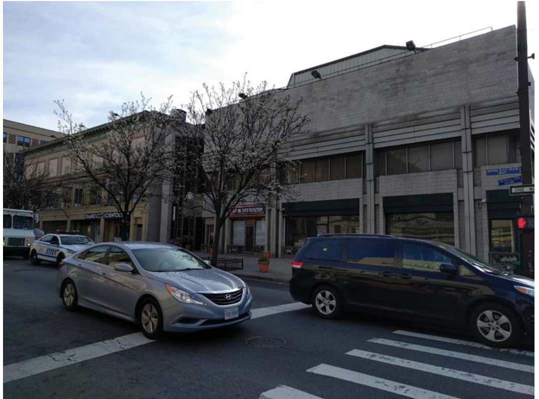
View of Existing Building Fifth Avenue frontage
