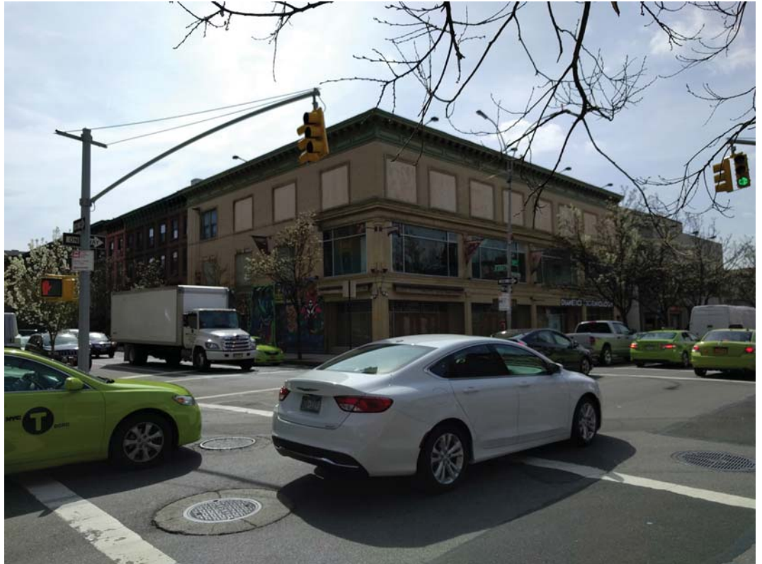
View of Existing Building looking southeast on 126th Street
