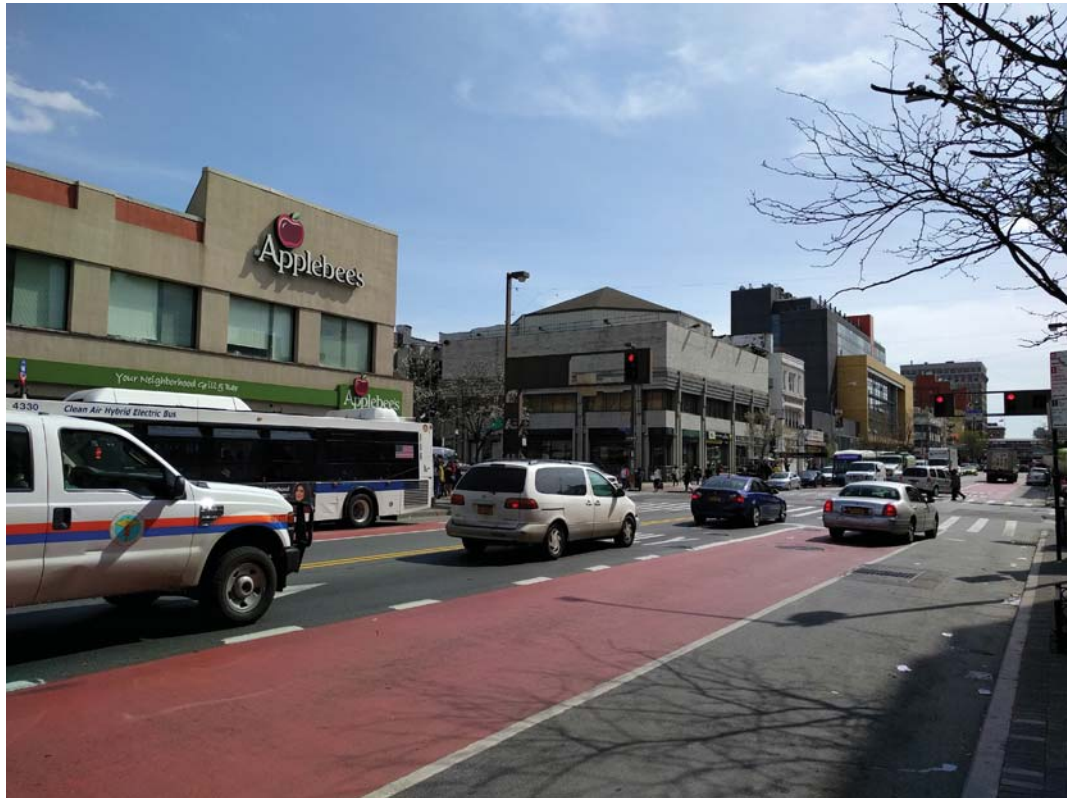
View of Existing Building looking east on 125th Street
