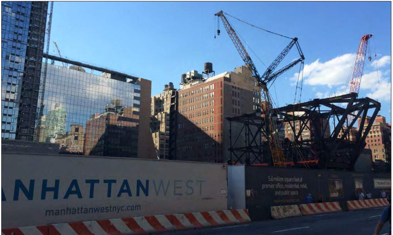
View looking northwest from West 31st Street and Ninth Avenue 1
