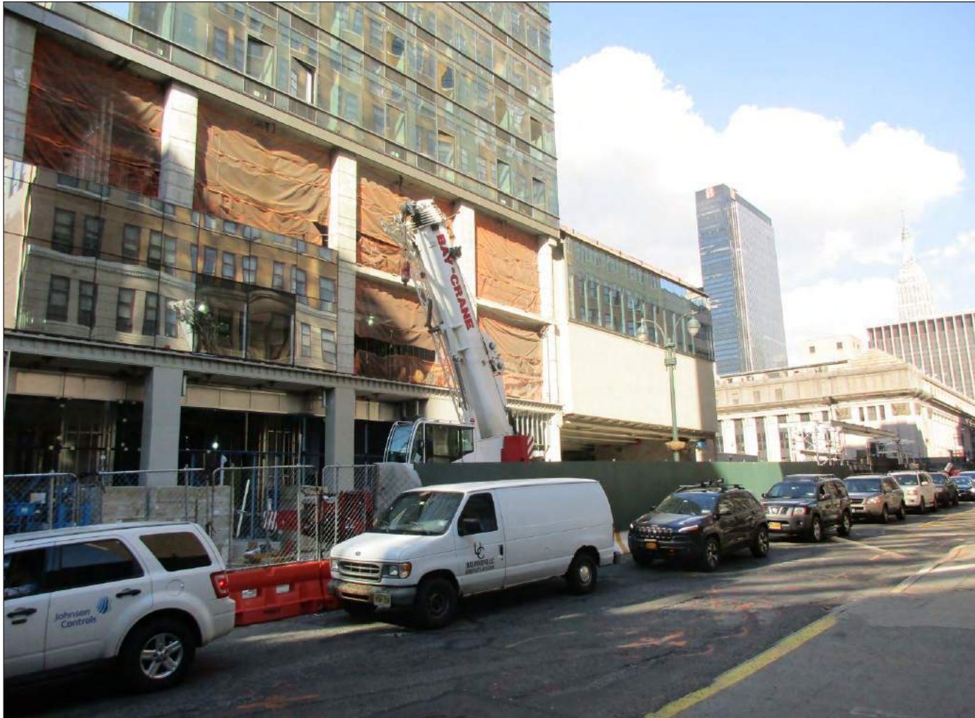
View looking northeast from West 31st Street and Dyer Avenue 5
