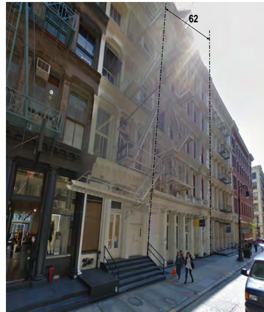
VIEW 3 GREENE STREET LOOKING SOUTH
