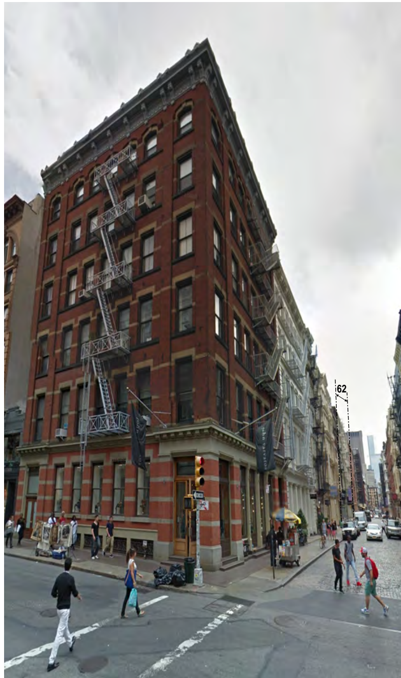
VIEW 1 GREENE STREET LOOKING SOUTH
