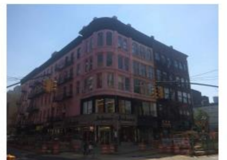
VIEW H: PRIOR TO CERTIFICATE OF NO EFFECT WORK
