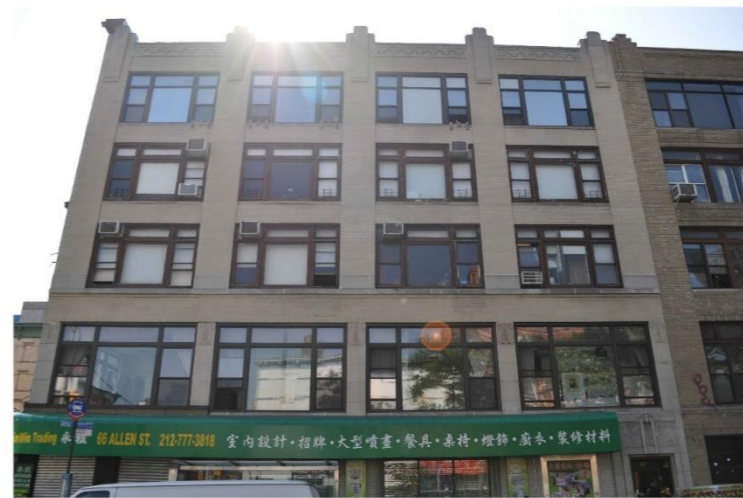
ALLEN ST FACADE PRIOR TO CERTIFICATE OF NO EFFECT WORK
