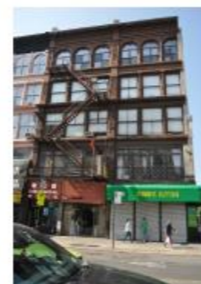
VIEW I: PRIOR TO CERTIFICATE OF NO EFFECT WORK
