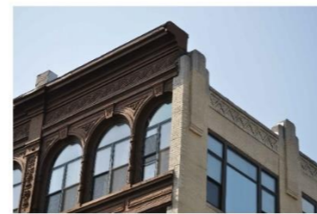
CORNER PRIOR TO CERTIFICATE OF NO EFFECT WORK
