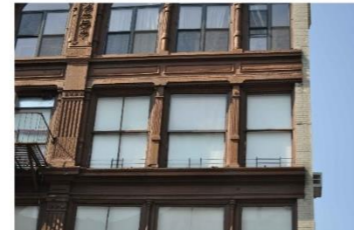
GRAND ST 4TH FLOOR PRIOR TO CERTIFICATE OF NO EFFECT WORK
