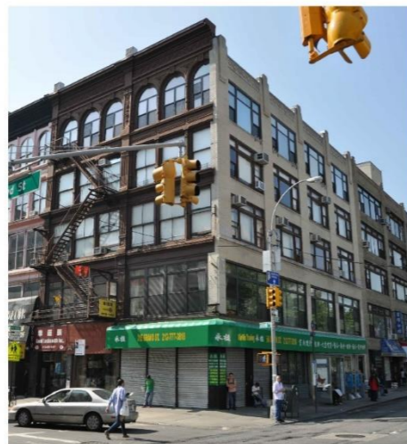
VIEW FROM ALLEN ST PRIOR TO CERTIFICATE OF NO EFFECT WORK
