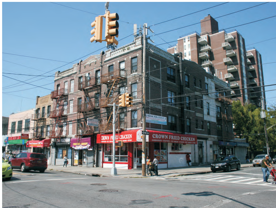
12. View of the intersection of Mermaid Avenue and West 28th Street facing northwest.
