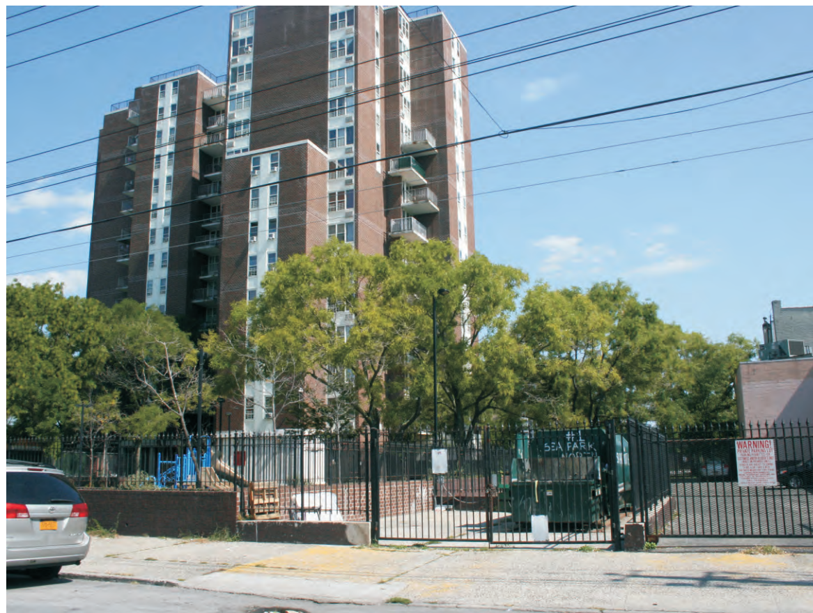
3. View of the side of West 29th Street facing northeast.
