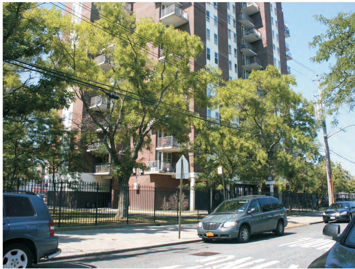
16. View of the side of West 28th Street facing northwest.
