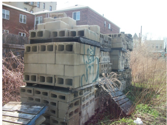
Concrete blocks typical of debris inside the Property
