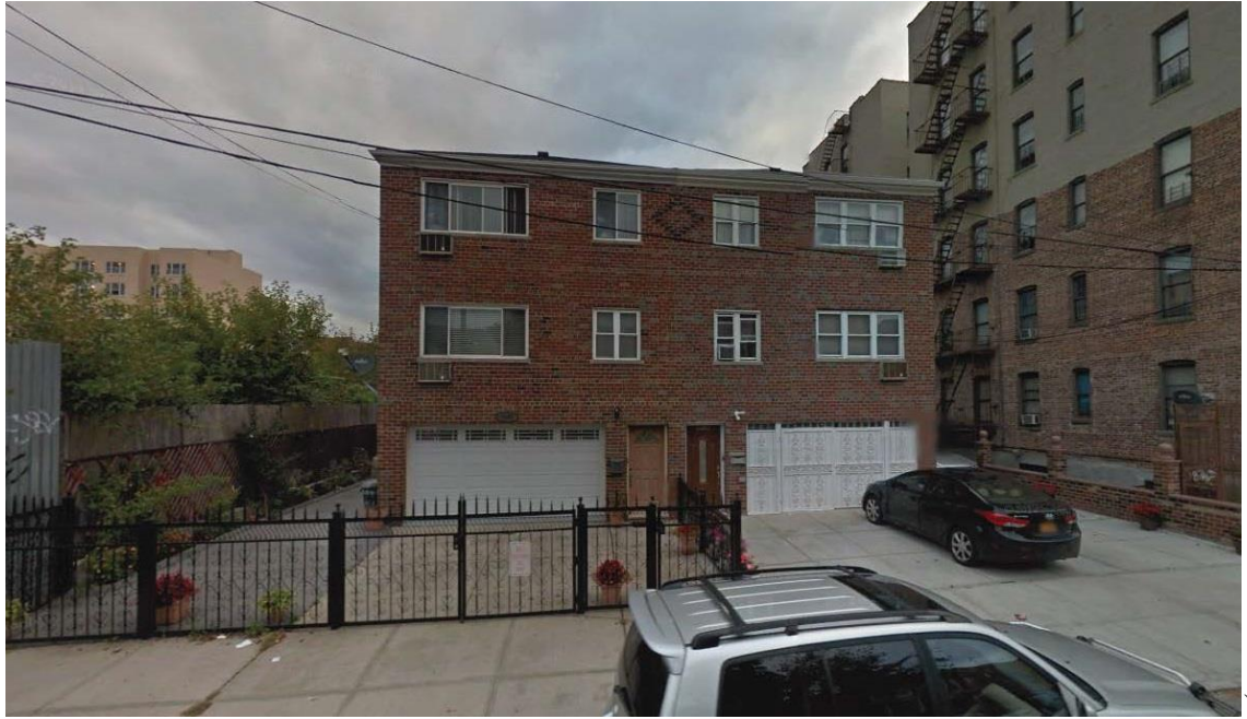
Figure 2.7-5: Existing Conditions – Projected Development Site 2 (Lots 55 & 56)
