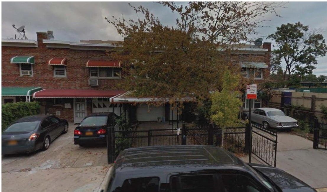
Figure 2.7-6: Existing Conditions – Projected Development Site 3 (Lots 69,71 and 72)
