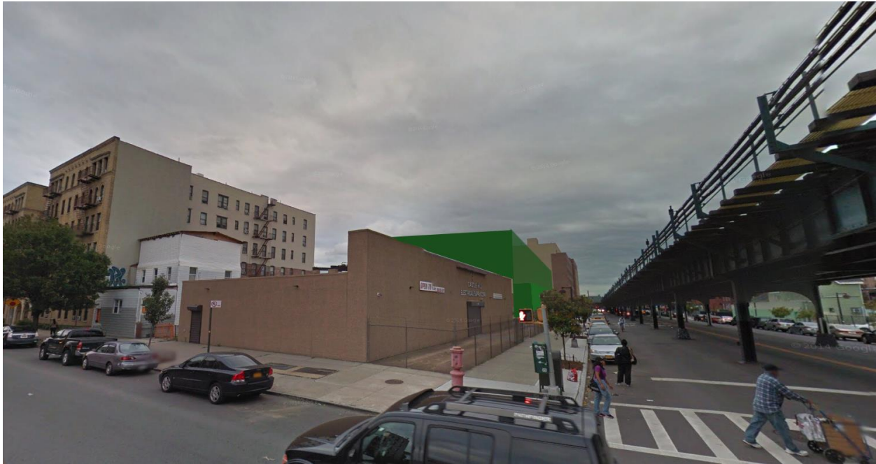
Figure 2.7-11: No-Build - Westchester and Olmstead Intersection Looking West
