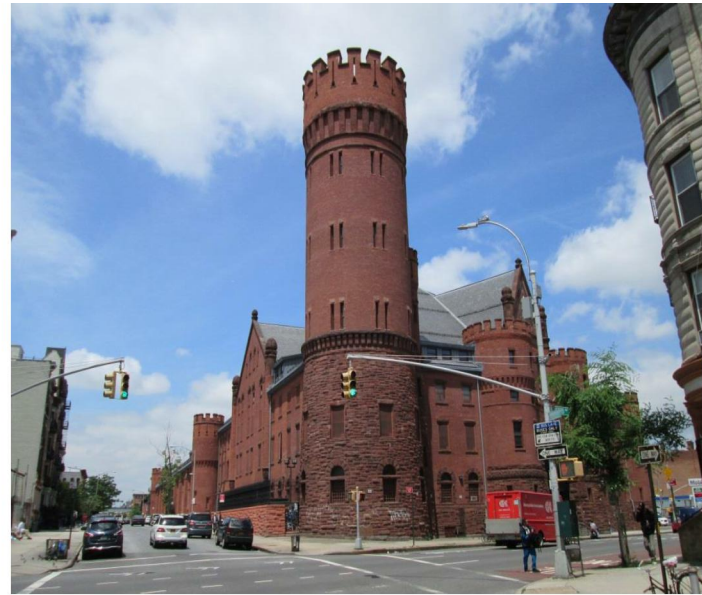
View of 23 rd Regiment Armory at 1322 Bedford Avenue (Across Pacific Street from Project Site)
