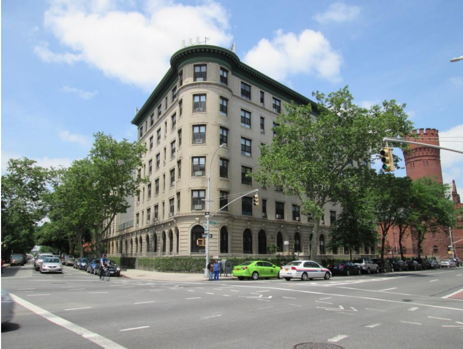
View of adjoining six-story residential building located at 1350 Bedford Avenue
