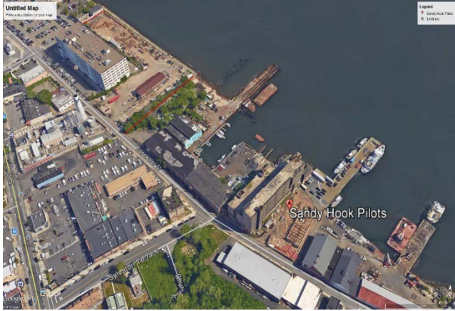
Figure 1: Sandy Hook Pilot Station and Yacht Yard
