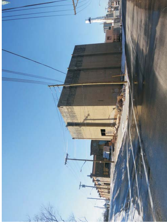
12. View of the northwest corner of Edgewater Street and Sylvaton Terrace.
