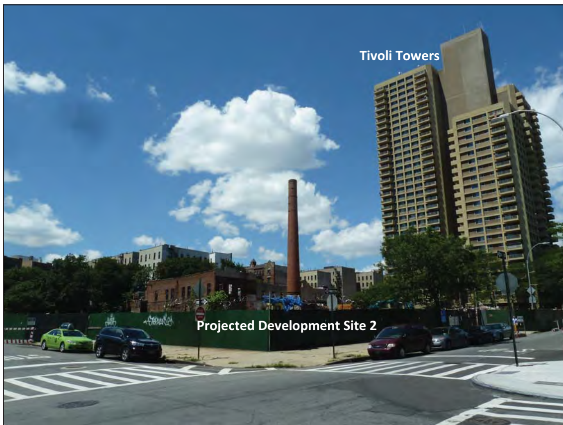
Photo 2: View northwest from the intersection of Franklin Avenue and Montgomery Street.
