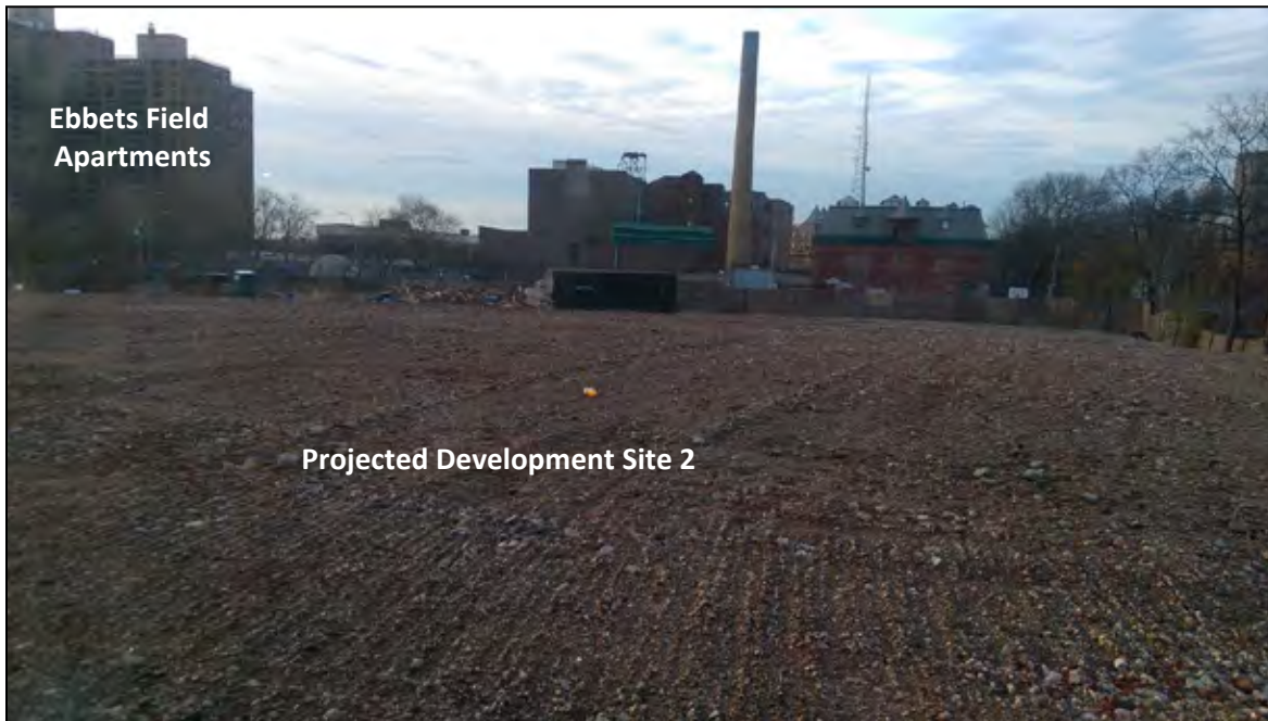
Photo 4: View south across Crown Street with Projected Development Site 2 in the foreground and the Ebbets Field Apartments in the background.
