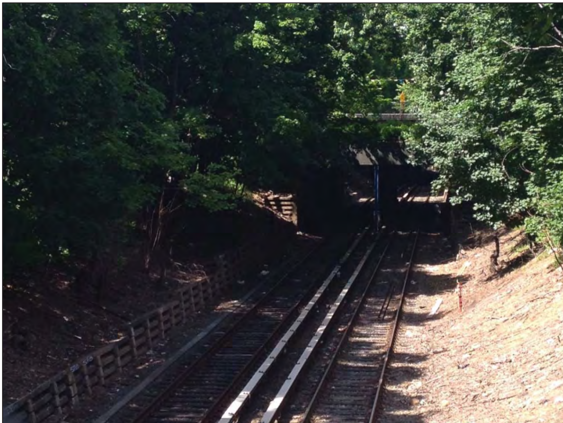
Photo 8: View south of the Franklin Avenue Shuttle tracks from President Street.
