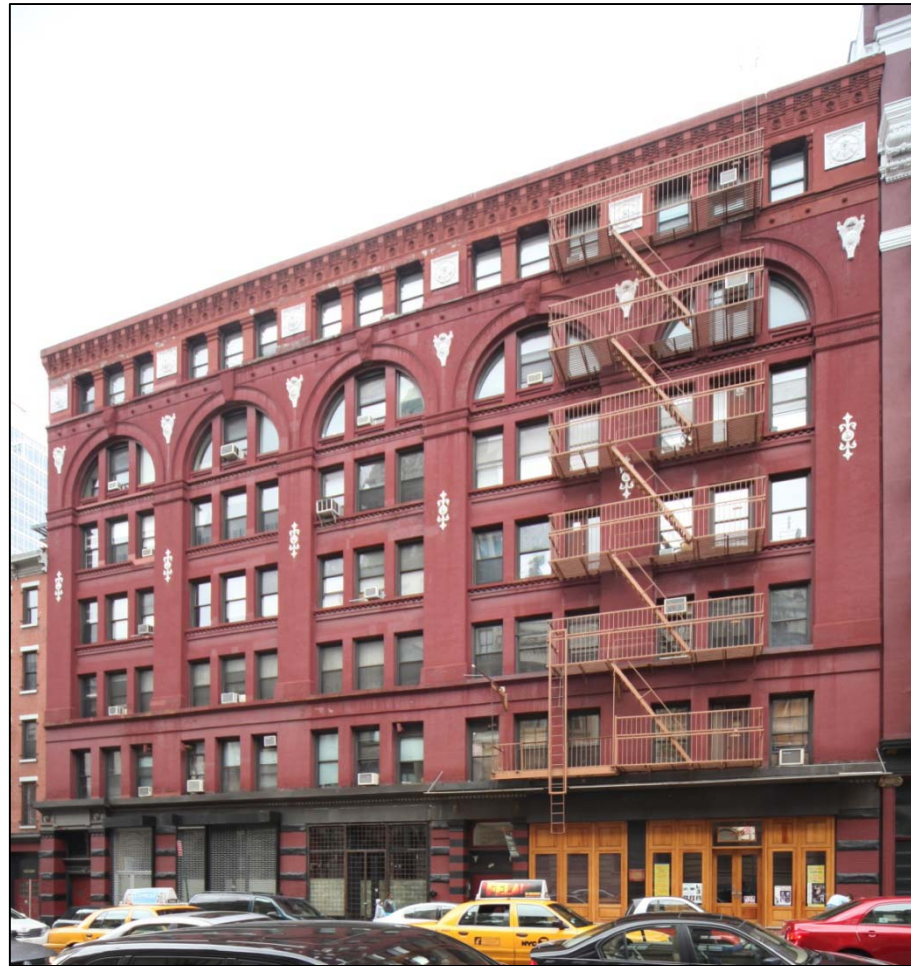
241-249 Centre Street (1888-89, DeLemos & Cordes) Photo by Christopher D. Braze, 2010
