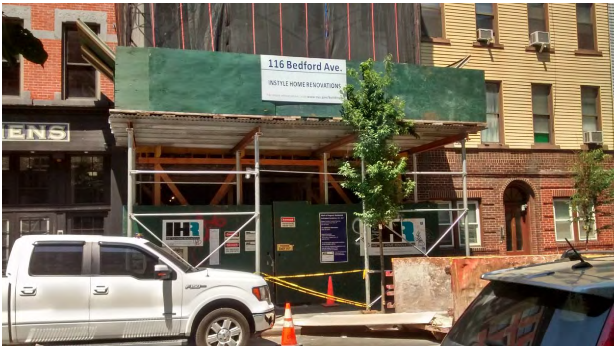
Up close construction and scaffolding at Projected Site 1 (Lot 16)
