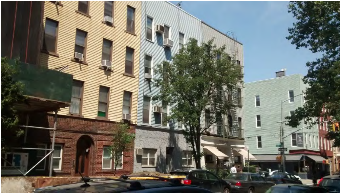
View of Projected Sites 2, 3, and 4 looking north on Bedford Avenue towards N. 11 th Street
