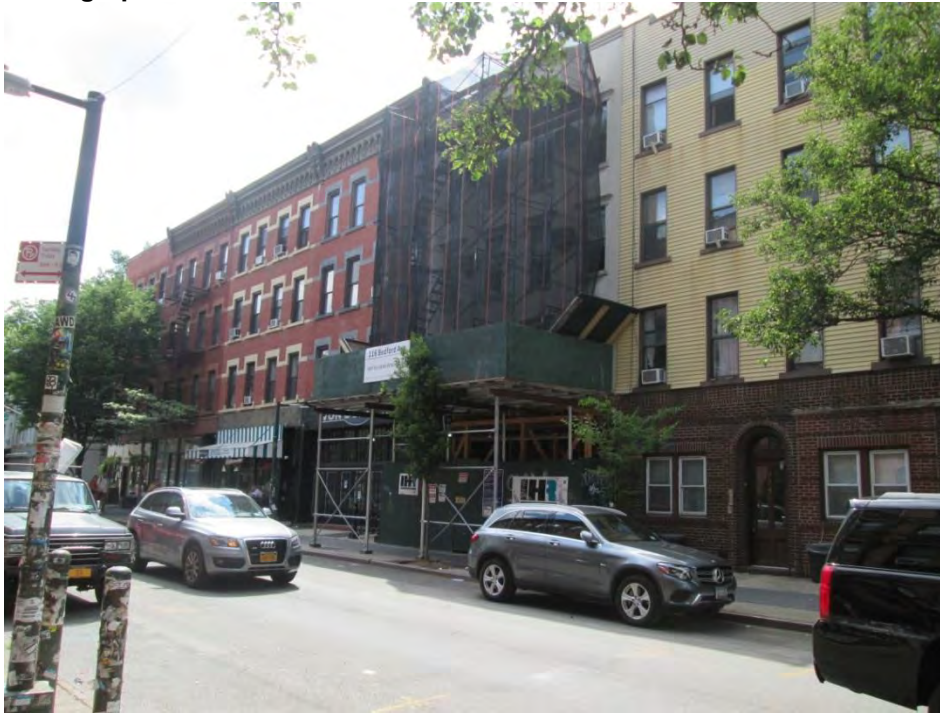
View of the projected development site at 116 Bedford Avenue (Lot 16) looking south
