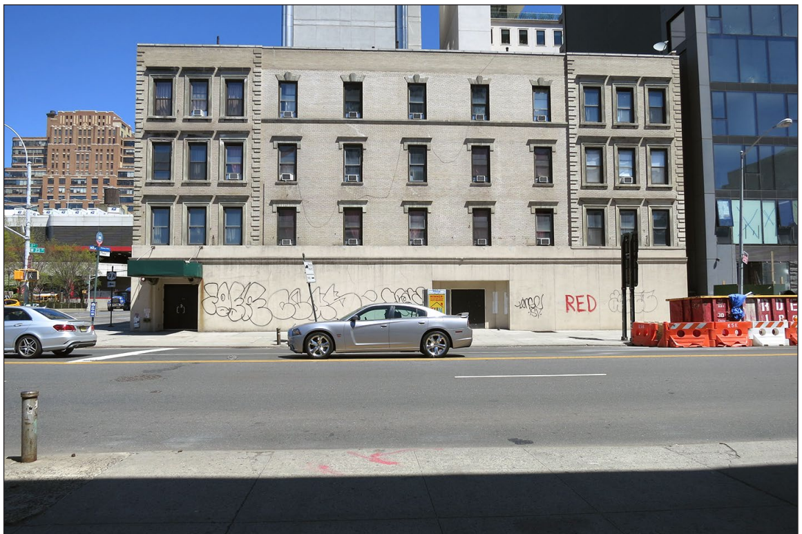
View of the West 23rd Street façade of the former Terminal Hotel 2
