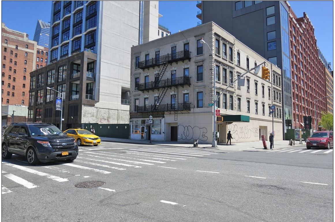
View northeast of the former Terminal Hotel 1
