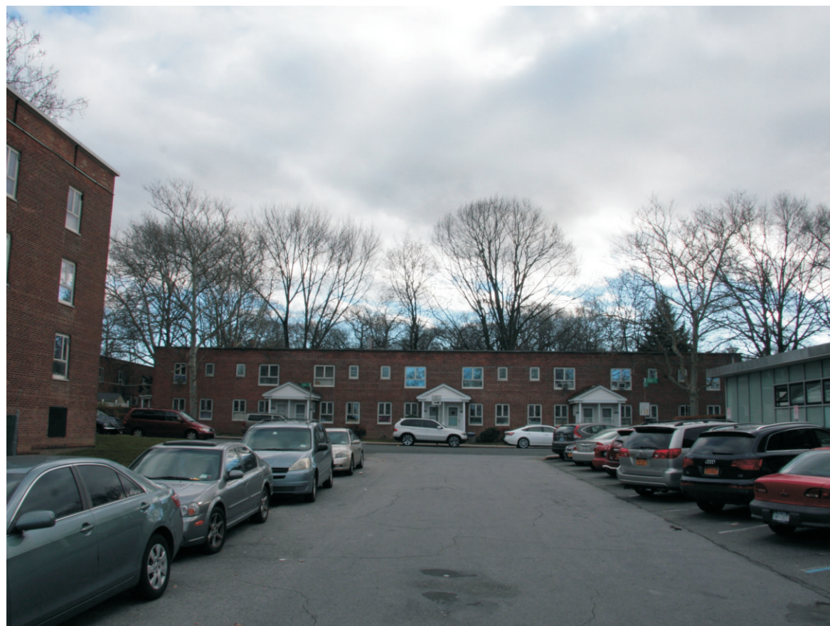
18. View of 194th Street facing south.
