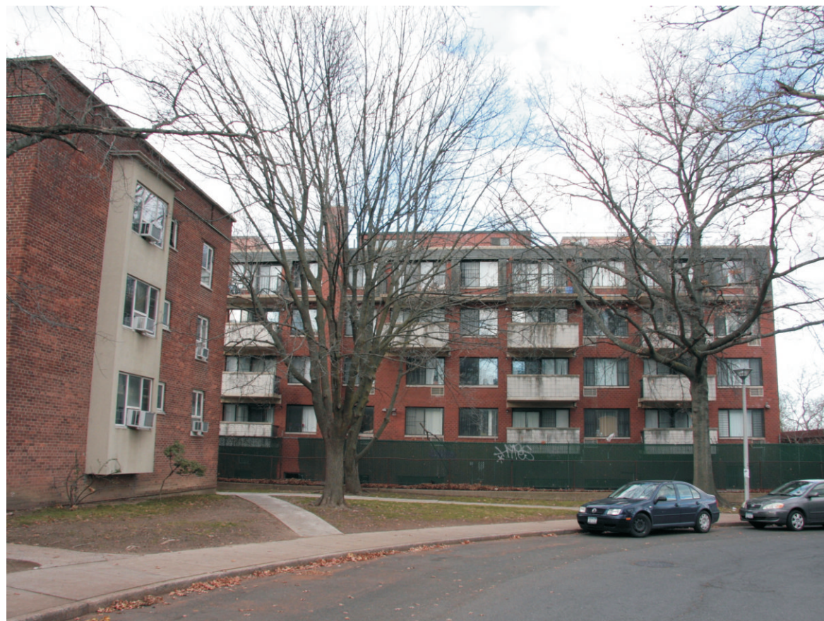
15. View of the Site along 194th Street facing north.
