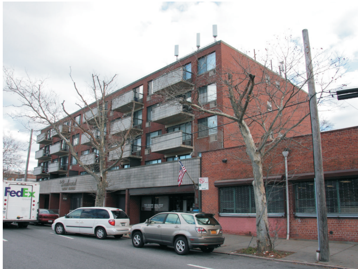
3. View of the eastbound side of Horace Harding Expressway facing southeast.
