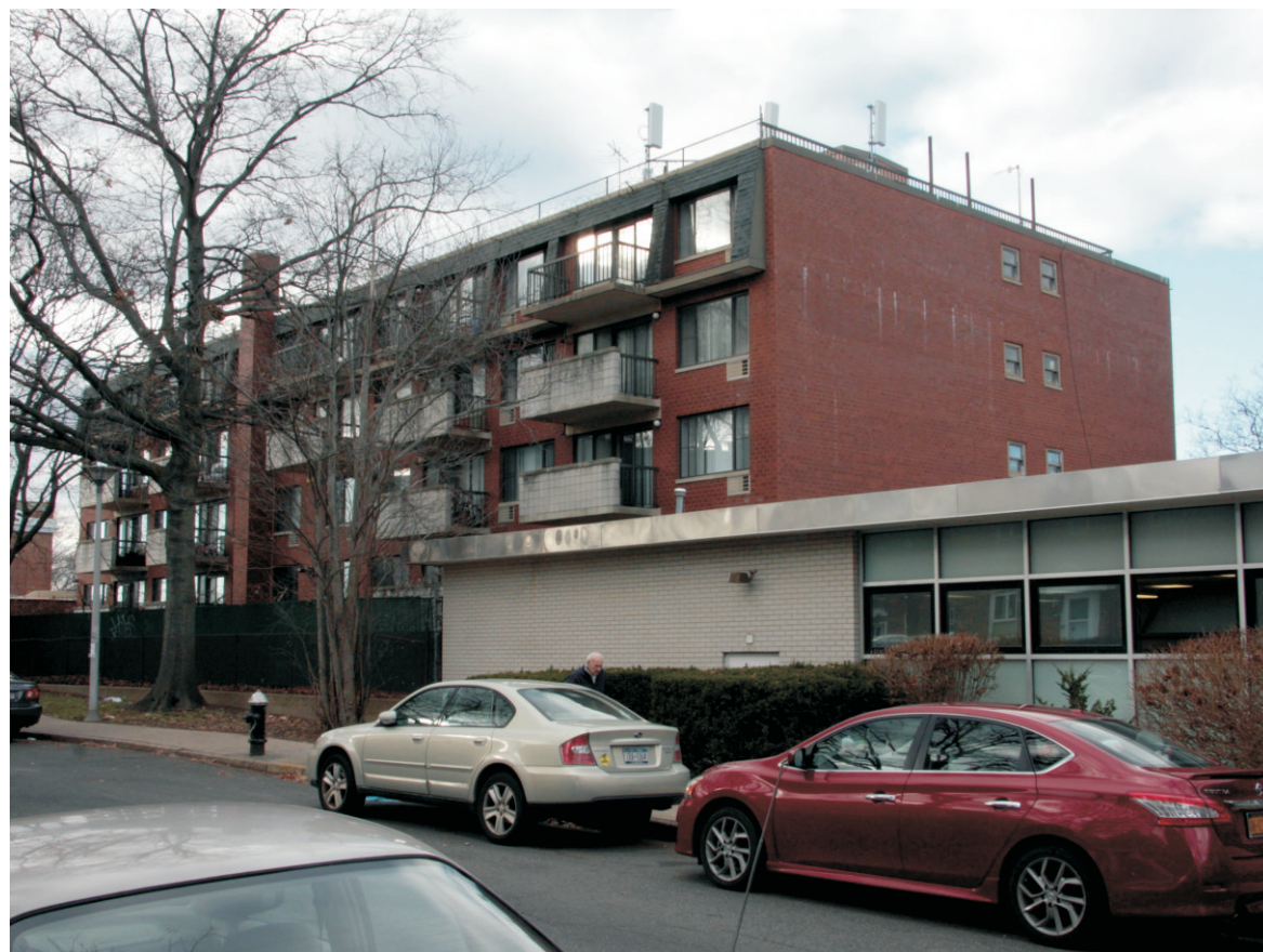
12. View of the north side of 194th Street facing northwest.
