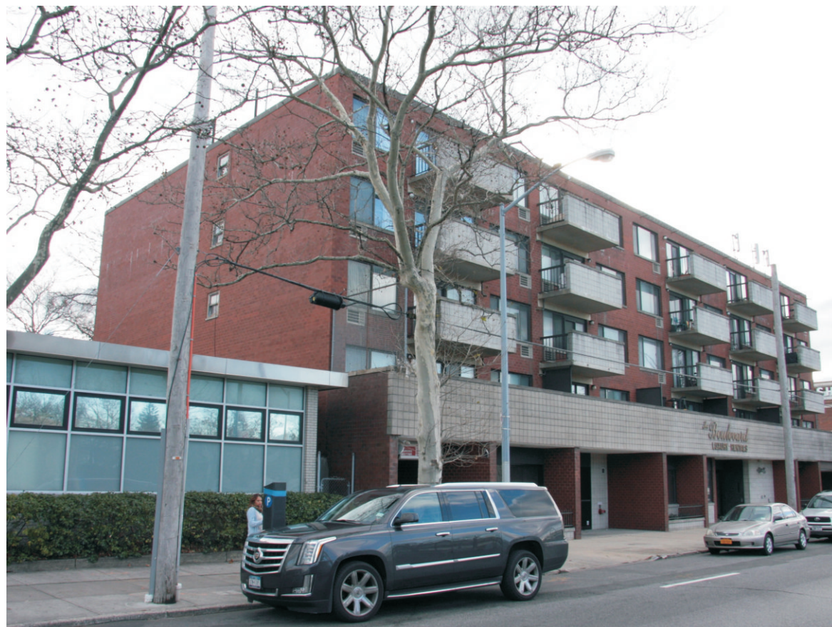
6. View of the eastbound side of Horace Harding Expressway facing southwest.
