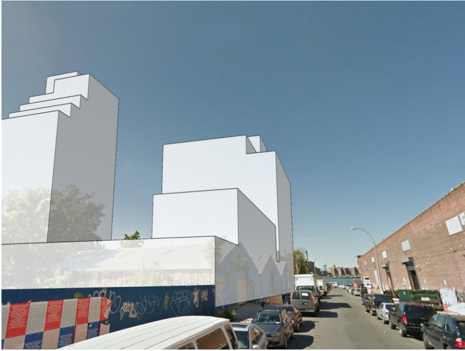
Kent Street facing west (Site at left)
