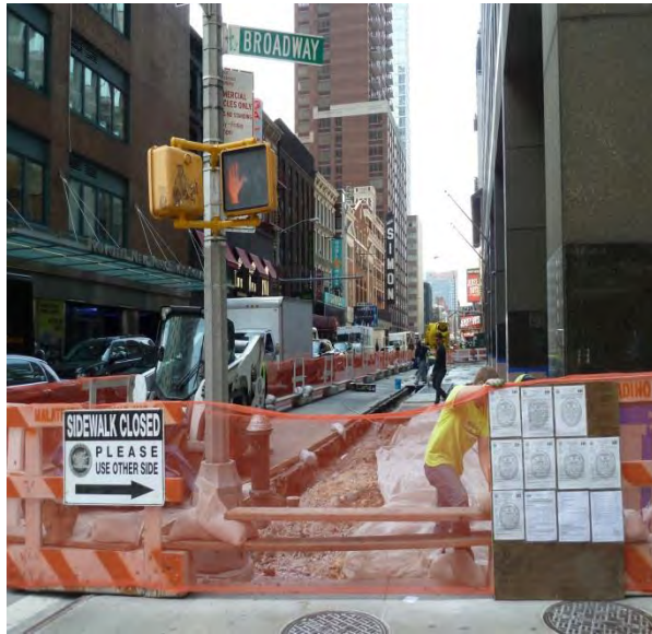
1. Looking towards site and adjacent sites from W. 52nd Street
