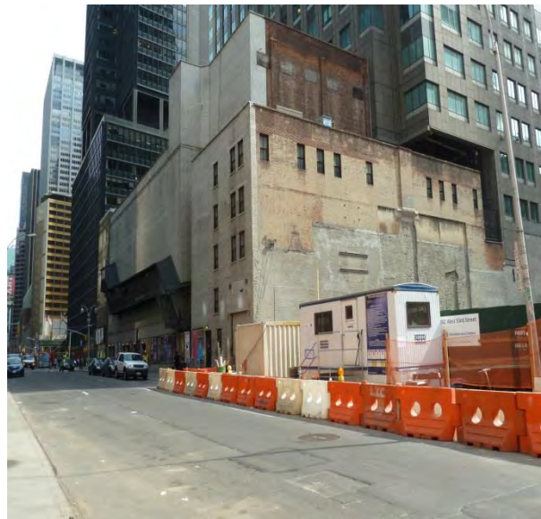
12. Looking towards adjacent sites from W. 53rd Street
