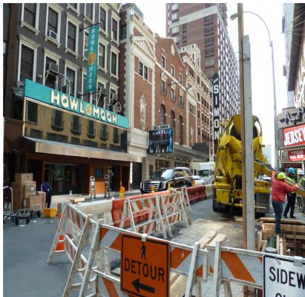
3. Looking away from site from W. 52nd Street
