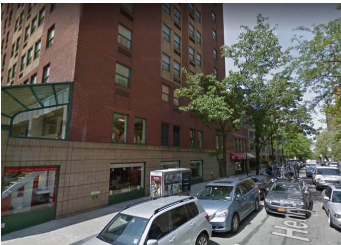
20. View of the Site facing west from West 90th Street.
