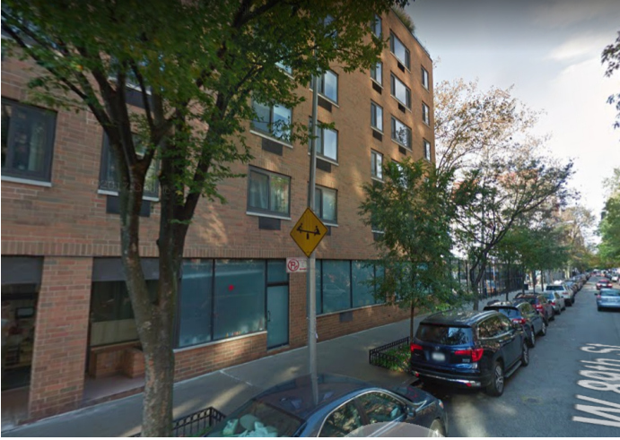
7. View of West 89th Street facing west from the Site.
