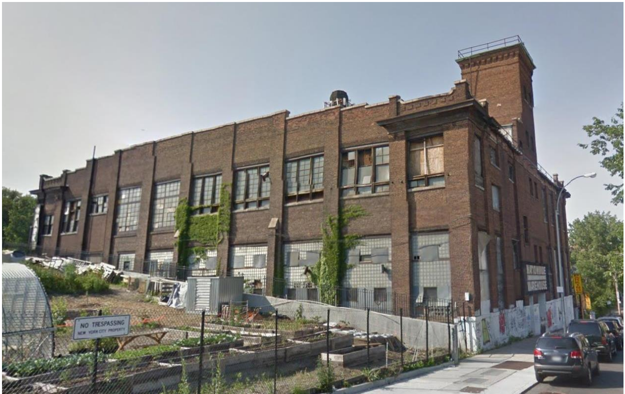
Circa 2015 Google street view looking at the south elevation of the Morgan Steam Laundry building.
