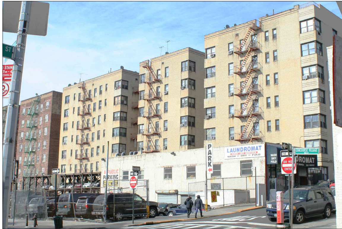
1. View of Site A from Concourse Village West and E. 156th Street.
