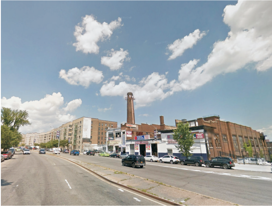
Grand Concourse facing northeast (Site at right)
