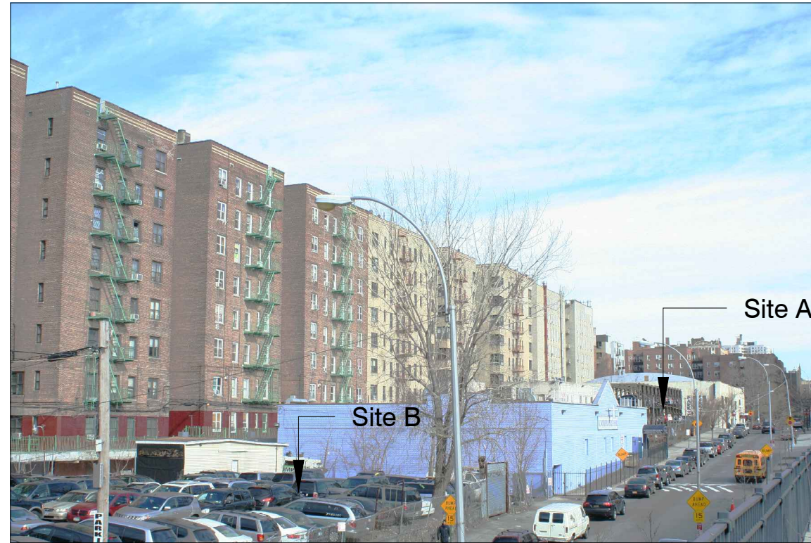
2. View of Site B and Site A beyond along Concourse Village West.
