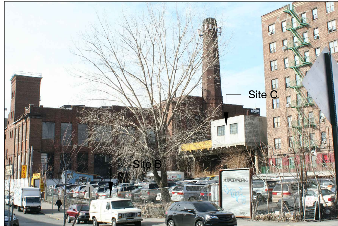
4. View of Site B and rear of Site C.
