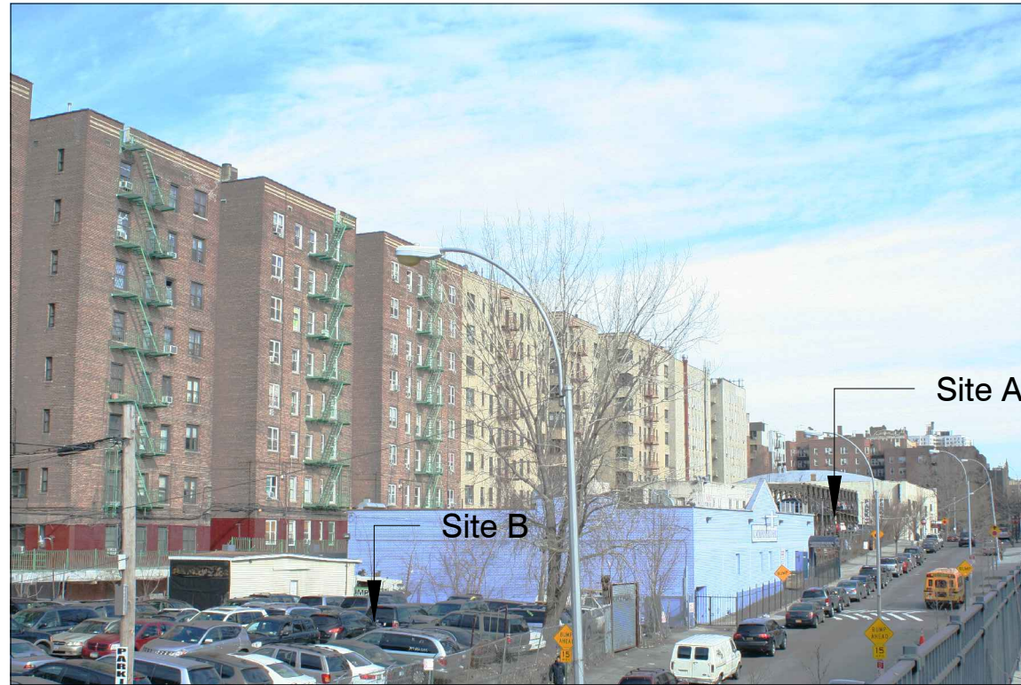
2. View of Site B and Site A beyond along Concourse Village West.
