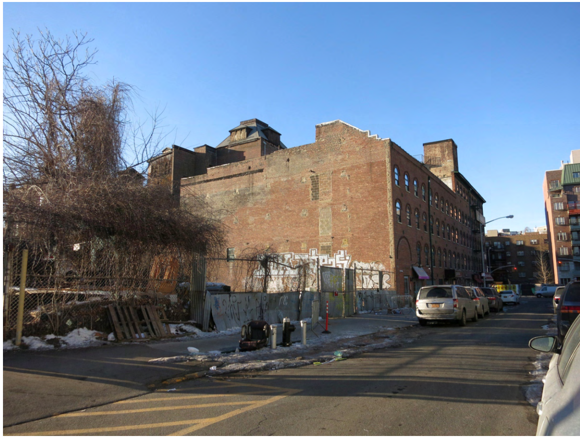
4. View of Site 2 facing northwest from Skillman Street.
