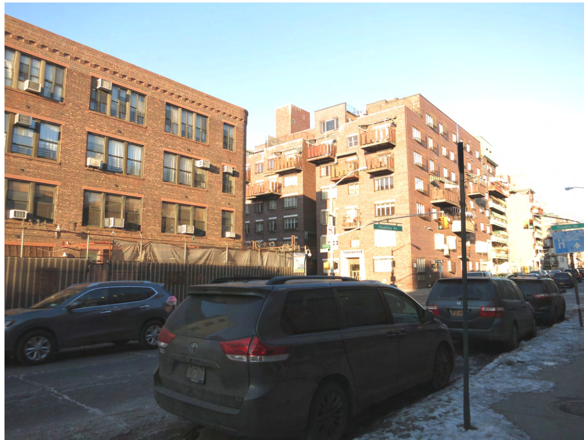
27. View of the side of Flushing Avenue facing northeast from Site 1.
