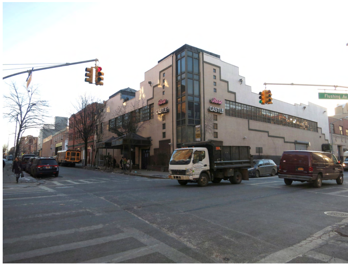
25. View of Site 1 facing southwest from the intersection of Franklin Avenue and Flushing Avenue.
