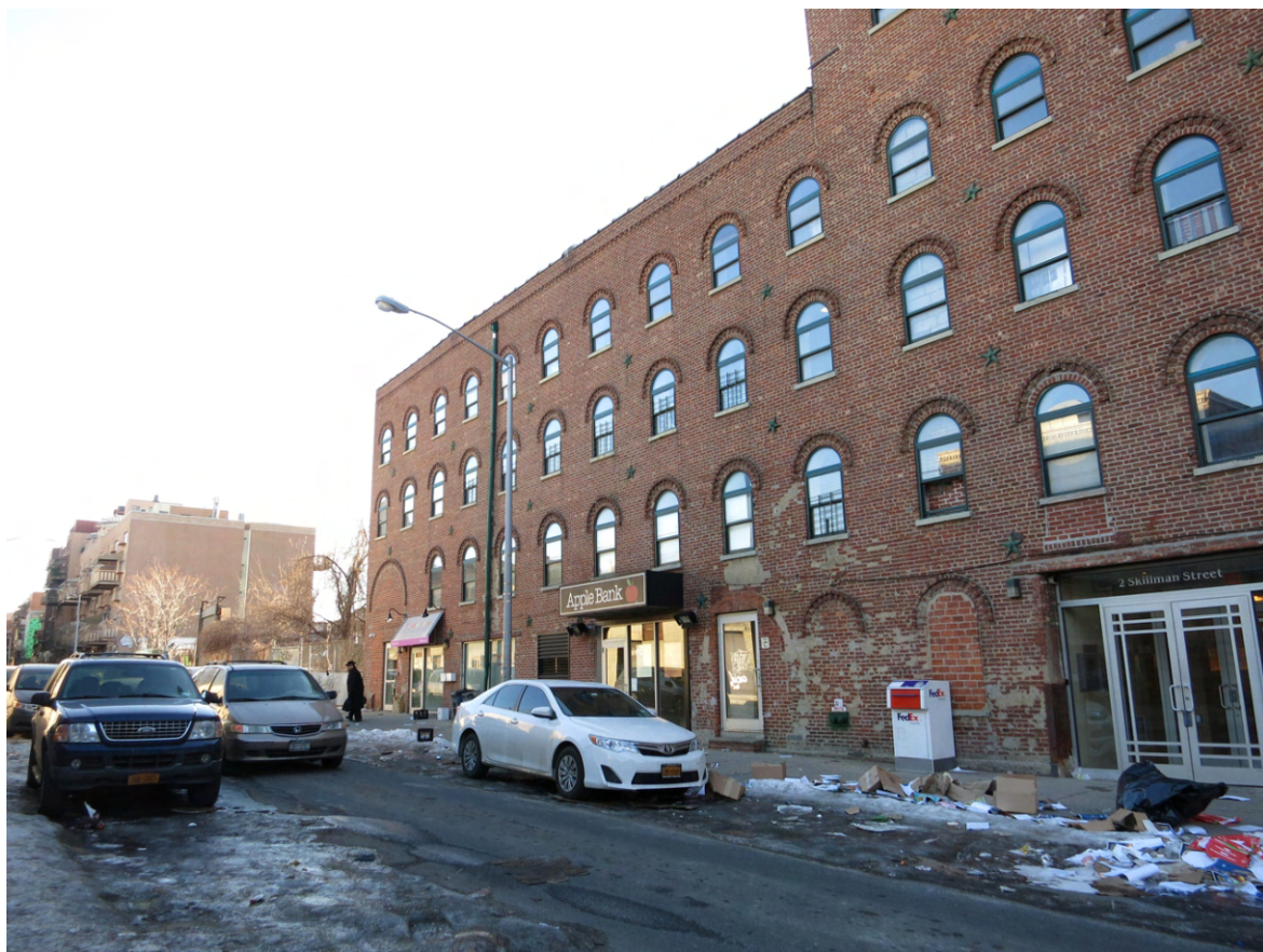
6. View of the west side of Skillman Street facing southwest.
