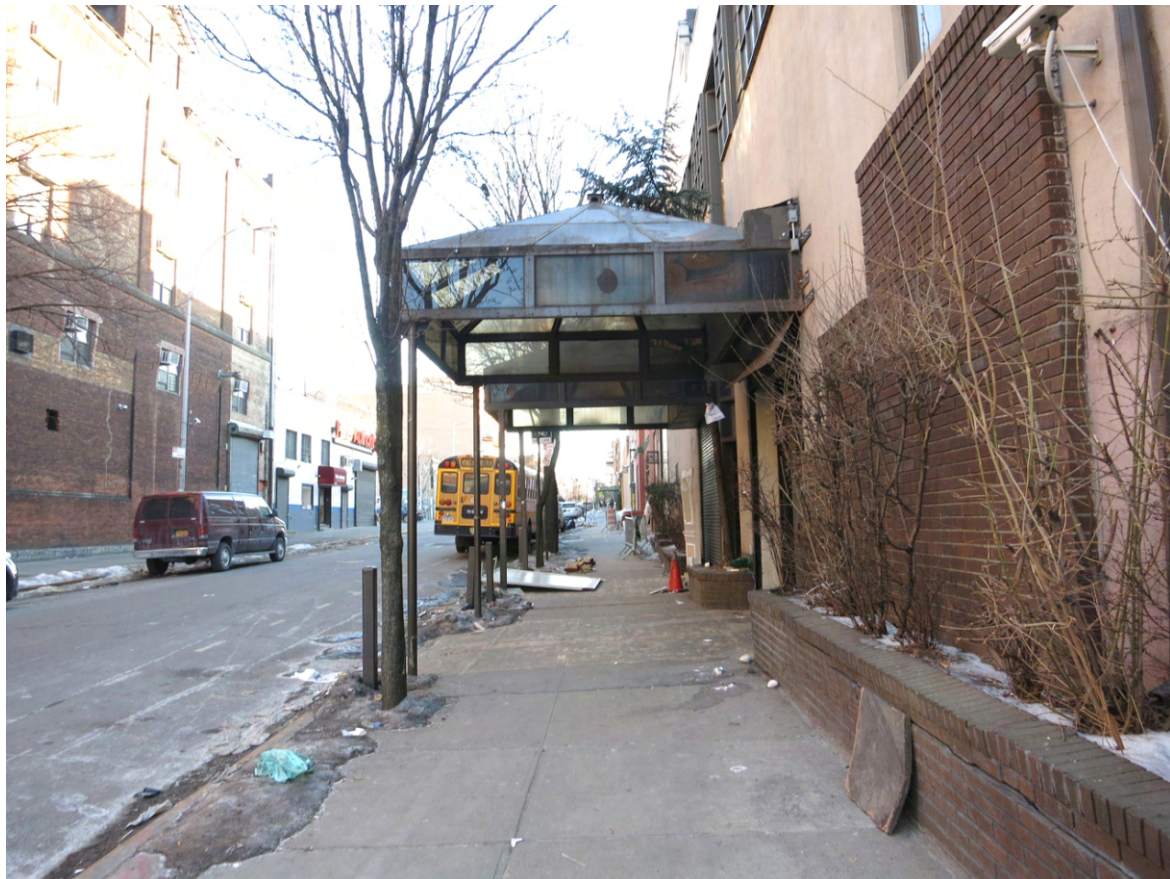
21. View of the sidewalk along the west side of Franklin Avenue facing south from Flushing Avenue.
