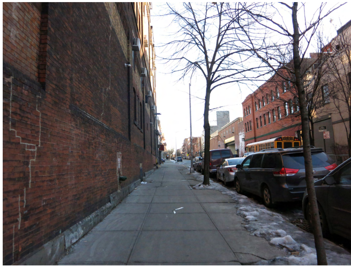
13. View of the sidewalk along the east side of Franklin Avenue facing south from Flushing Avenue.
