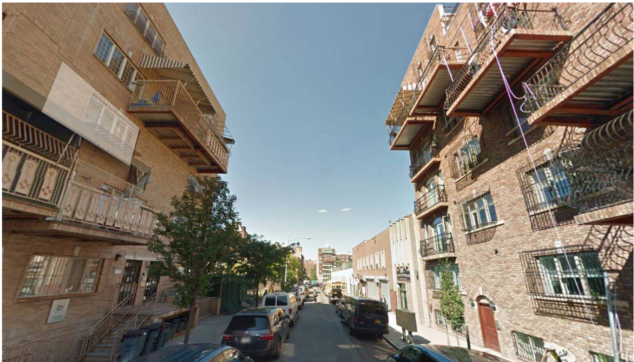
Urban Design 4b: Development Site 2, view north on Skillman Street – No Action
